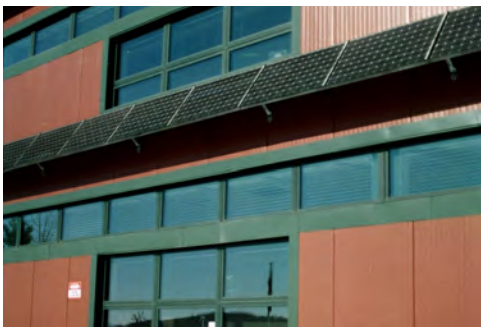
a (top) not built at the AJLC, b (middle) part of the roof structure at St. Gabriel's, and c (bottom) supporting PV panels at Wind NRG.
