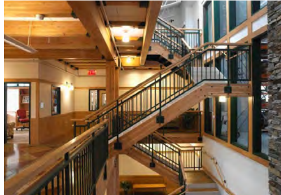
Figure 4.2.34 Looking west through the interior commons
