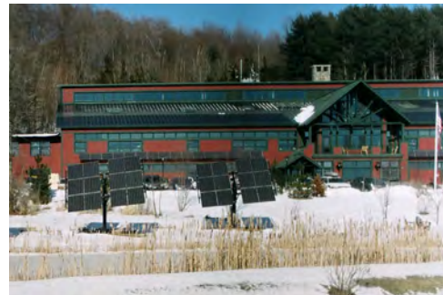
Figure 4.6.10 Synergy: landscapes are enjoyable and may assist with climate control inside the building
