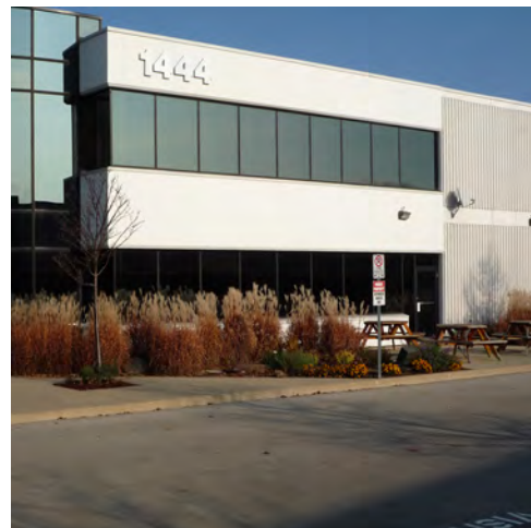
Figure 5.1.11 Various combinations of WWR and solid enclosure material
