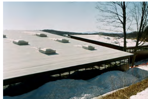
Figure 4.5.9 Alternatives used to realize a thermally resistive roof: a (middle) "green roof" at Plaza at PPL (image Peter Aaron/Esto) b (bottom) white TPO membrane at Wind NRG.
