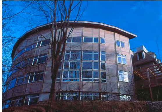
Figure 4.2.54 North facade, from the ravine
