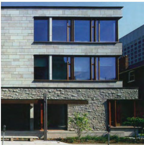
Figure 2.4.7 b Contrasting surface textures at McKinsey & Company Headquarters
