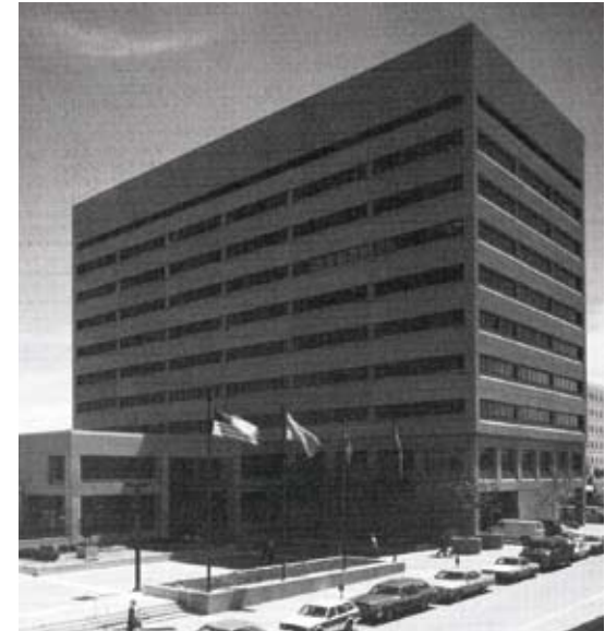
Fig. 2.5 Wilmington Delaware City Hall
