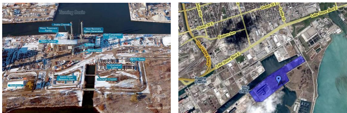
Figure 3.8: The construction site layout (Photo source: The project website and Google map) The general methodology and plan of the field experiments are discussed in the following sections.
