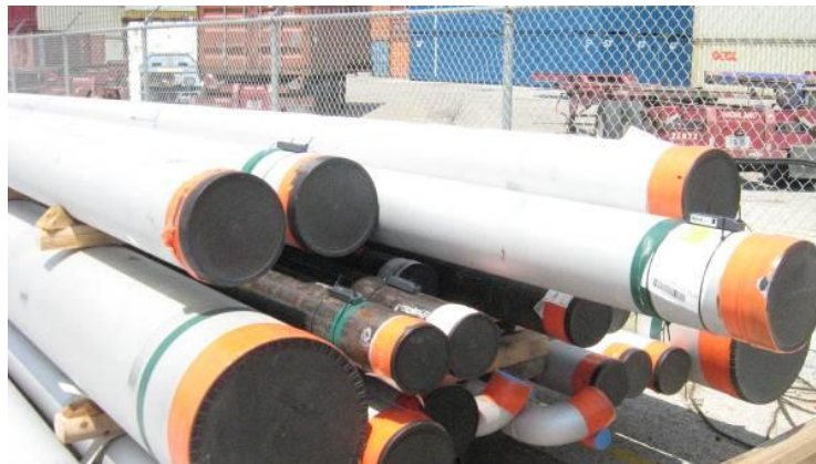
Figure 3.9: Tagged pipe spools at the receiving point
