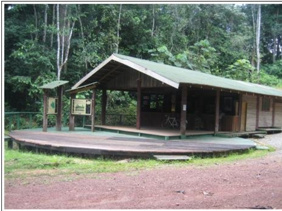
Figure 42. Visitors' Centre and Restaurant.
