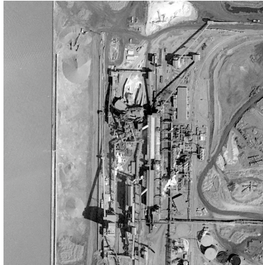
Blast Furnace E, Stelco
