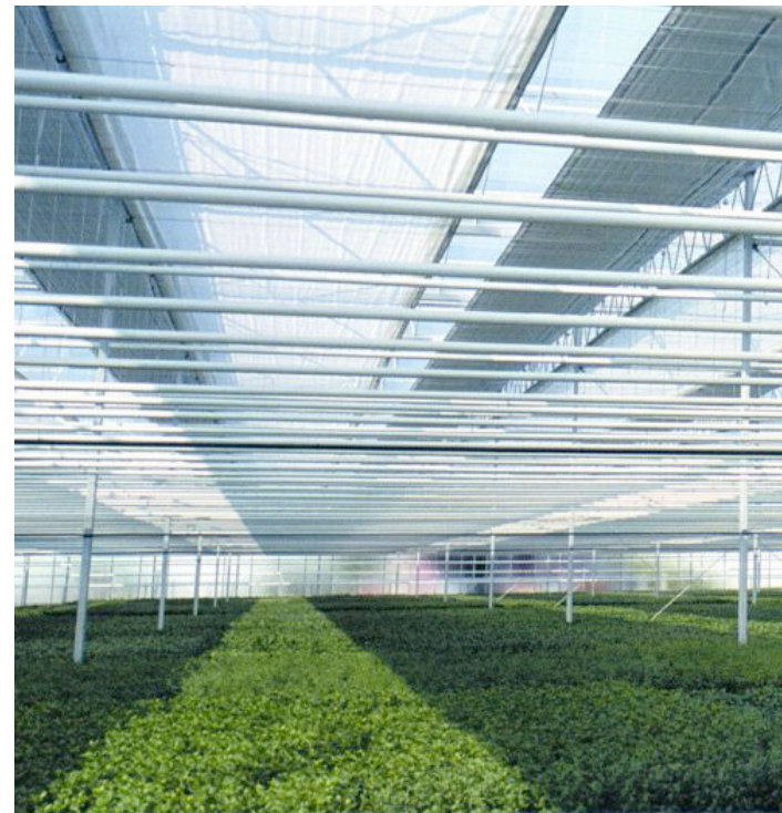
Fig.2.40 A commercial scale greenhouse facility
