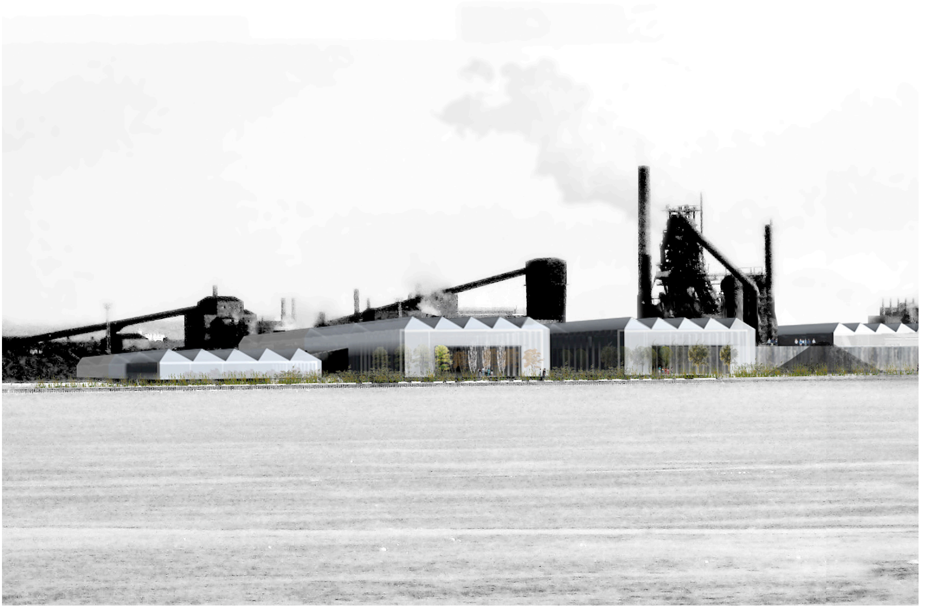
Fig.2.59 A panoramic view of the site from across Hamilton Harbour
