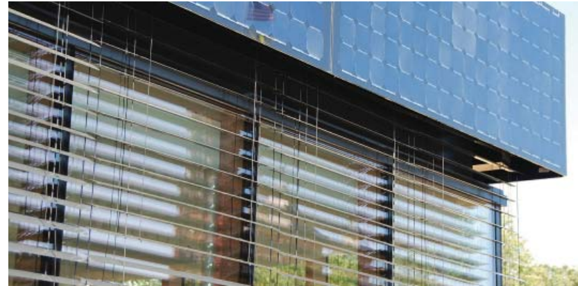
Figure 2.19: Detail of Building Integrated Photovoltaic Panel at south fascia, and deployed exterior shades.
