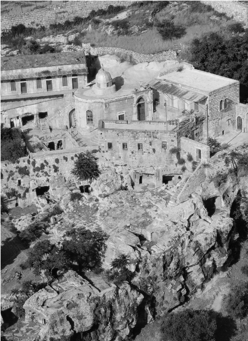
fig.2.15. Saint Onuphrius, built into the existing rock and caves embedded boundaries
