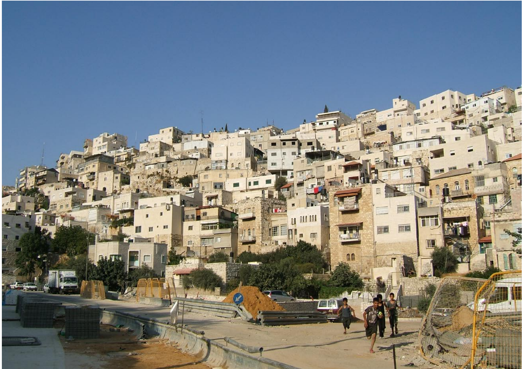
fig.1.21. road work in Silwan, 2009
