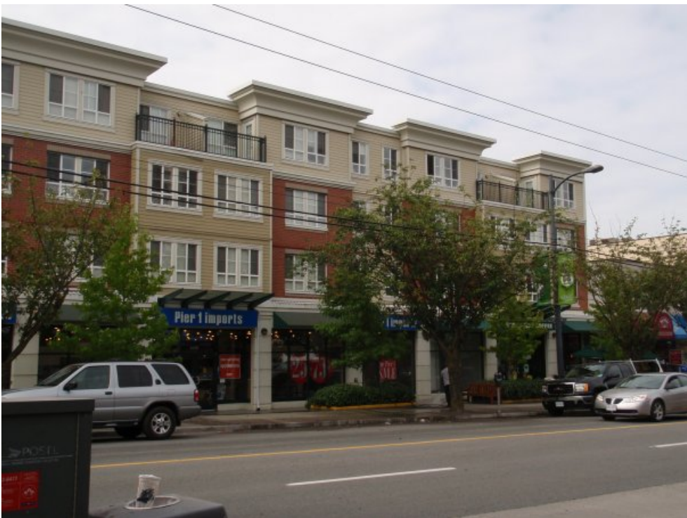
Figure 3.4. W 41 st Ave View 3.
