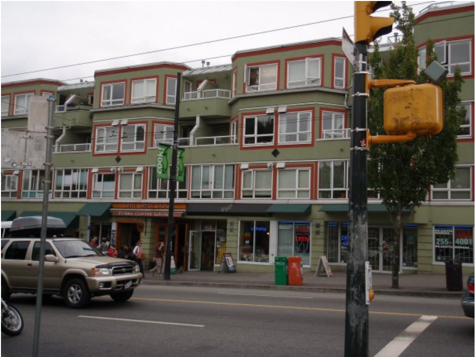
Figure 3.7. Commercial Drive View 2.
