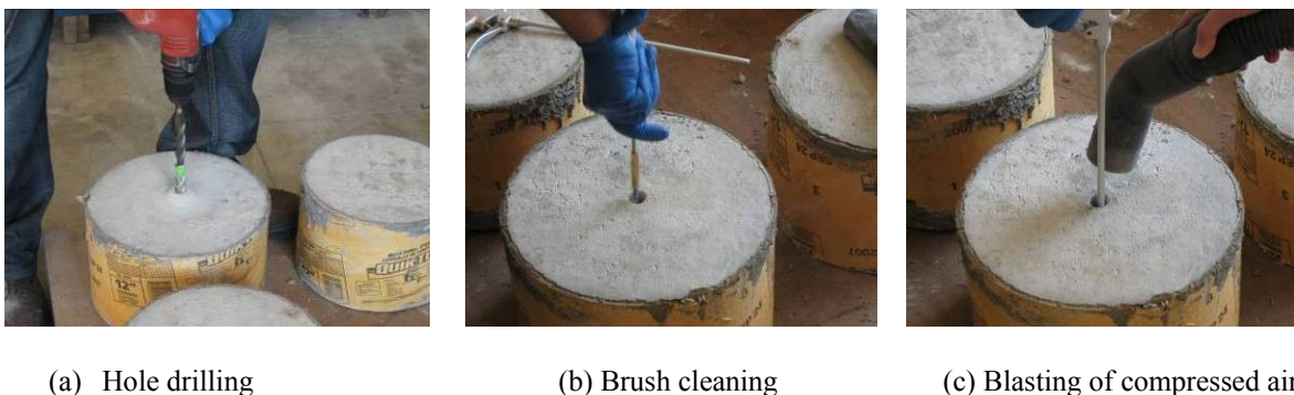
Figure 3.2 – Drilled hole preparation prior to anchor installation
