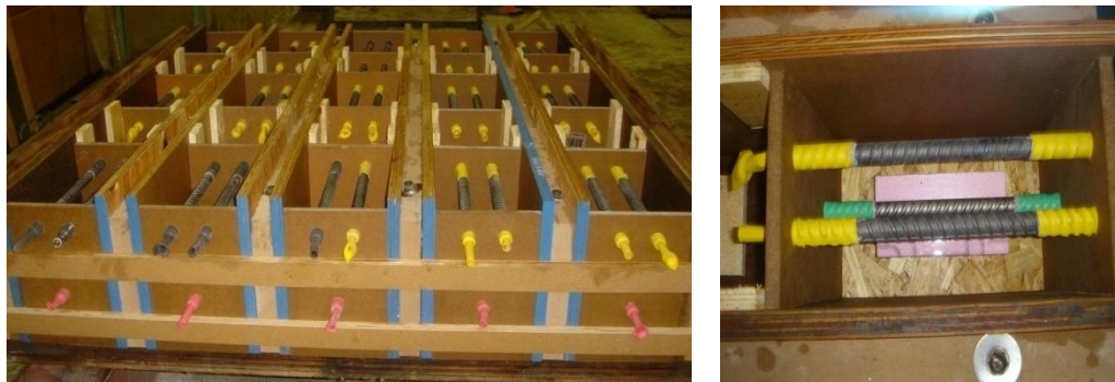
Figure 19: Form work for the casting of the ASTM A 955M prisms
