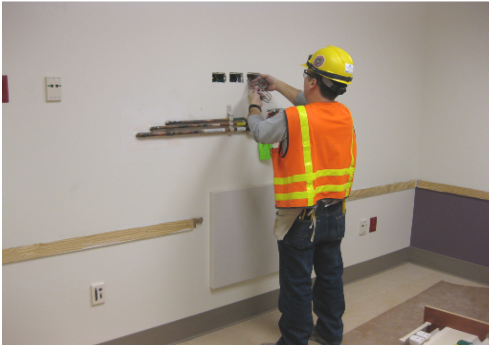
Figure 9: Example of direct-work - electrician installing outlet
