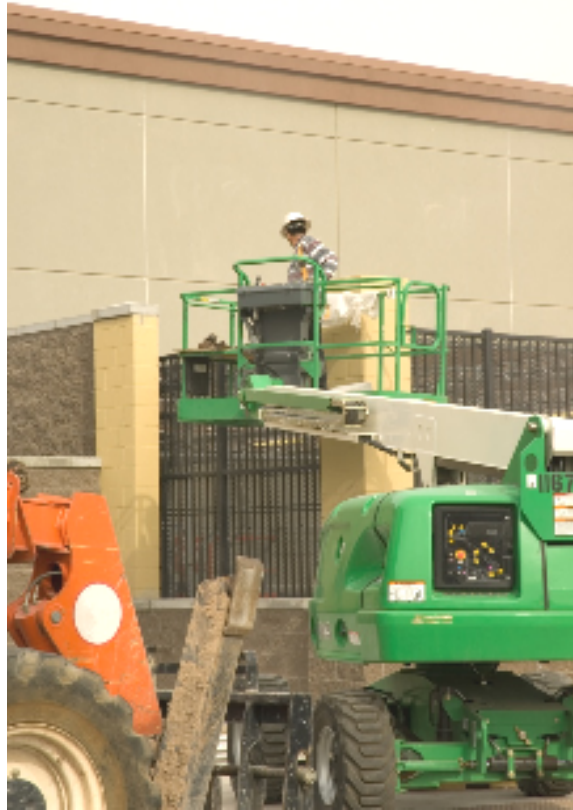
Figure 12: Example of tools-and-equipment - adjusting boom lift
