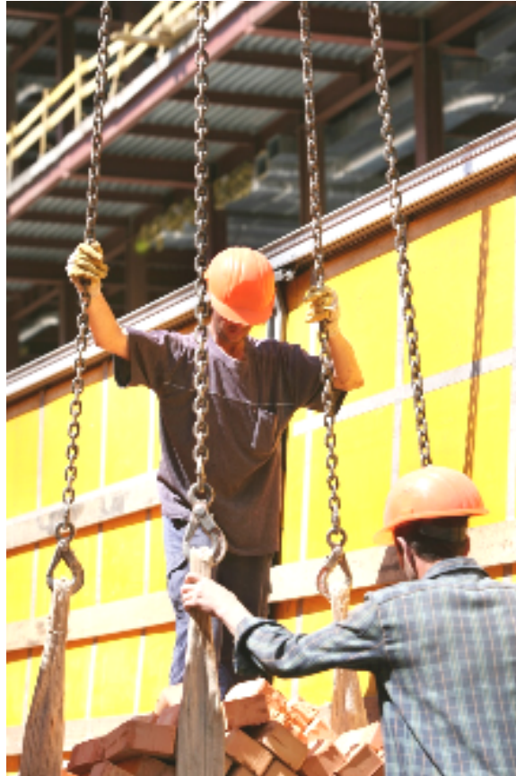
Figure 13: Example of material-handling - moving bricks
