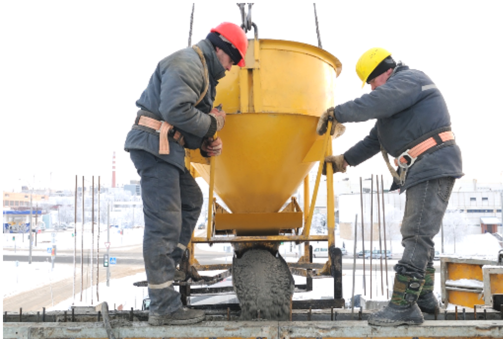
Figure 7: Example of direct-work - placing concrete
