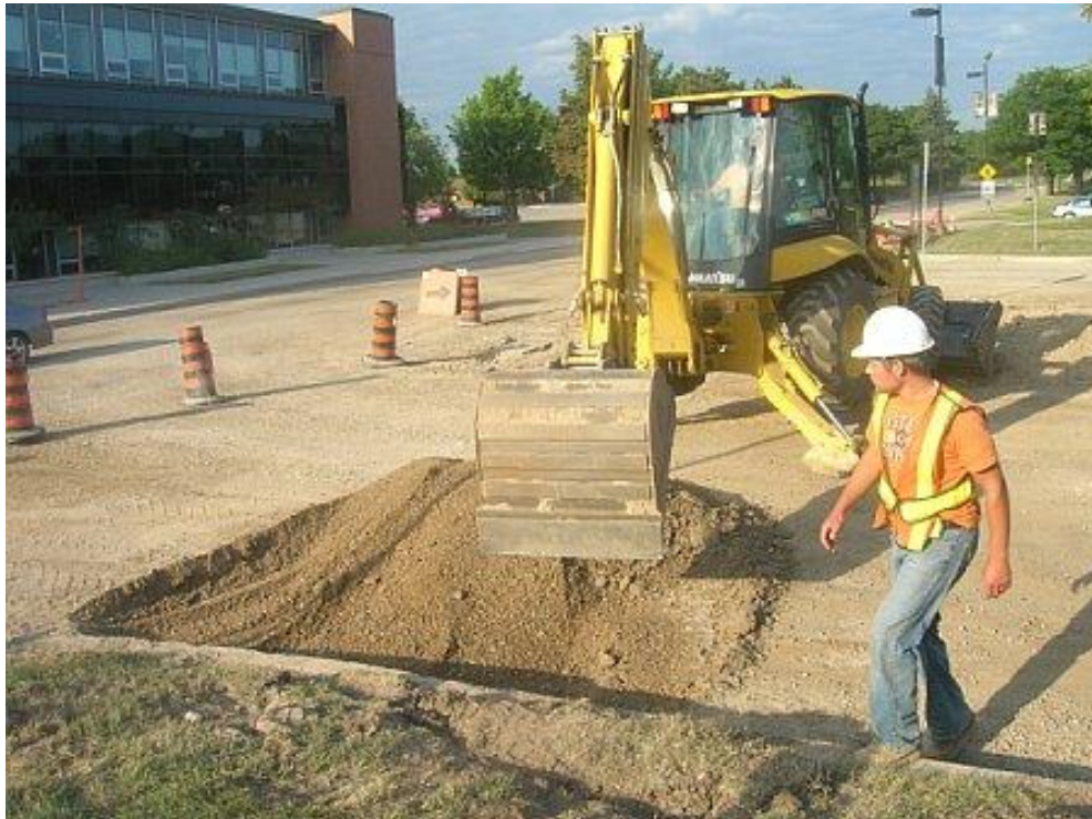
Figure 56 Excavation of Subbase
