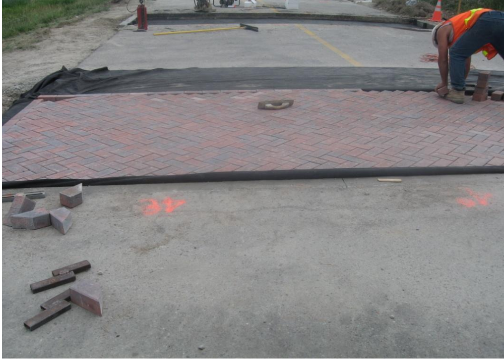
Figure 18 Laying Interlocking Concrete Pavers
