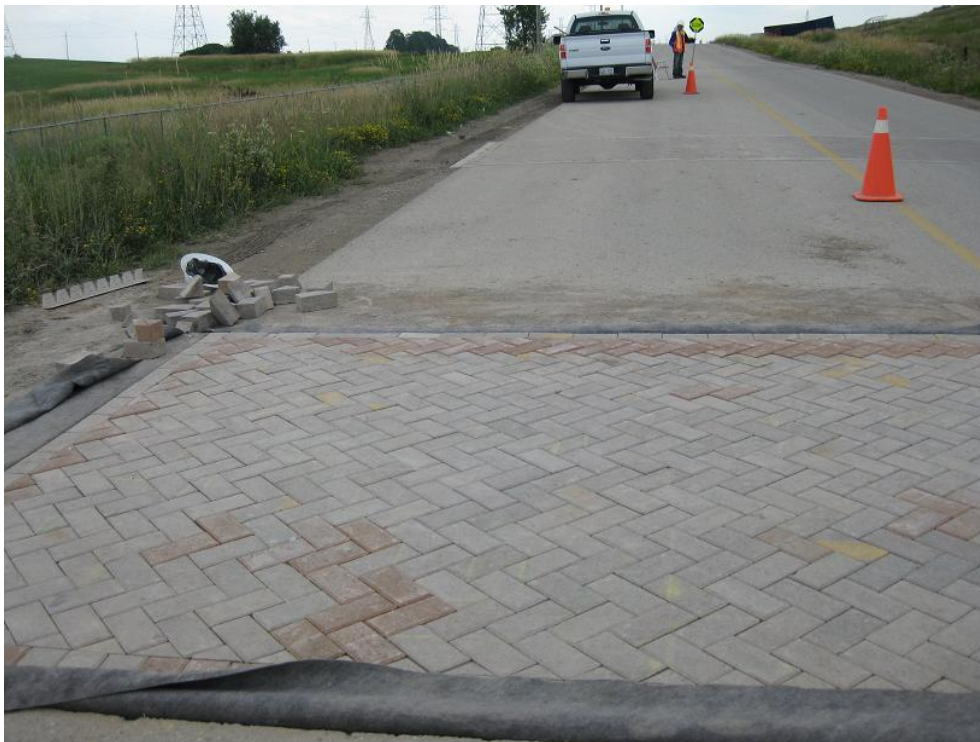
Figure 77 Traffic Control Operations
