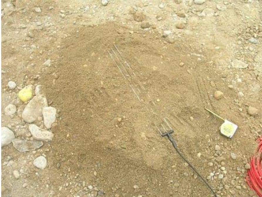
Figure 65: Installation of Moisture Probes
