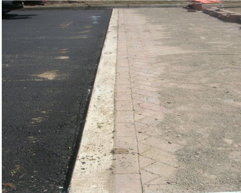
Figure 64 Concrete Header and Joint Sand
