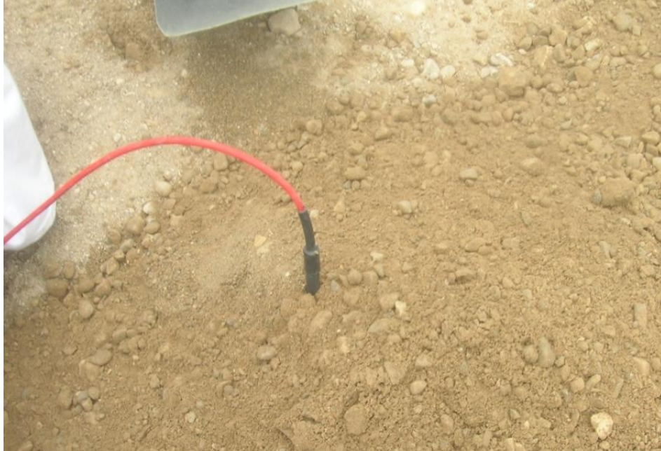
Figure 66 Temperature Probe Installation
