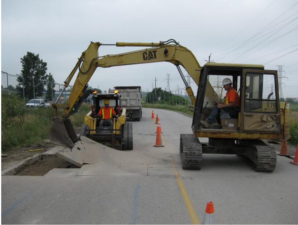
Figure 20 Excavation of Asphalt Pavement
