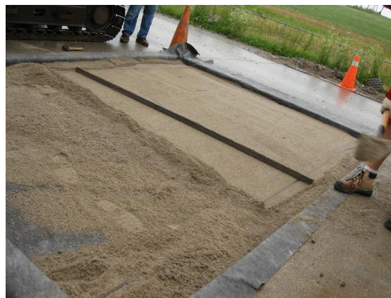
Figure 24 Spreading and Screeding of Bedding Sand
