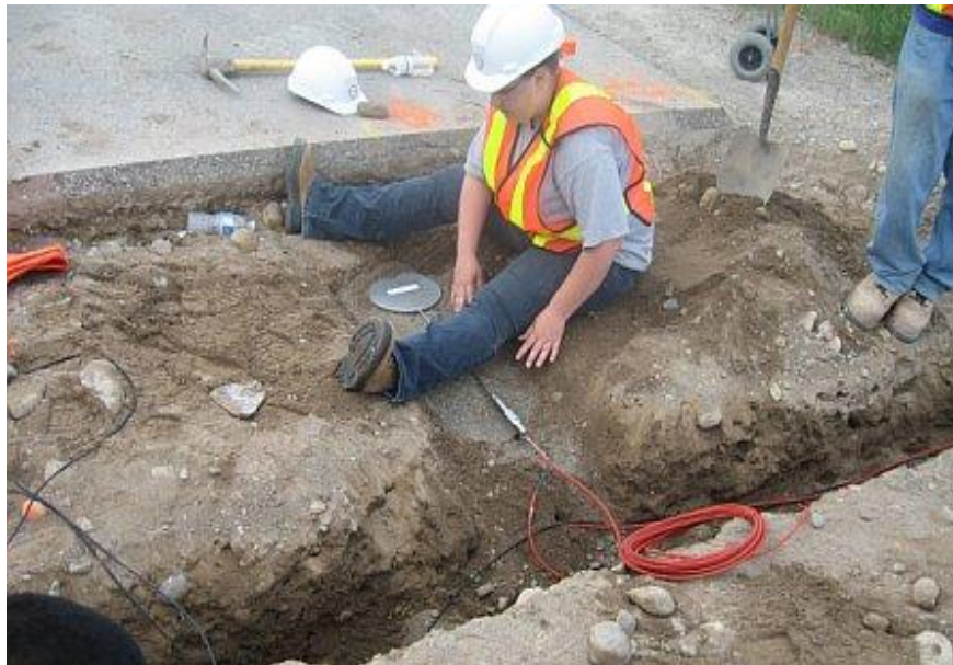
Figure 31 Earth Pressure Cells Installation
