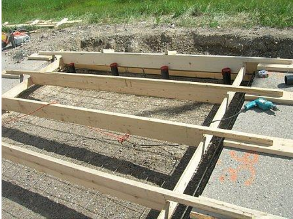
Figure 11 Formworks, Drain Pipes and Reinforcement Bars for Concrete Base Section
