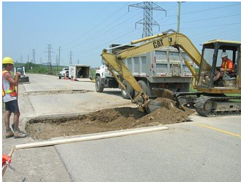
Figure 9 Excavation of Asphalt Pavement
