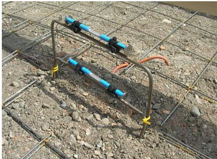
Figure 38 Vibrating Wire Concrete Strain Gauges Installation
