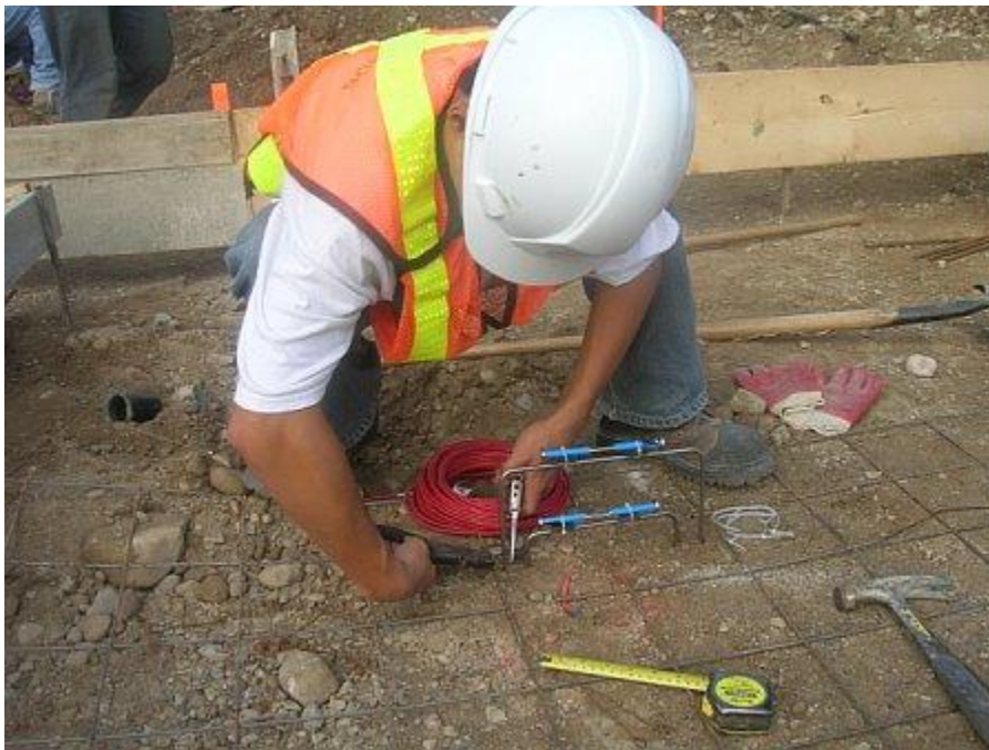
Figure 68 Vibrating Wire Concrete Strain Gauges Installation
