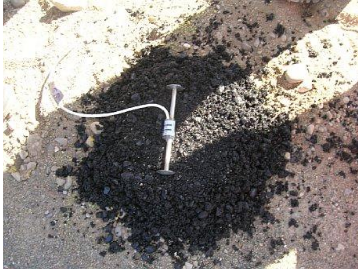
Figure 37 Asphalt Strain Gauge Installation
