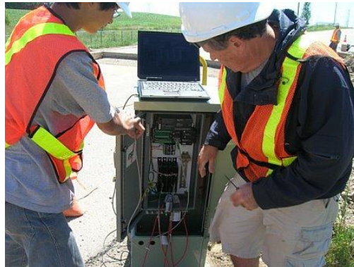
Figure 47 A Preliminary Check of the Sensors after Installation
