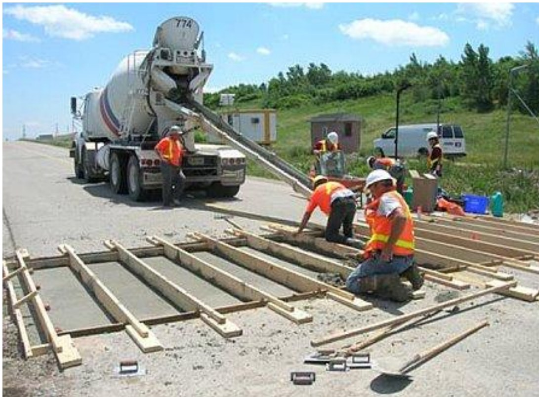
Figure 10 Concrete Base Construction
