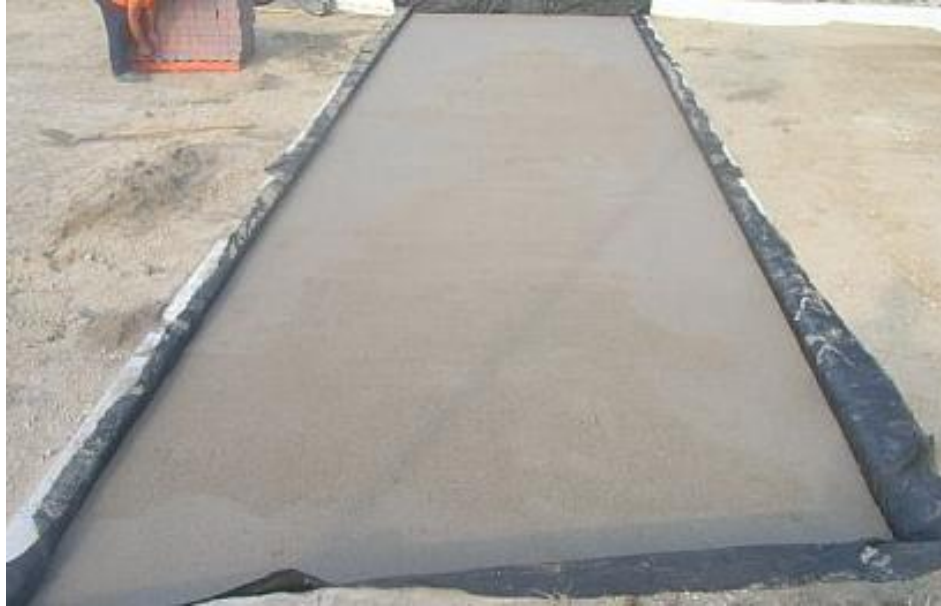
Figure 15 Bedding Sand and Non-woven Geotextile
