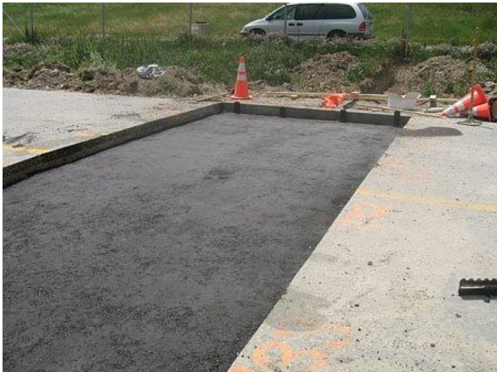
Figure 14 Asphalt Base Section
