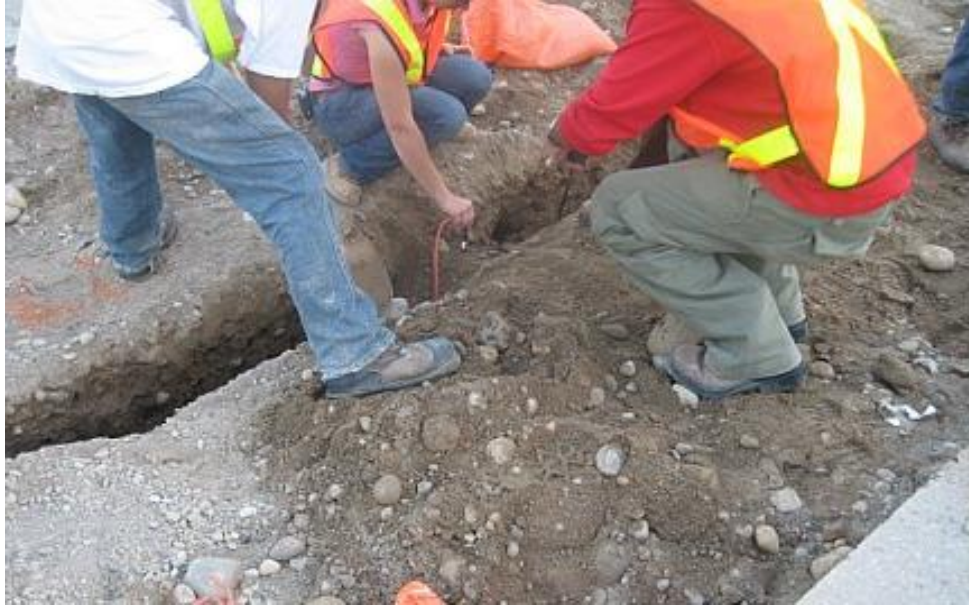
Figure 32 Temperature Probe Installation in First Phase
