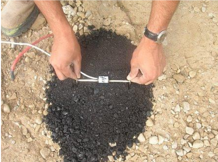
Figure 67 Asphalt Strain Gauge Installation
