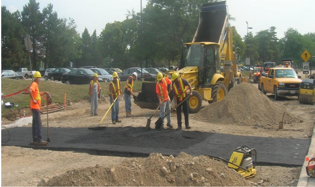
Figure 60 Asphalt Base Construction
