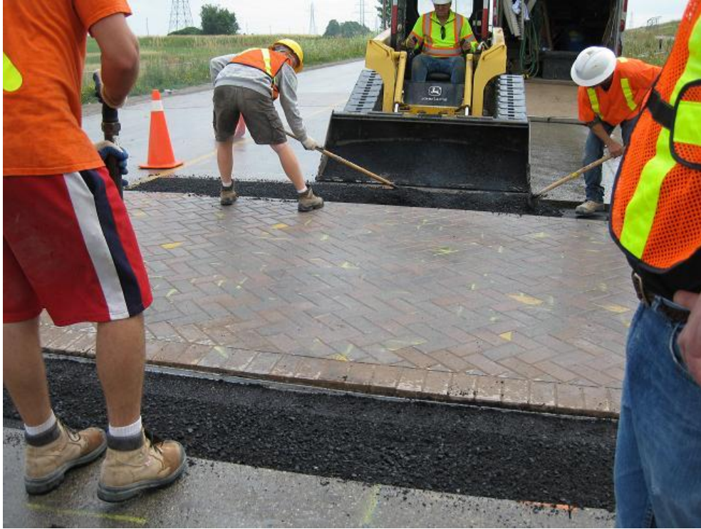
Figure 80 Replacement of Hot Mix Asphalt
