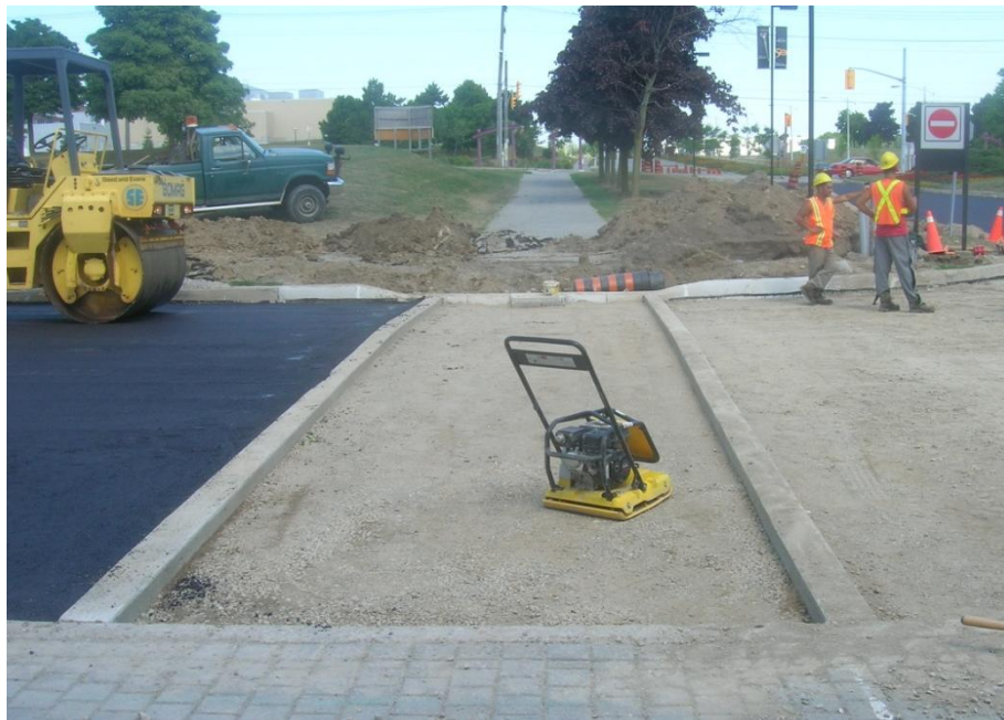
Figure 61 Aggregate Base Construction
