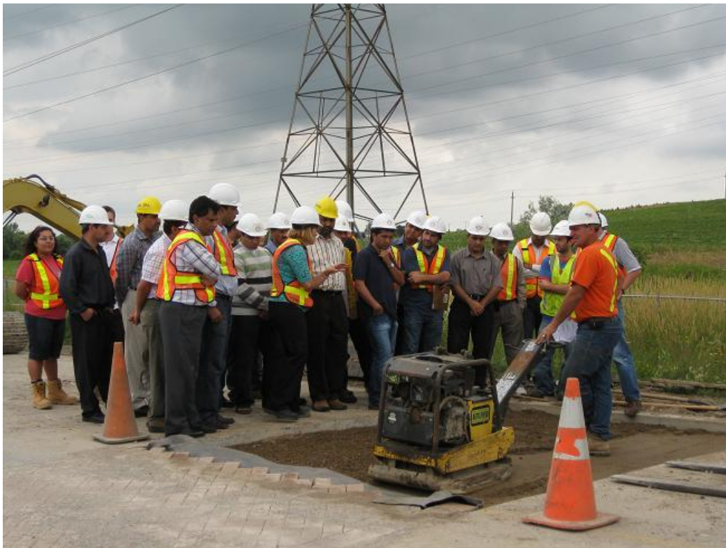
Figure 22 Vibratory Plate Compactor in Crosswalk Base
