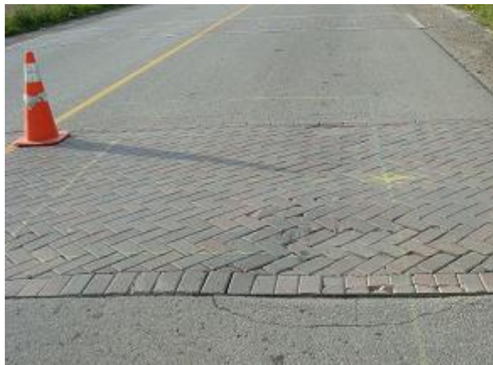
Figure 78 Crosswalk Before Lifting the Pavers
