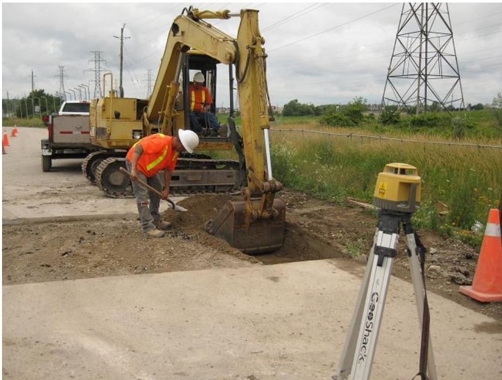
Figure 21 Excavation of Granular A
