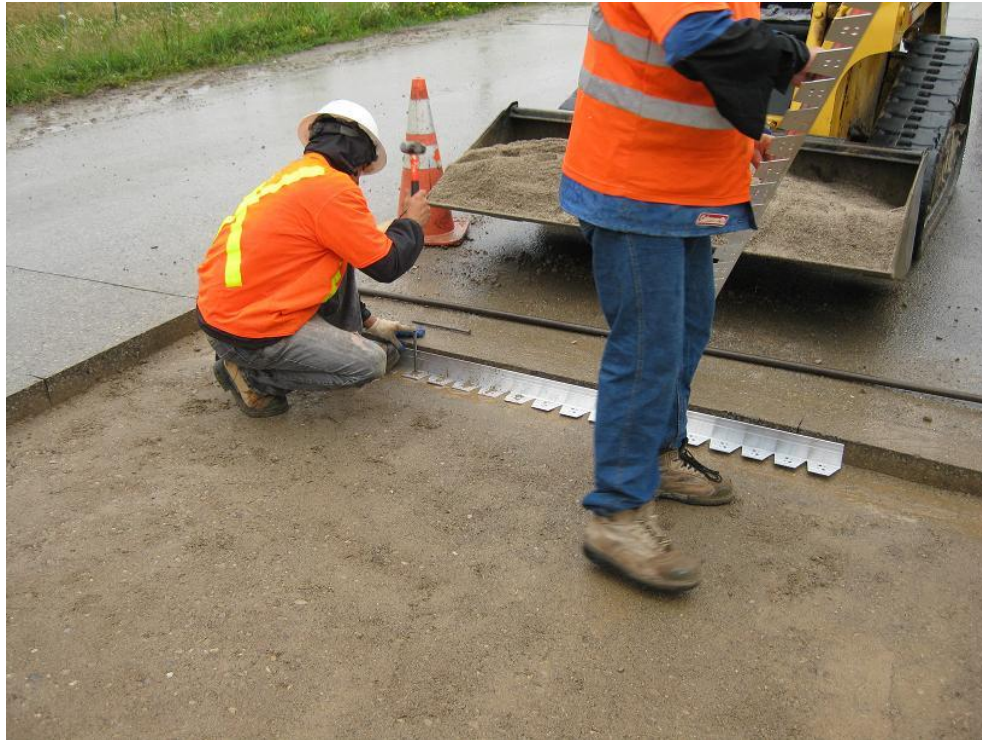
Figure 23 Installation of Aluminum Header
