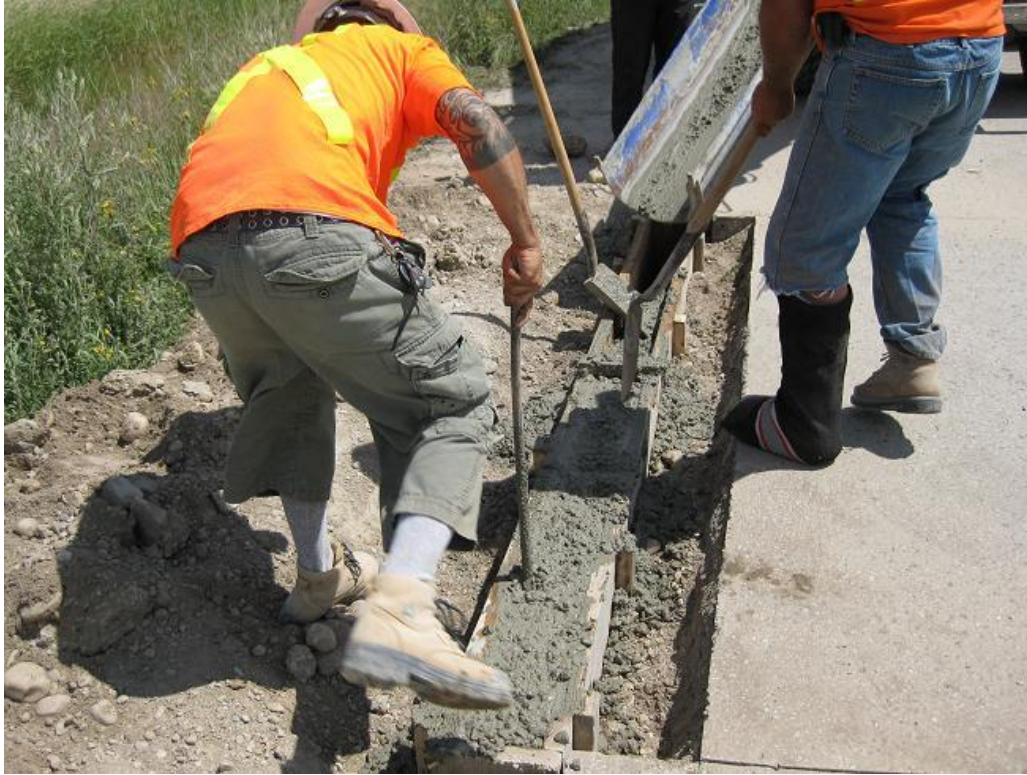
Figure 19 Construction of Curb
