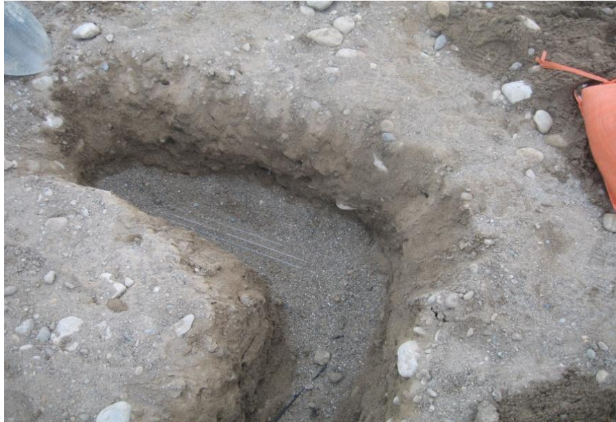
Figure 29 Installation of Moisture Probes in First Phase
