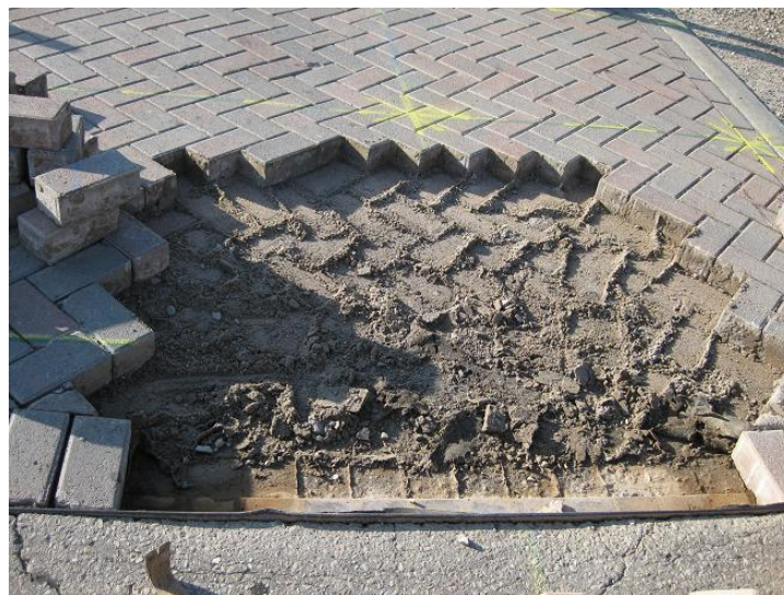
Figure 79 Crosswalk After Lifting the Pavers
