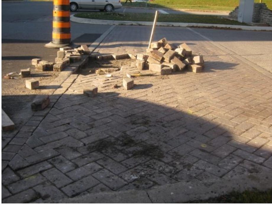
Figure 82 Repair work in Progress SSCBCH
