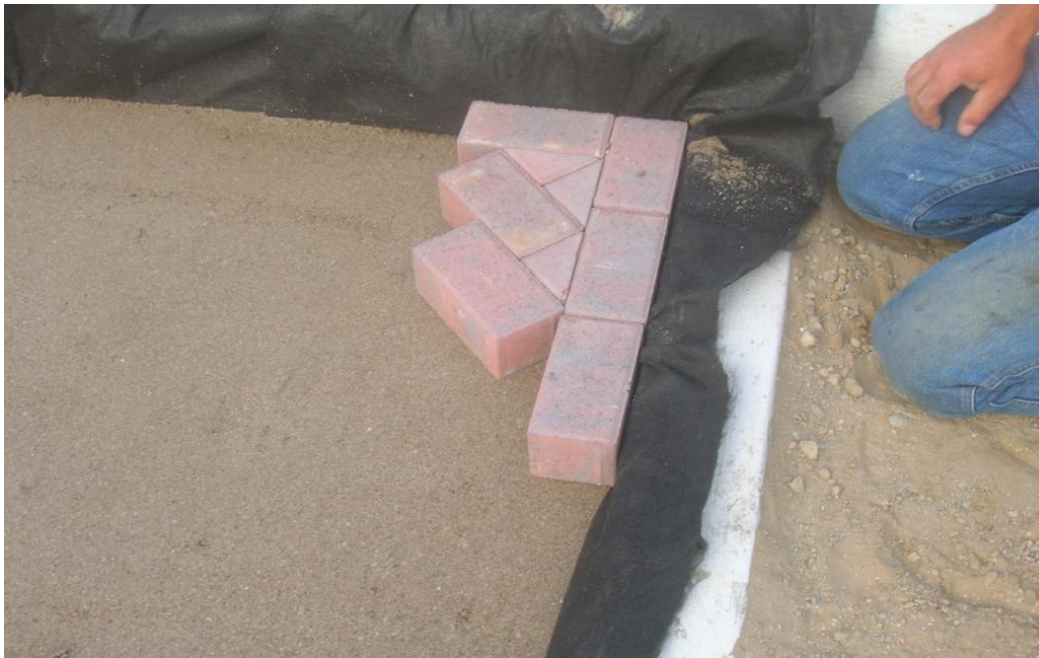
Figure 17 Laying Interlocking Concrete Pavers
