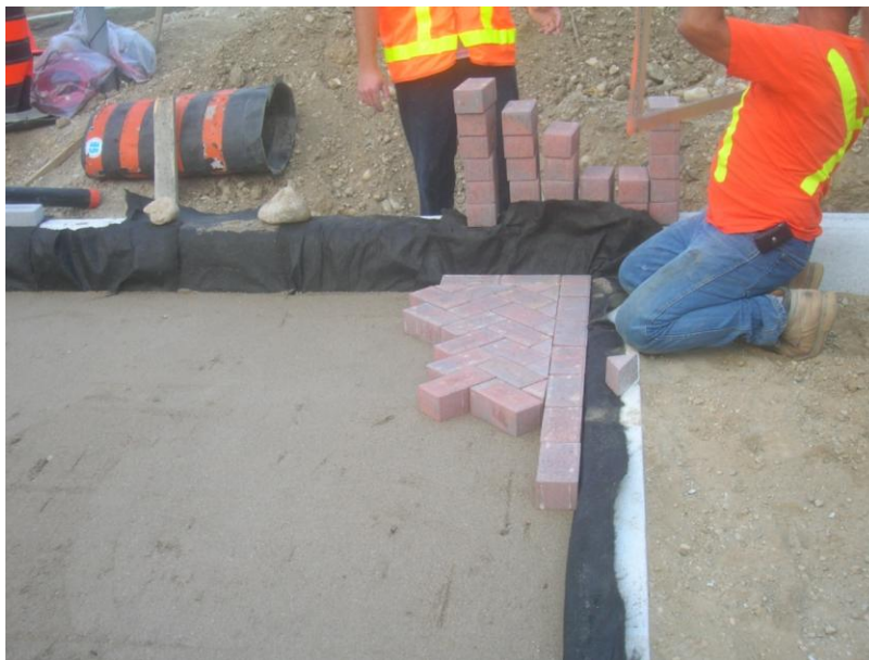
Figure 63 Laying Interlocking Concrete Pavers
