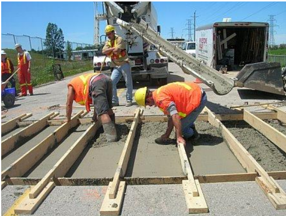
Figure 12 Concrete Placement
