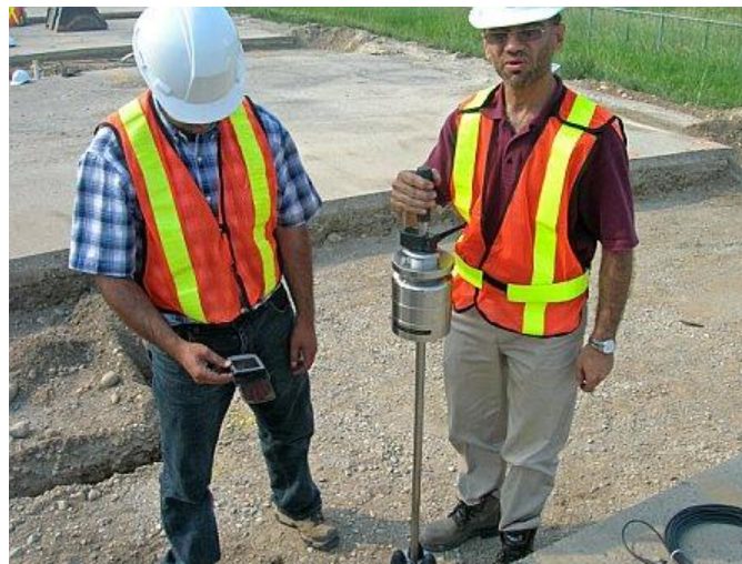
Figure 44 PFWD Testing on Crosswalk Subbase
