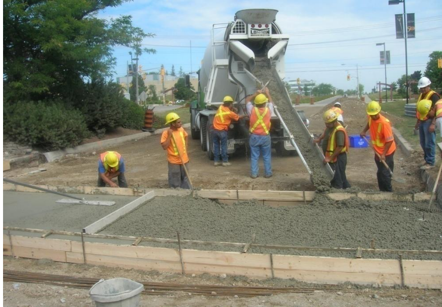
Figure 58 Concrete Placement
