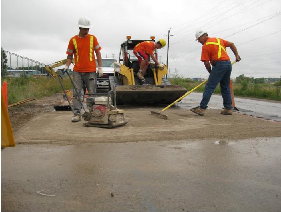
Figure 26 Spreading of Bedding Sand on the Pavers
