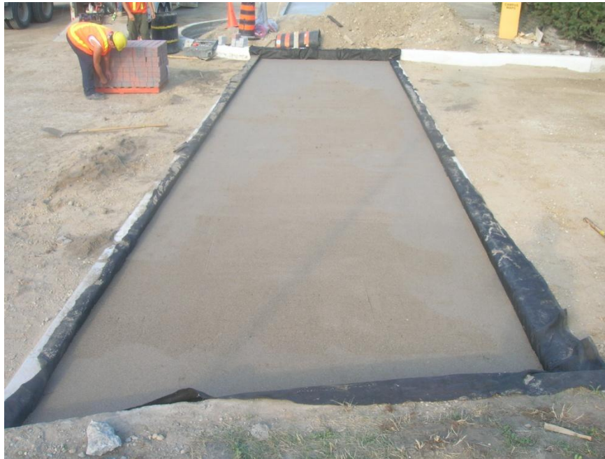
Figure 62 Bedding Sand and Non-woven Geotextile
