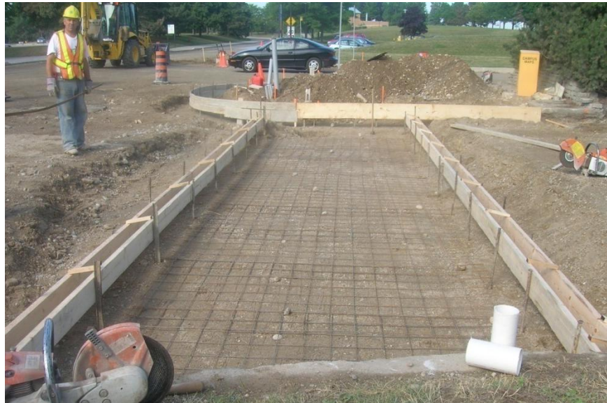
Figure 57 Formworks, Drain Pipes and Reinforcement Bars for Concrete Base Section
