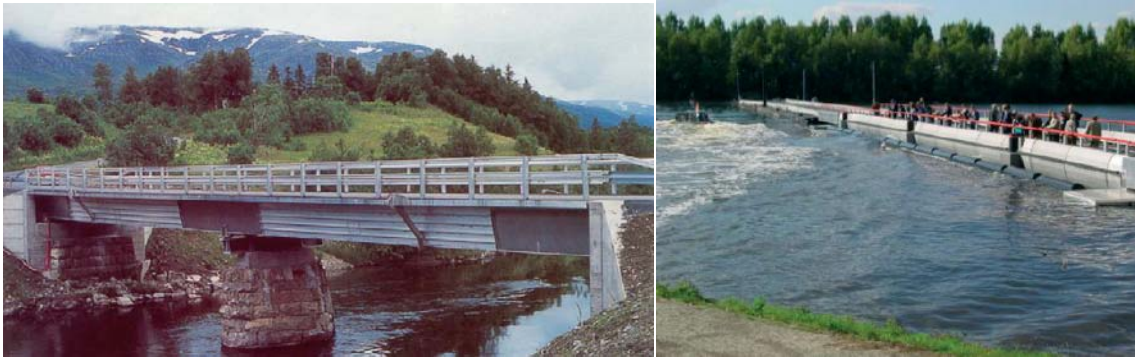
Figure 2.6: All-aluminum bridge in Norway (left) and floating bridge in Netherlands (right) [Siwowski 2006]
