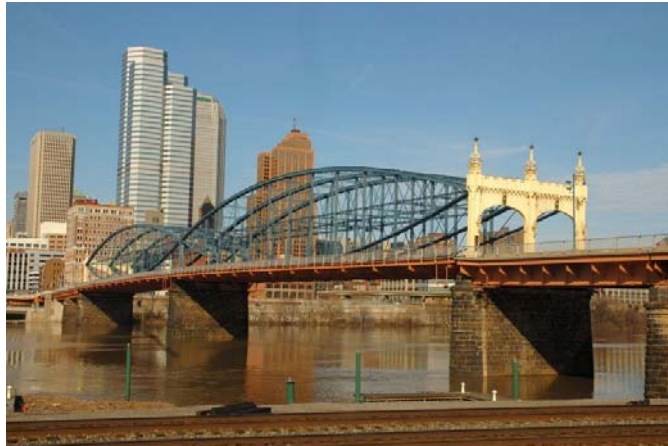
Figure 2.2: Smithfield Street Bridge in Pittsburgh, PA [Hecker 2003]
