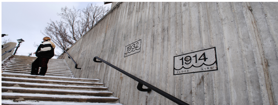
Picture 7- Flood lines, Grand River, Cambridge (Picture taken, Winter 2010)
