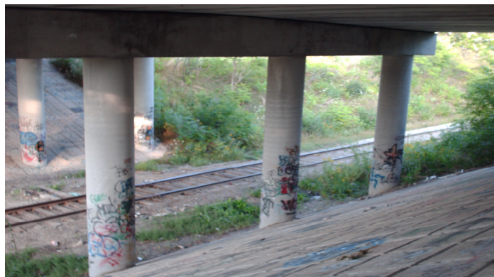
Picture 2- Sterling St. bridge (East Kitchener, Summer 2009)
