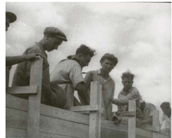
fig. 1.16 Constructing the wall, defining the bounding 'line'
