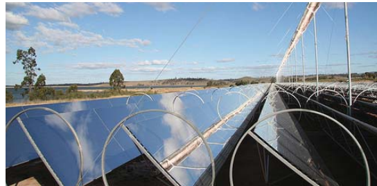
fig. 3.42 Compact Linear Fresnel Reflector
