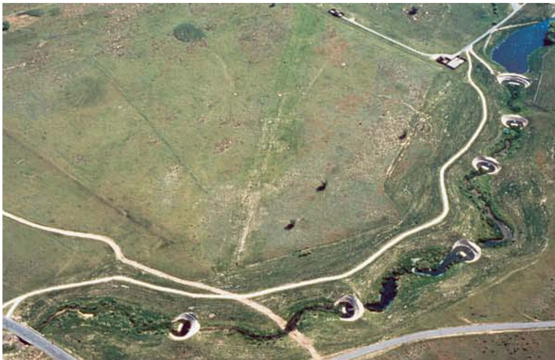
fig. 3.22 Drop structures aerial view
