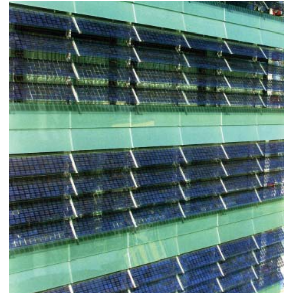
fig. 3.49 Semi-transparent crystalline cells integrated with facade glass slats.
