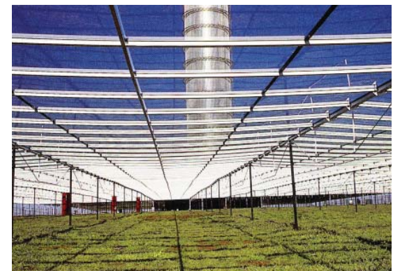
fig. 3.35 Conditions under the collector's glass roof are optimal for greenhouses
