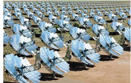
fig. 3.40 Parabolic dish and heat engine
