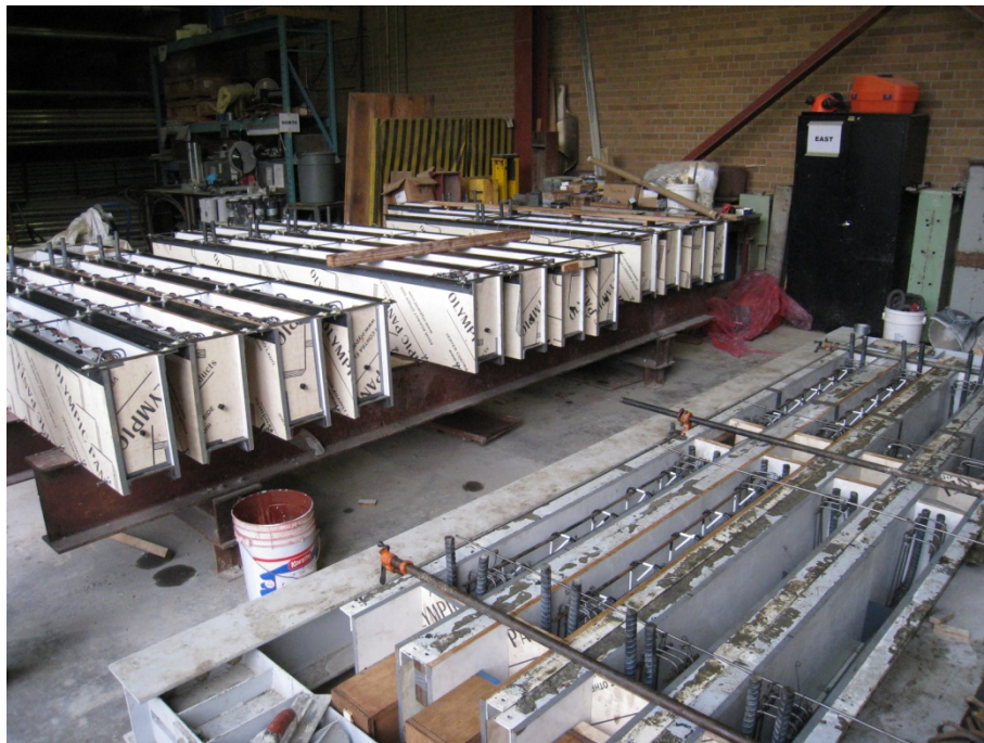
Figure 3.5: Formwork with cages
