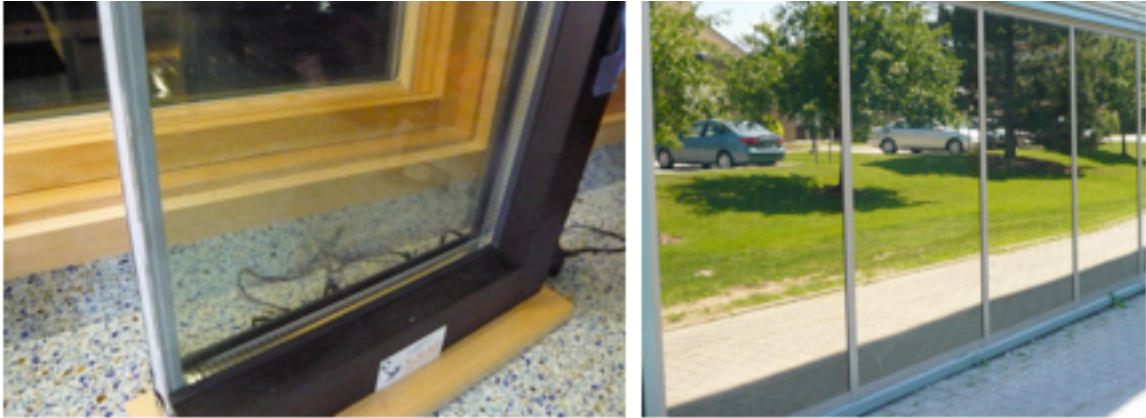
Figure 2.2.1 Photographs of electrochromatic IGU (left) and tinted glazing (right)
