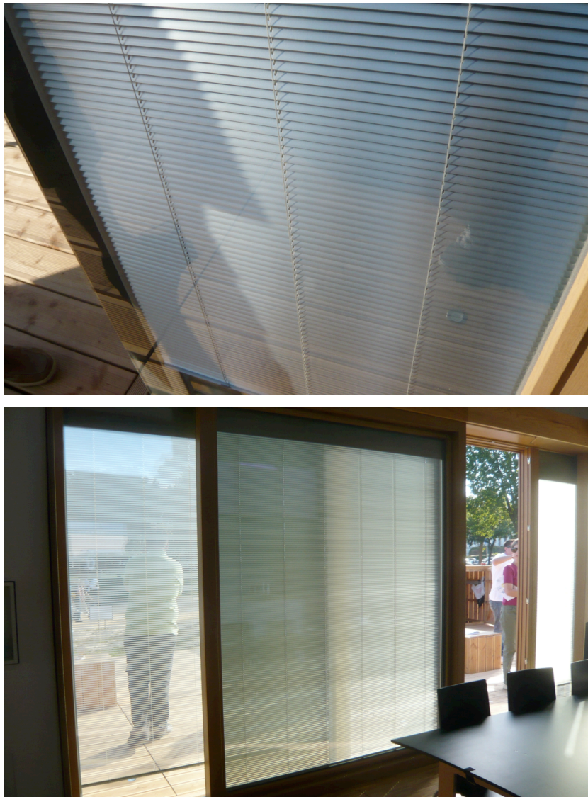
Figure 2.2.3 In-between blinds from SurPlus Home, Team Germany 2009 Solar Decathlon. Top: exterior view, bottom: interior view
