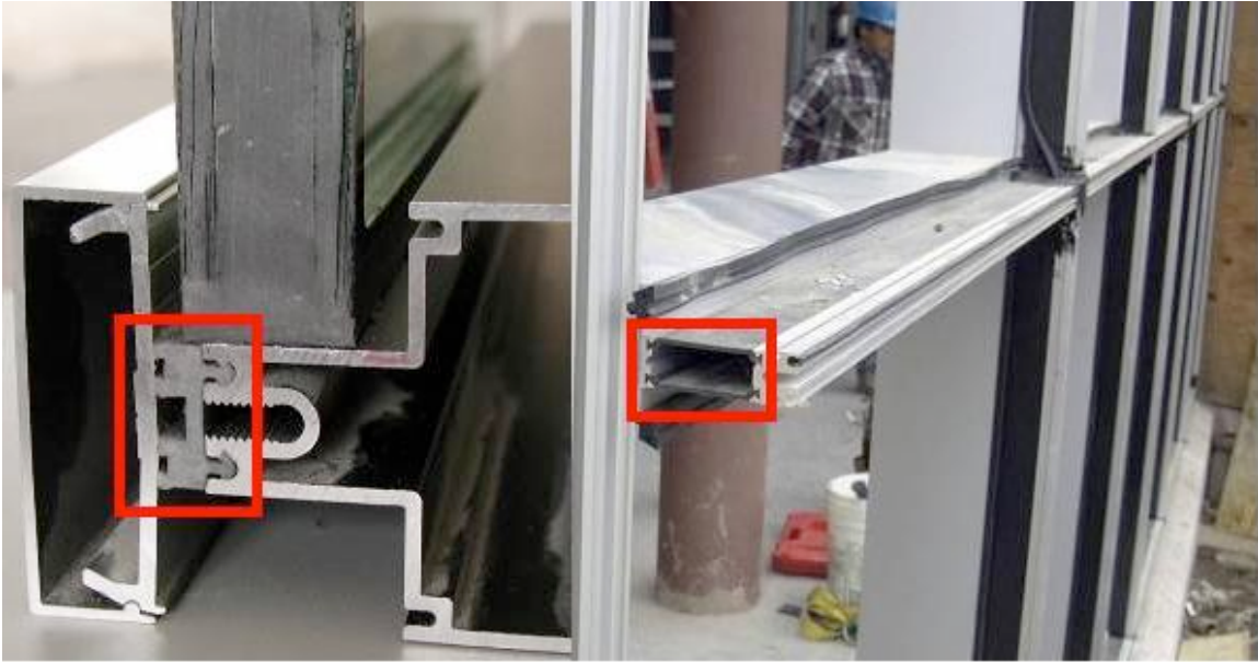
Figure 4.1.3 Thermally broken aluminum curtain wall sections (Left: Kawneer 1600 curtain wall section, Right: Kawneer 7550 curtain wall section)
