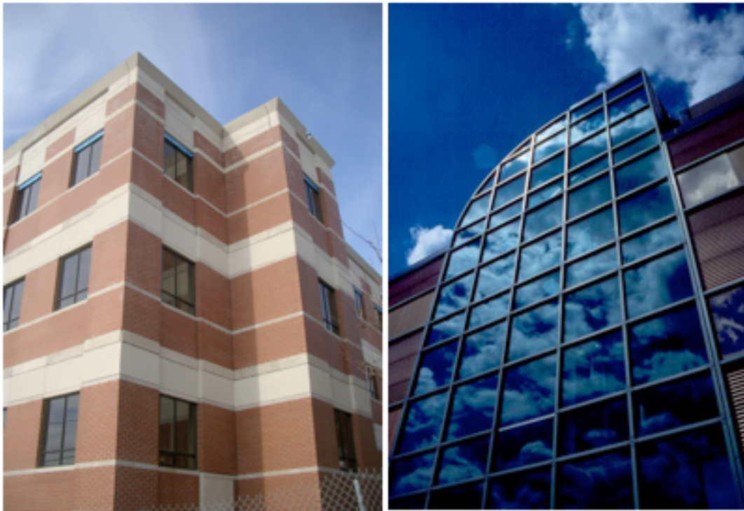
Figure 2.1.2 Buildings with punched windows and curtain-wall systems (Lstiburek and Straube, 2008)
