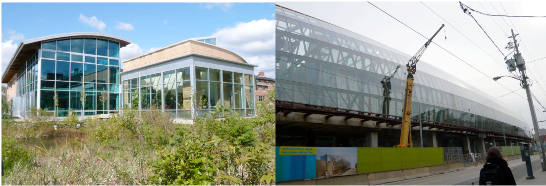
Figure 4.1.1 Buildings with curtain wall system (Left: Adam Joseph Lewis Center for Environmental Studies, Oberlin College, Right: Art Gallery of Ontario)
