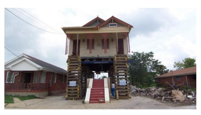
fig. 84: An Elevated Double Shotgun House
