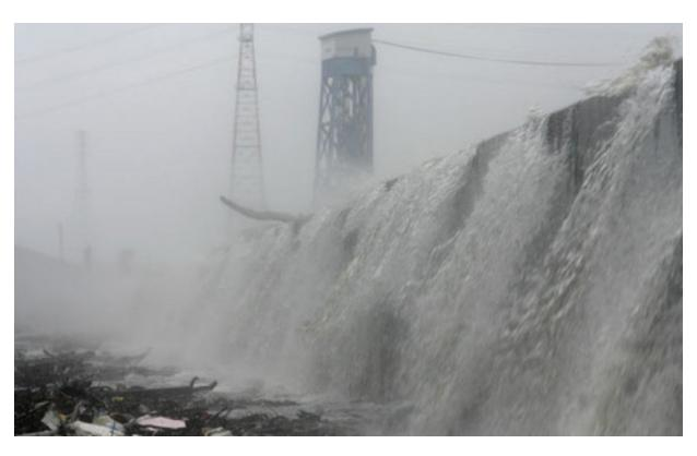
fig. 40: Levee Overtopping at the Industrial Canal
