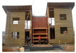
Day 66 – "You will notice in Photo25...the house on the right is higher than the left.. its floating!" (this has the recapped plastic bottle buoyancy blocks)
