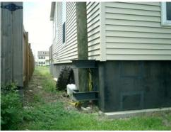
Figure 5: Lakeview House, New Orleans. Elevation and detail of connection to post.
