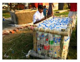
Buoyancy blocks made of recapped empty plastic bottles
