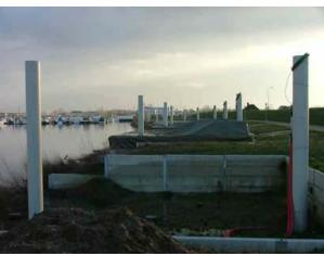
all components are ready to receive the first concrete box foundation for the amphibious house
