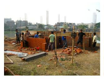
fig. 218: Construction Team Assembling Masonry Wall
