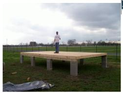
Setting the vertical guidance posts (Note post design has since been changed to telescoping posts)
