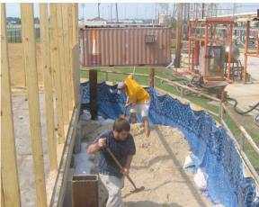
A layer of sand holds down the tank liner
