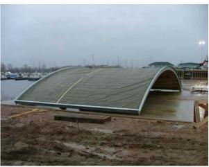
the prefabricated roof is assembled on site
