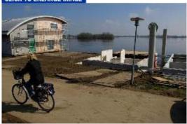
Associated Press photo by PETER DEJONG Metal pylons, right, stand between the foundations of amphibian houses under construction in the central Dutch village of Maasbommel, Netherlands, southeast of Amsterdam. The houses, attached to pylons, stand on solid ground, but float if water levels rise.
