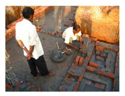
Starting the brick walls for the composting latrines and rainwater storage cisterns
