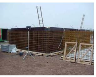
concrete walls of each box are reinforced with steel
