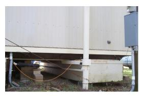
fig. 124: Detail of Amphibious Foundation
