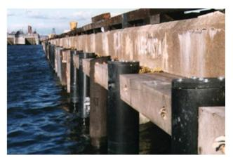
fig. 238: Thermoplastic Timber Pilings
