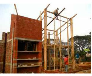
fig. 221: Bamboo Structure in Place beside Concrete Spine, Perspectival View
