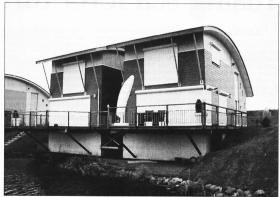
This house in a flood-prone community in the Netherlands has a 'buoyant foundation' to reduce flood damage. The system works like a floating dock.
