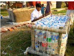
Figure 7: The LIFT House in Dhaka, Bangladesh. Concrete and brick base structure under construction; buoyancy block made of recapped, recycled plastic bottles.
