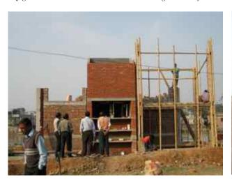
fig. 220: Bamboo Structure in Place beside Concrete Spine
