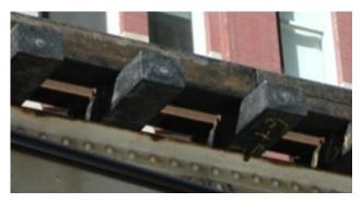
fig. 248: Elevated Rail in Chicago Using Thermoplastic Ties
