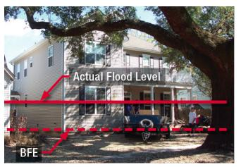
fig. 108: Flood Level Exceeded BFE
