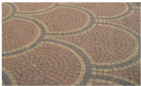
1 existing paving Fig. 4.22
