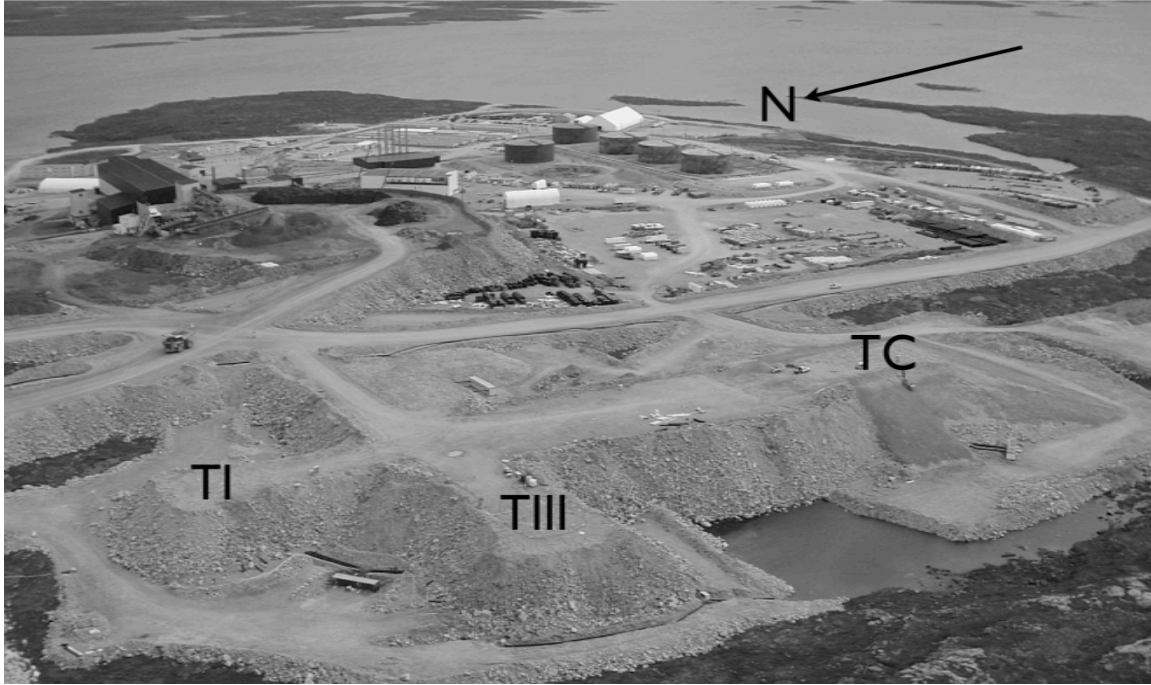
Figure 2 - 1: Aerial photo of the Diavik test-pile waste rock research area.
