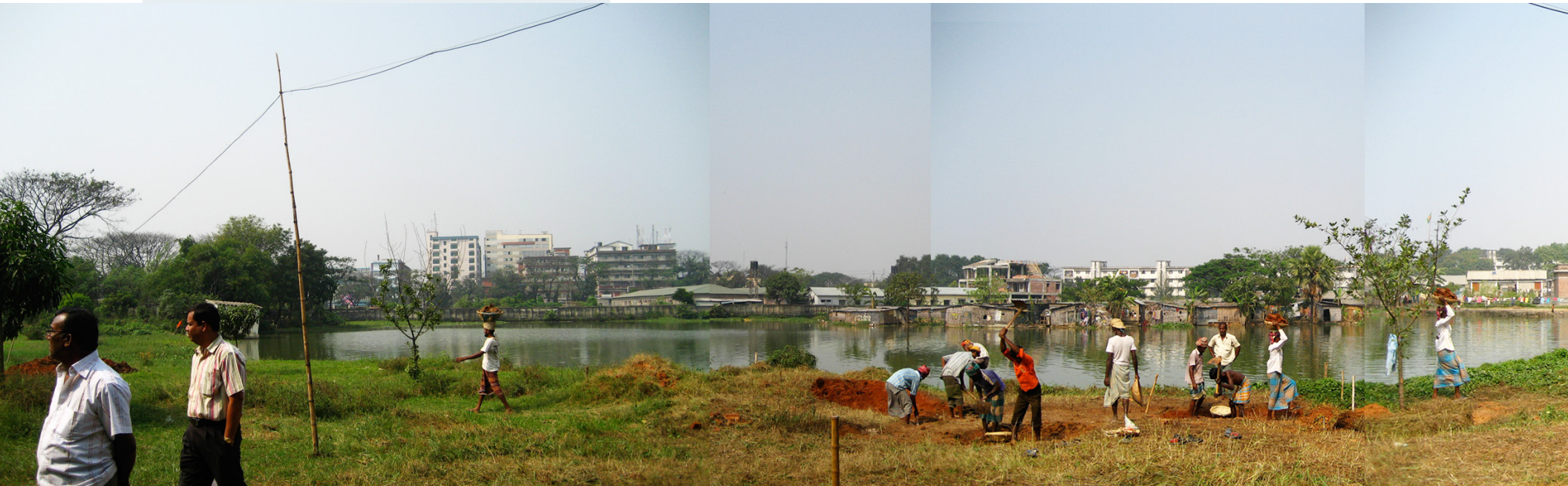
8.16. Workers excavating the site manually
