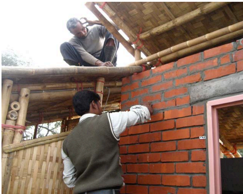
8.145. Installation of toilet roof 8.146. (opposite) The LIFT house complete
