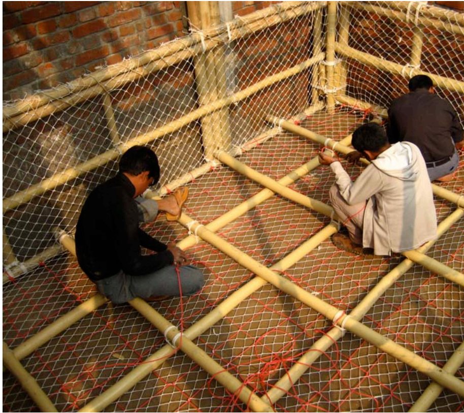
8.91. Bamboo frame with nylon net for water bottle foundation
