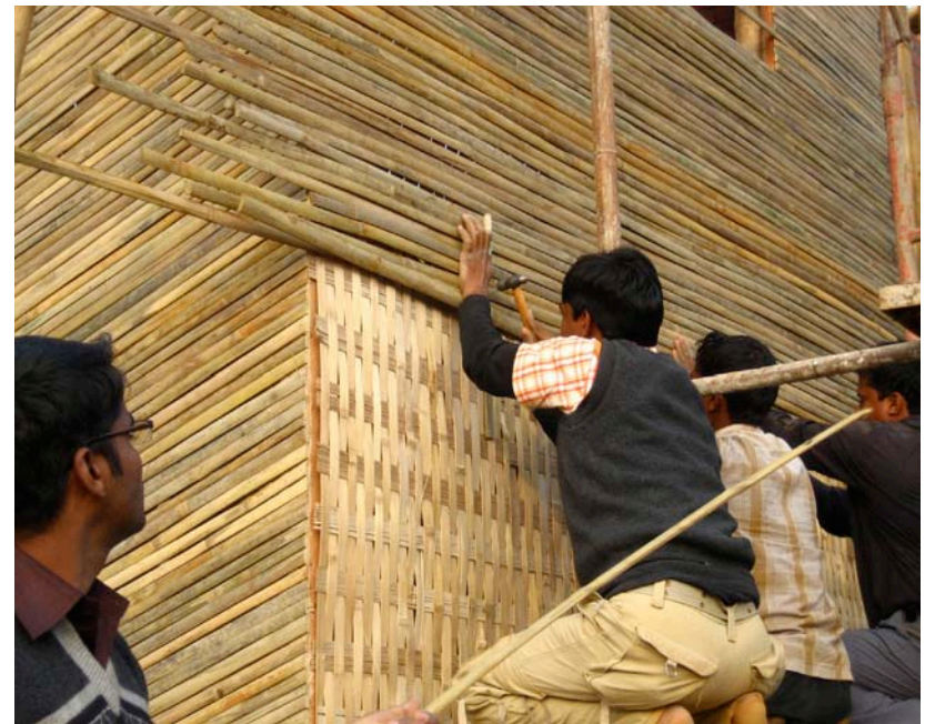
8.132. Installation of Mulli bamboo strips as wall finish
