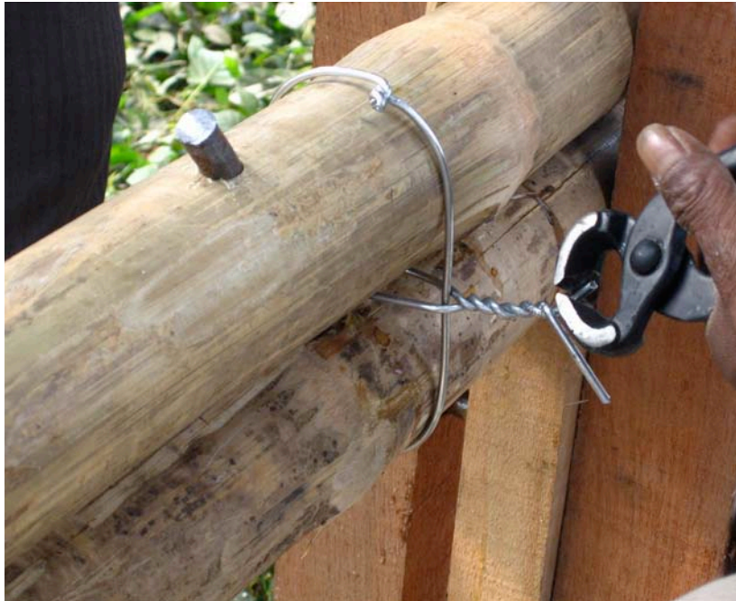
8.73. Metal wires tied around steel rod insertion in bamboo beams
