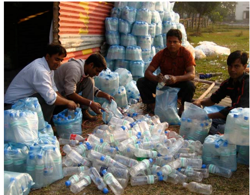
8.89. Used water bottles prepared for foundation by volunteers
