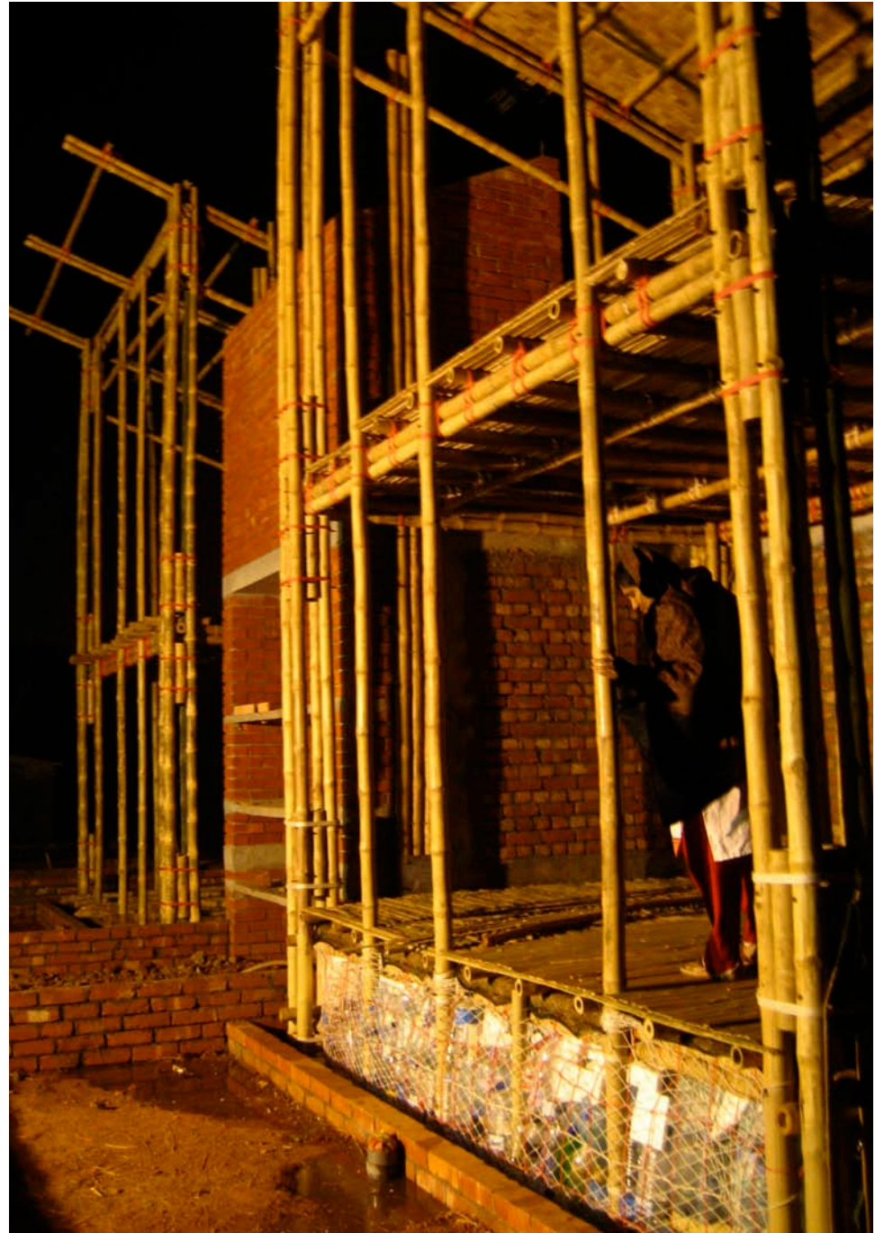
8.111. Water bottle foundation dwelling in buoyant state
