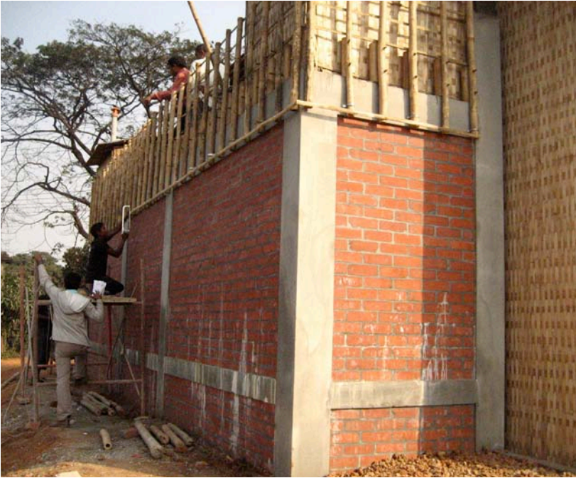
8.140. Railings being secured
