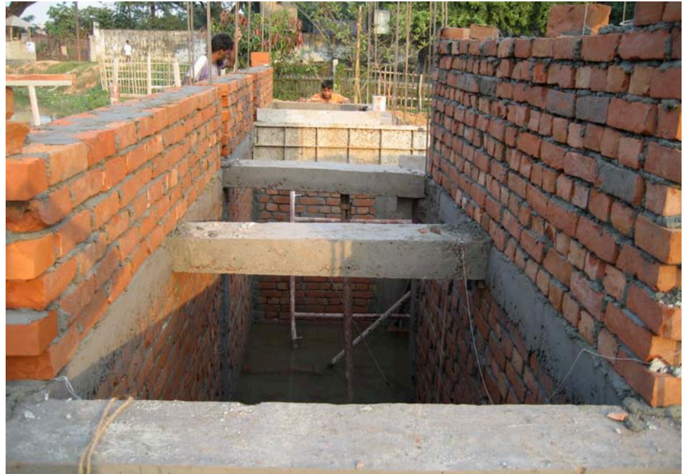
8.49. Lintels for lateral support inside the water cisterns in the service spine
