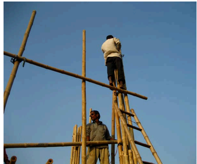
8.85. Installment of top beams
