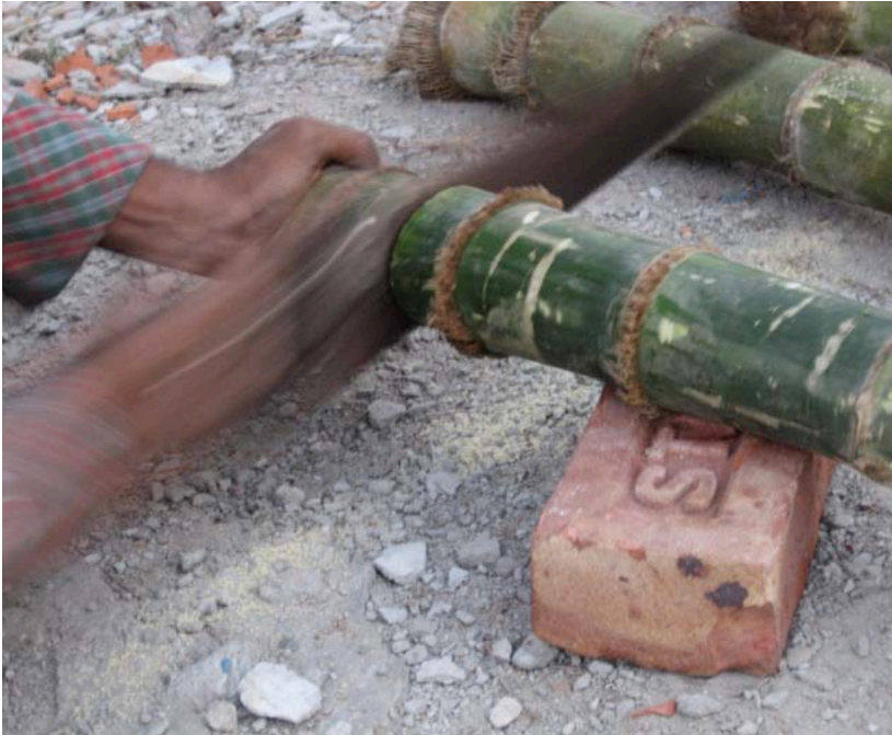
8.45. Bamboo cut by hand saws
