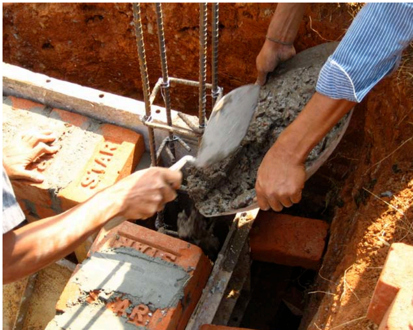
8.30. Concrete poured into gaps left for columns in the brick walls of the service spine
