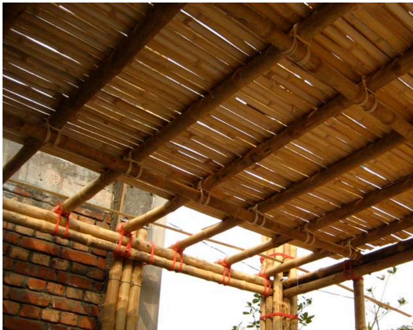
8.97. Underside of second floor
