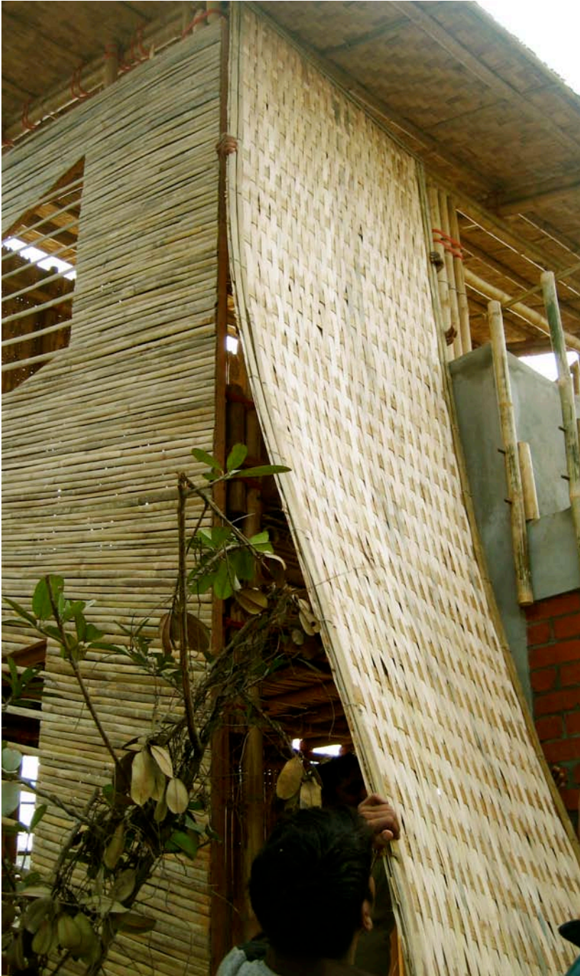
8.135. Installation of interior wall
