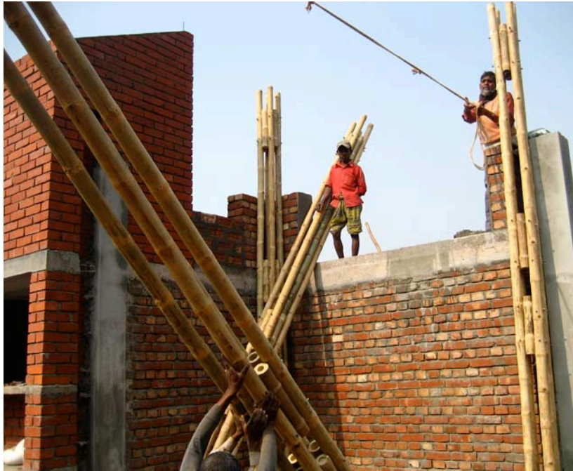
8.79. Bamboo columns carried to position
