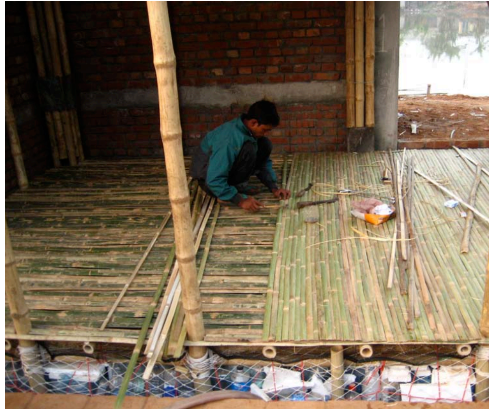
8.90. Jawa bamboo pieces layed in two layers for floors in dwelling
