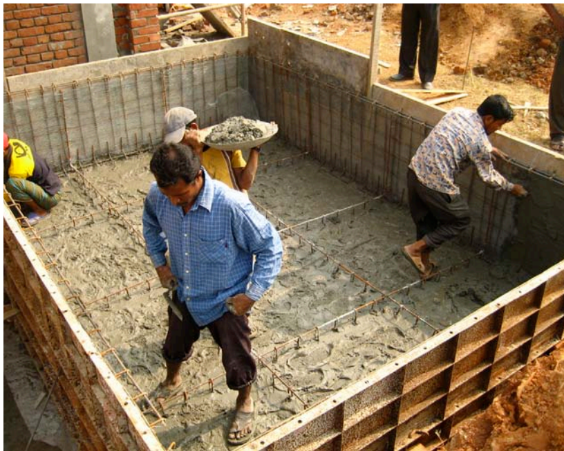
8.62. Cement mixture poured into frame and compressed
