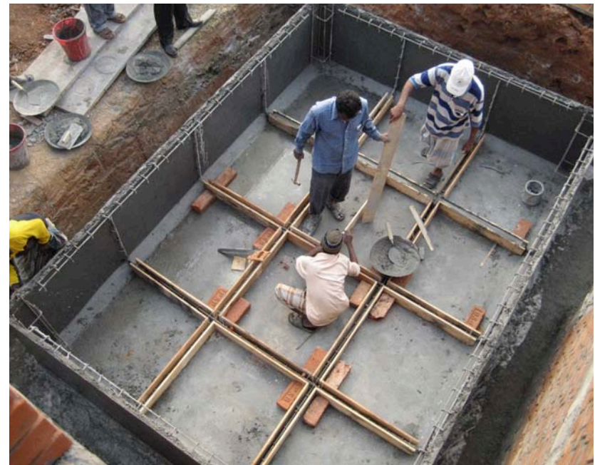
8.64. Shutters laid for concrete ribs
