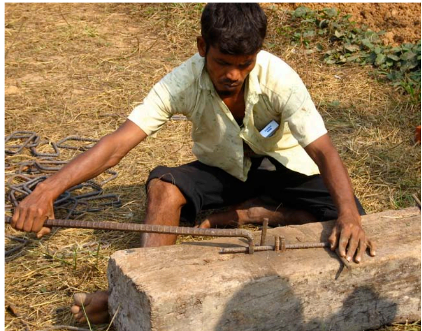
8.48. Worker bending dowels
