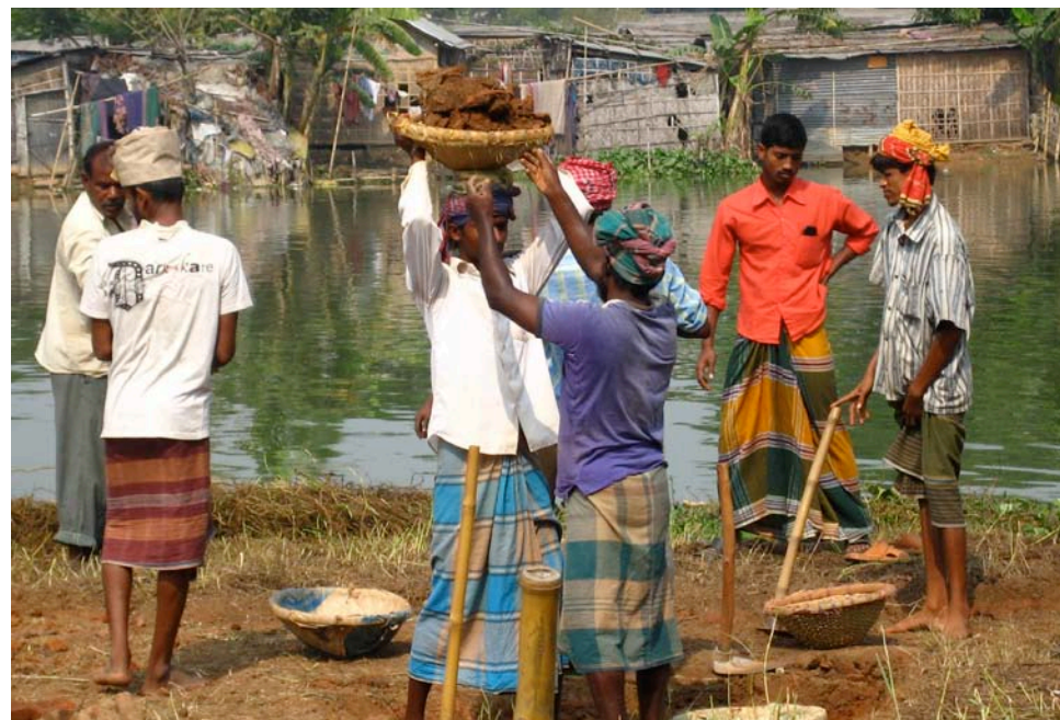
8.17. Excavators using bamboo baskets to move the soil
