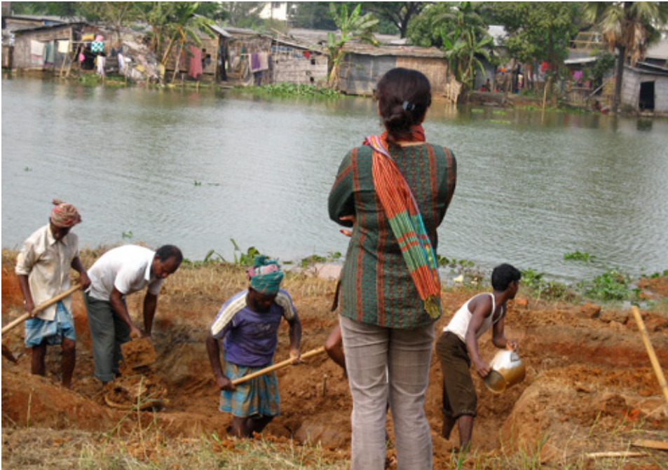
8.14. Beginning of excavation
