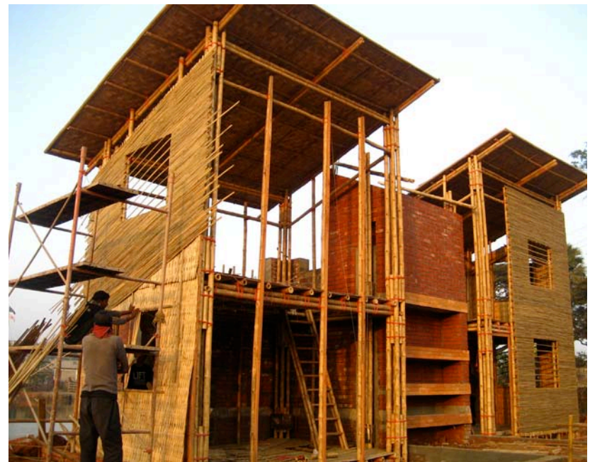
8.137. Installation of side walls
