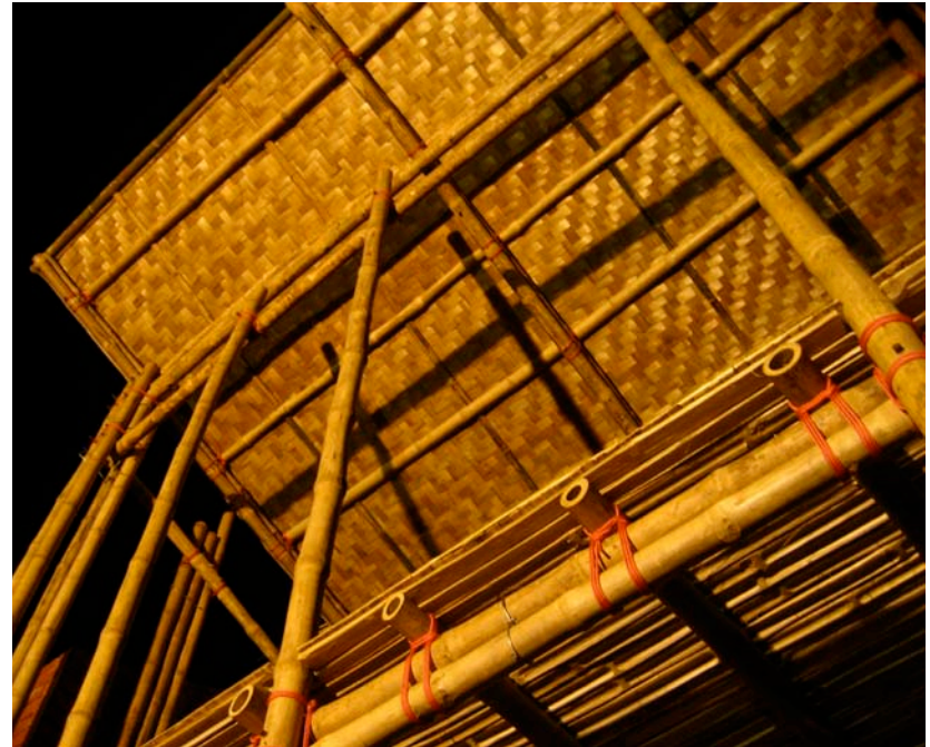
8.113. Bamboo frame with roof
