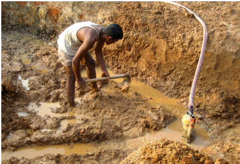
8.18. Water being pumped out of the excavated area
