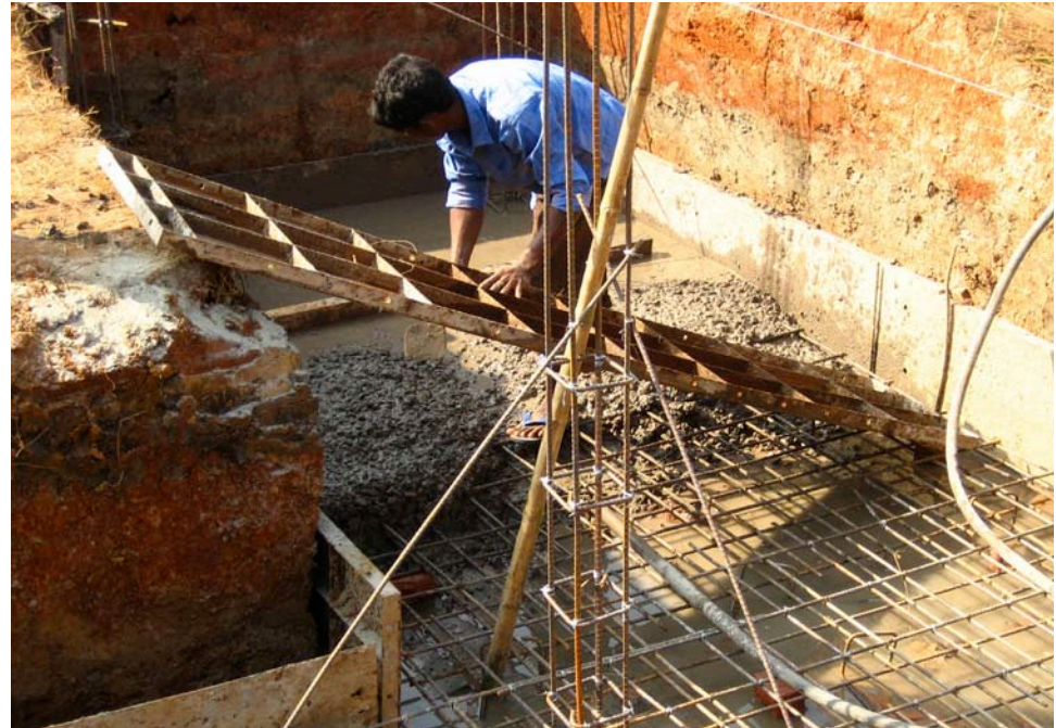
8.27. Worker pouring service spine floor slab
