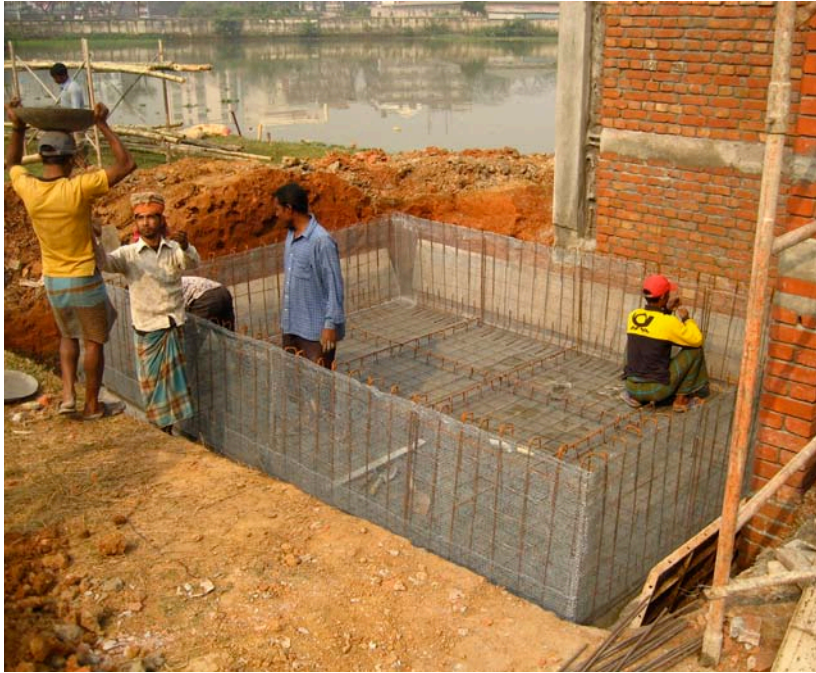
8.61. Ferrocement foundation placed into holding tank
