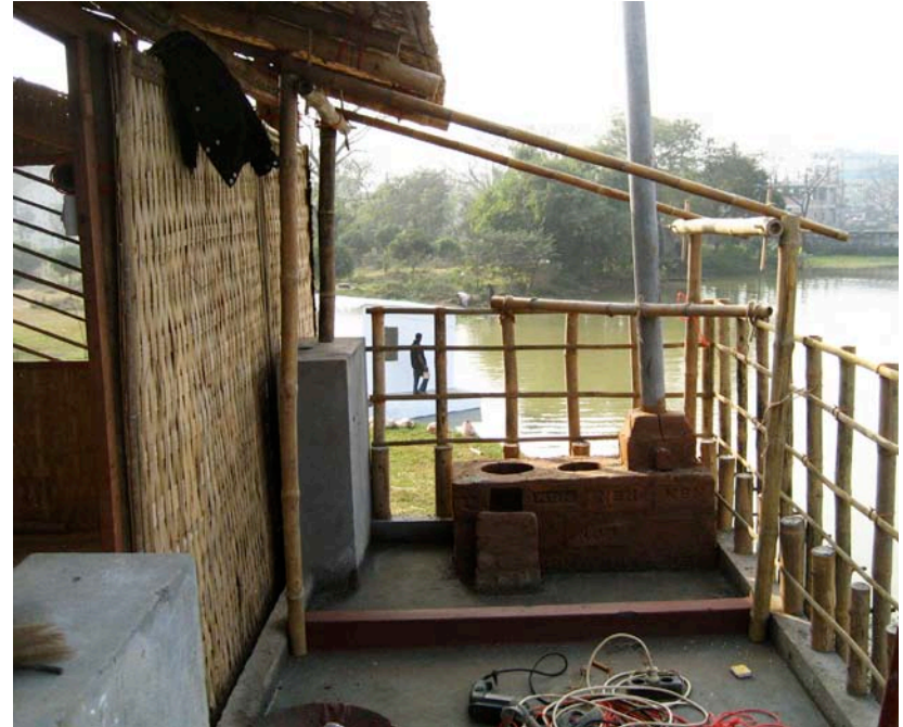
8.136. Bamboo frame for kitchen on top of service spine
