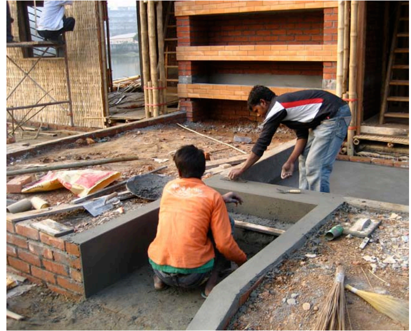
8.131. Construction of front steps
