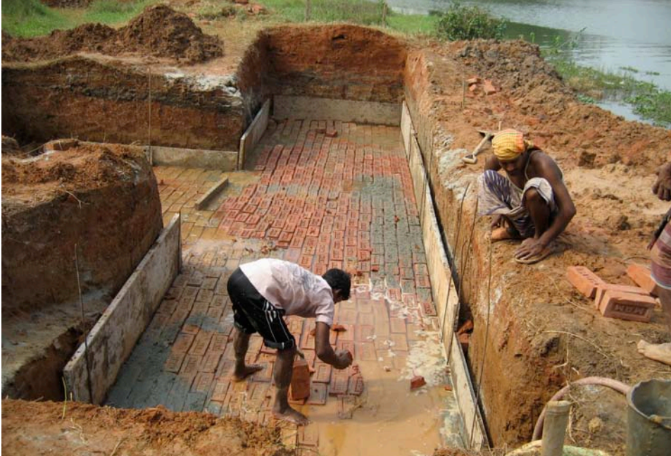
8.21. Brick soiling prepared for concrete slab
