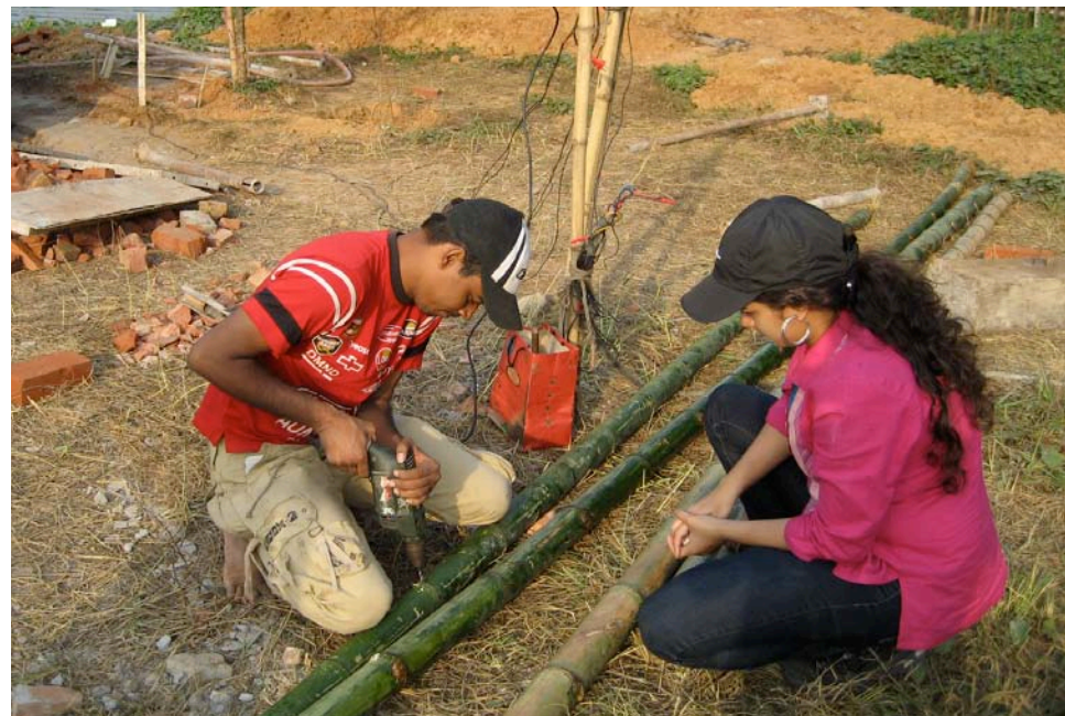
8.44. Bamboo drilled at every joint by a volunteer
