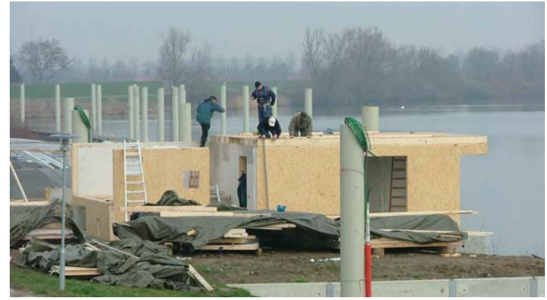
5.7. Ground floor completed of the amphibious houses
