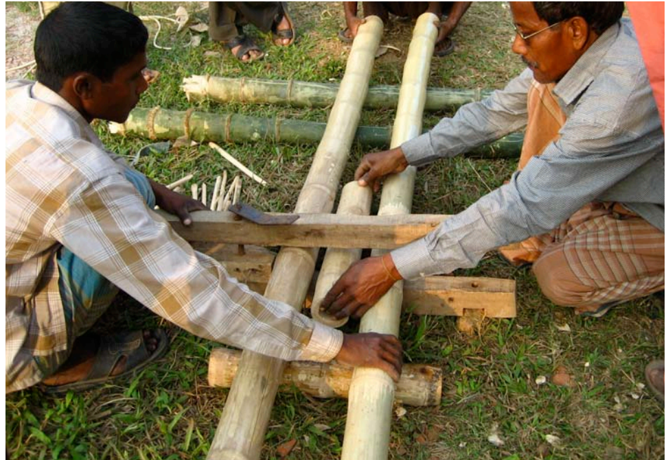
8.71. Bamboo placed in wood clamps to straighten the bamboo before joining
