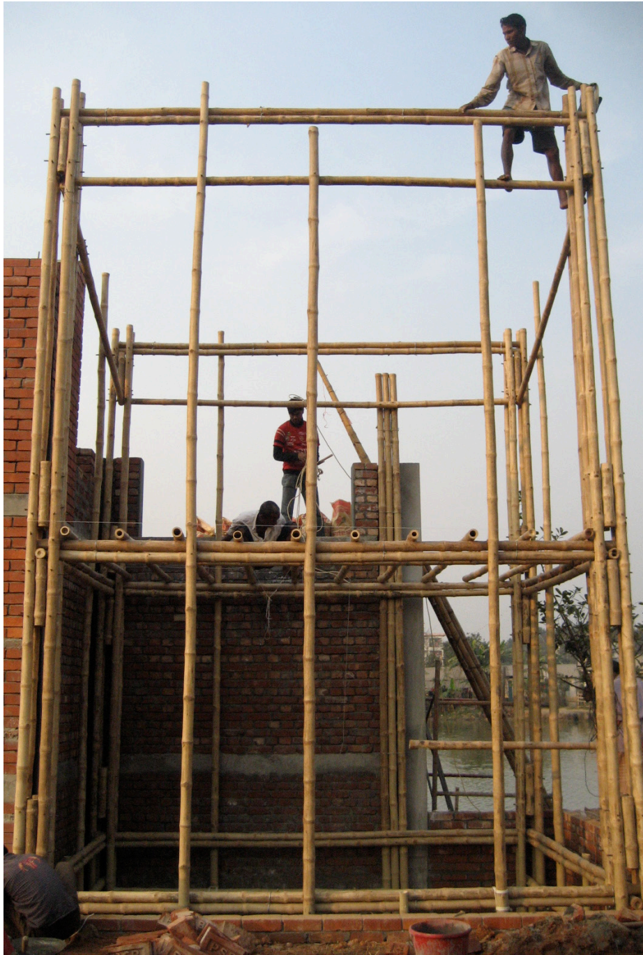
8.83. Structural frame for water bottle foundation dwelling
