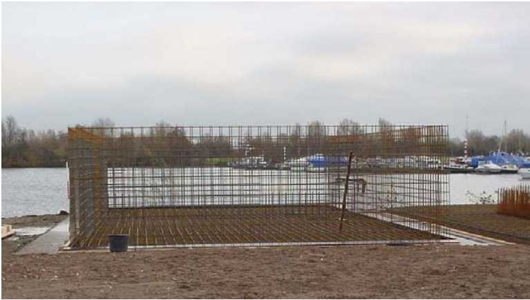
5.4. Reinforcement for the amphibious foundation
