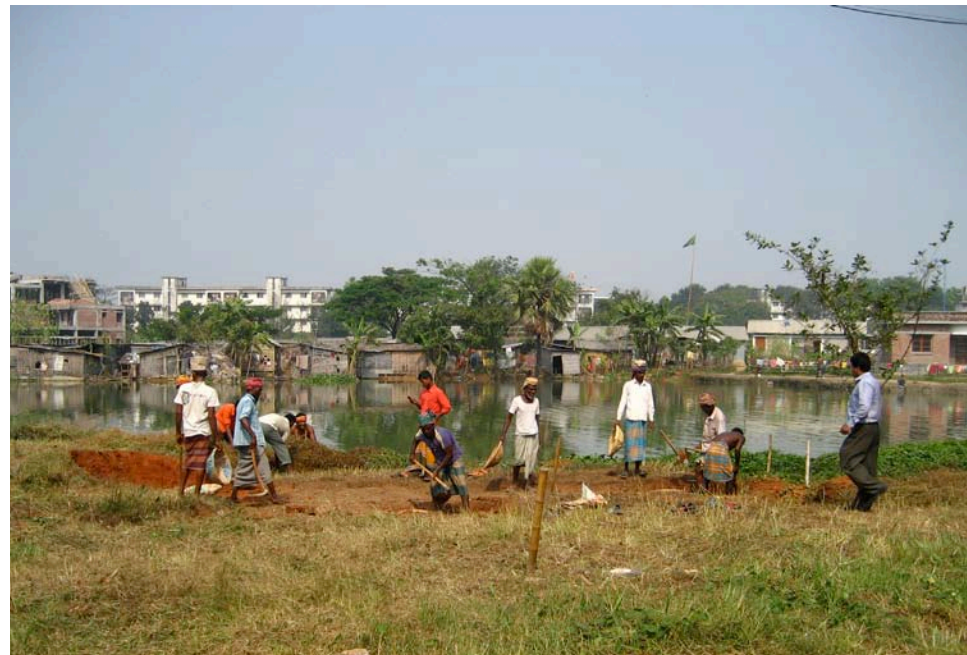
8.1. Excavation for the LIFT house service spine
