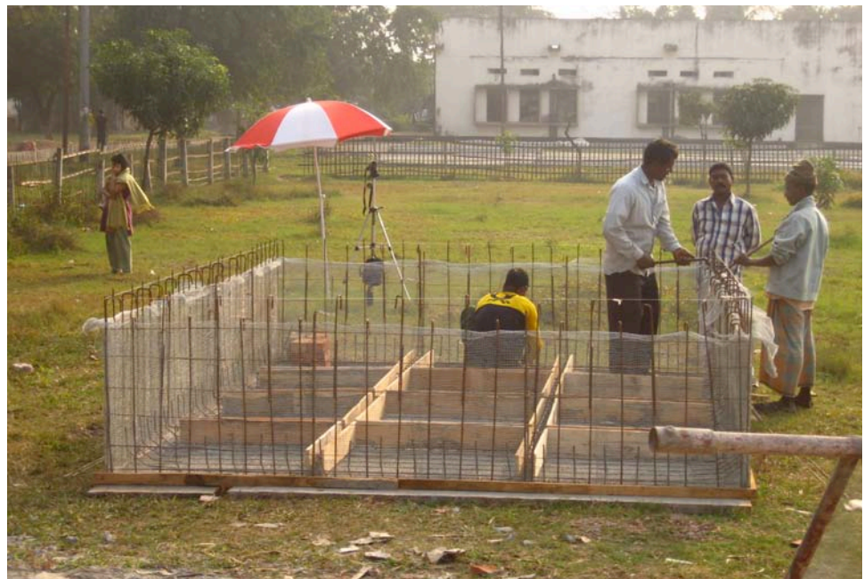
8.60. Ferrocement foundation structural frame
