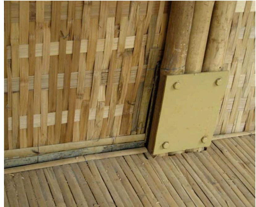
8.147. Steel plate attaching dwelling to vertical guidance system
