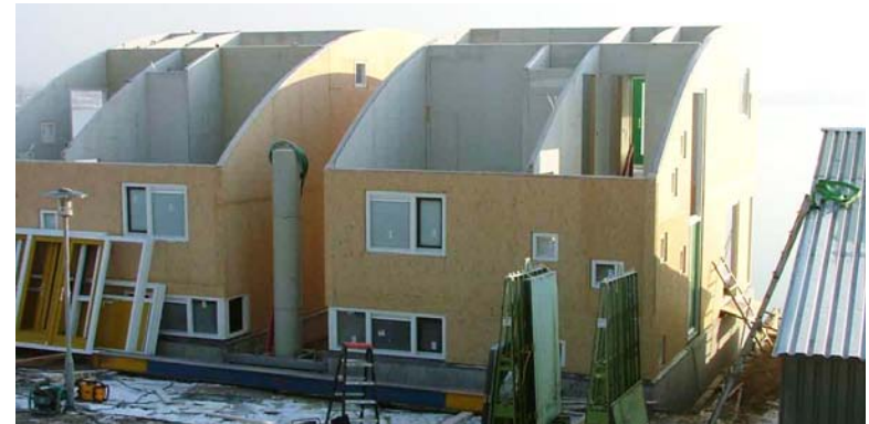
5.8. The two houses sit on a shared platform that allows them to float together
