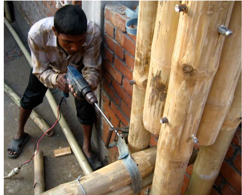
8.81. Connection of bamboo beam and column
