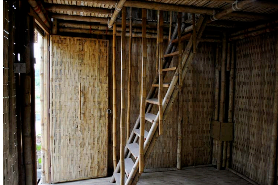
8.134. Interior stairs made of bamboo and wood
