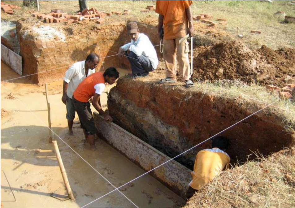
8.20. Shutters placed around the perimeter in preparation for concrete pour
