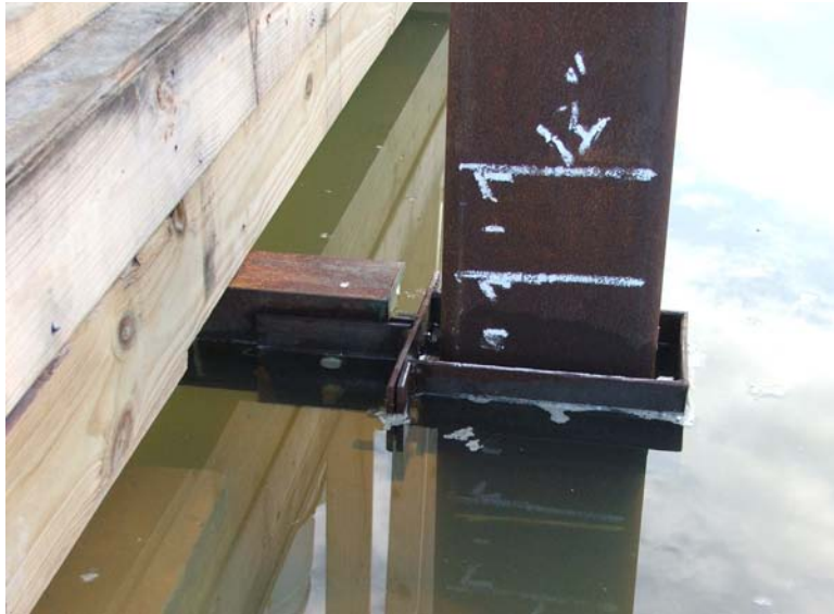
5.10. Vertical guidance system for the LSU prototype
