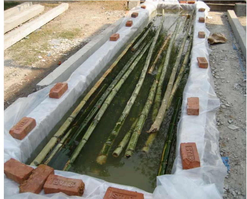
8.47. Chemical treatment of the bamboo before installment
