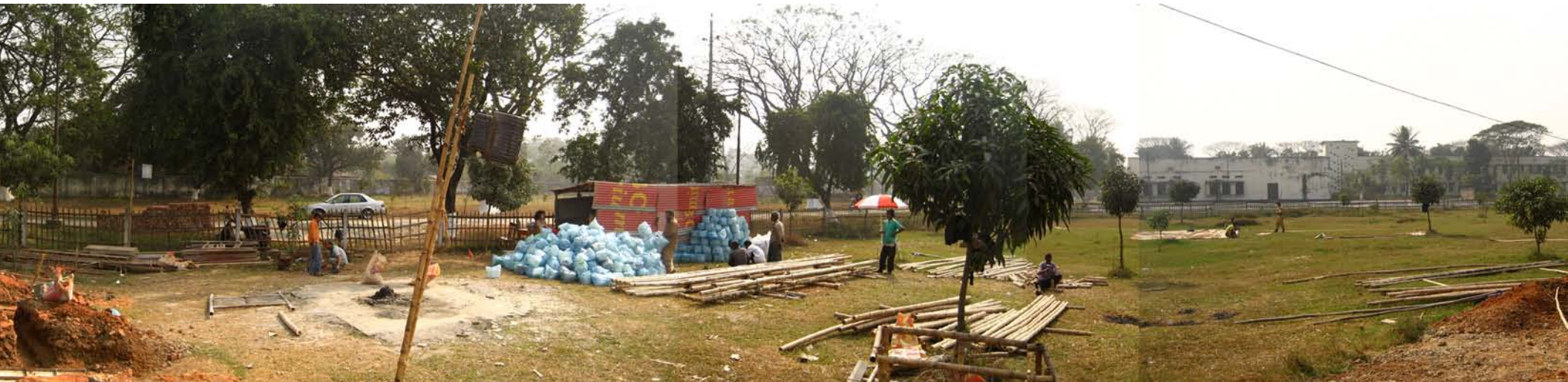
8.93. Panoramic photo of the LIFT construction site
