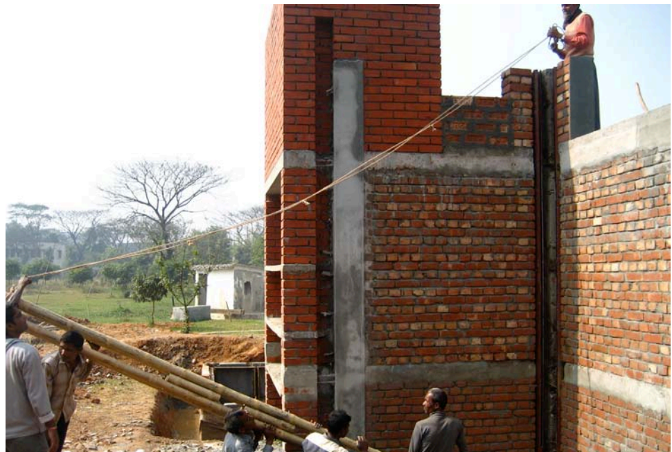
8.78. First column pulled into place
