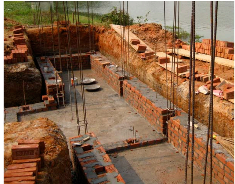
7.1. Perimeter brick wall under construction
