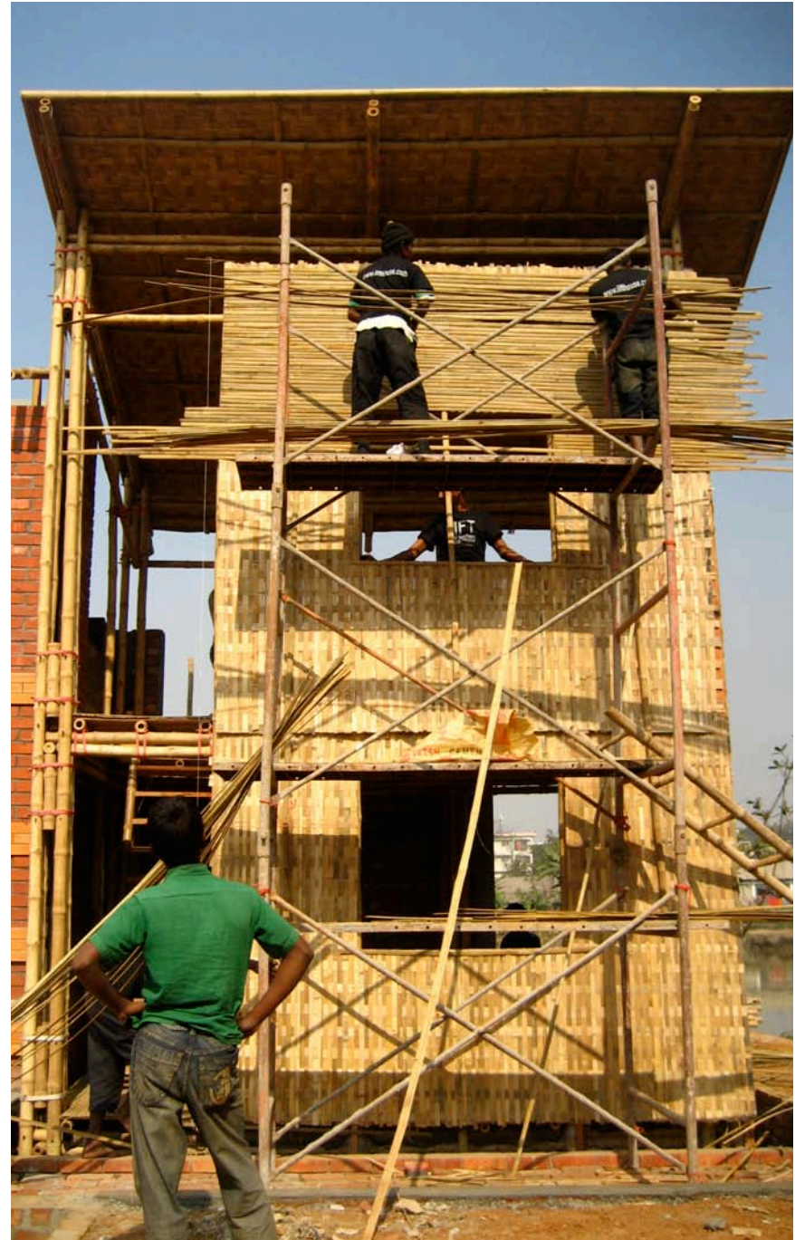
8.126. Installation of front wall finish
