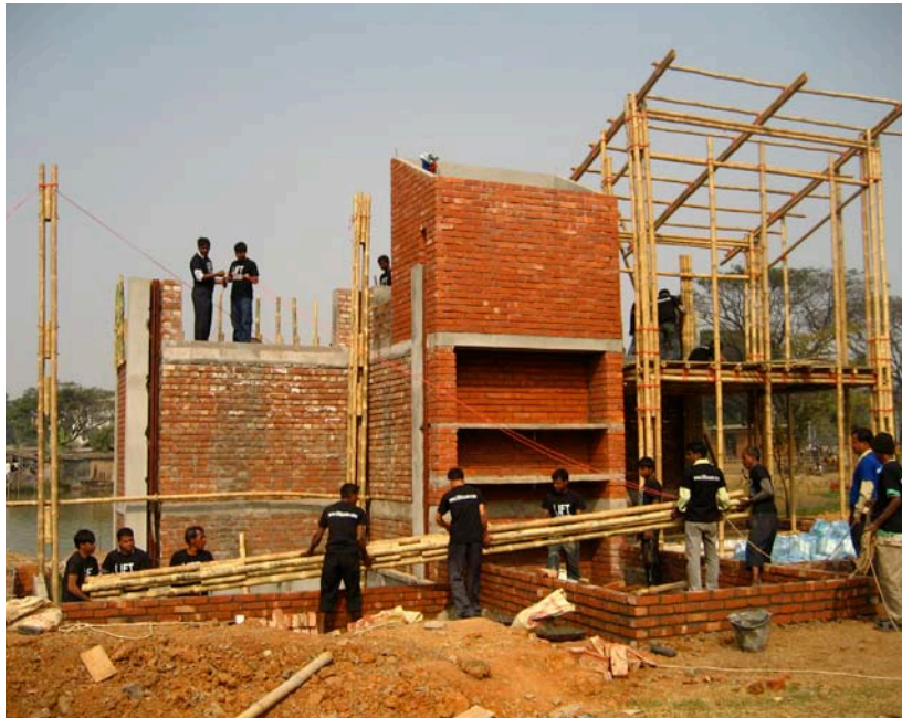
8.105. Second bamboo frame under construction
