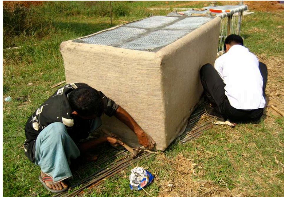
8.39. Second foundation model wrapped in metal wire and cotton cloth
