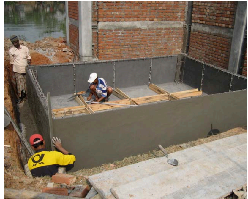
8.63. Cement mixture laid on both the outside and inside face of the foundation
