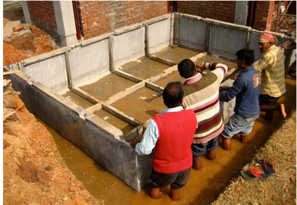
8.94. Ferrocement foundation moved into position after curing
