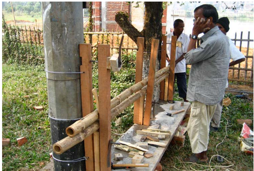
8.72. Method of creating beams
