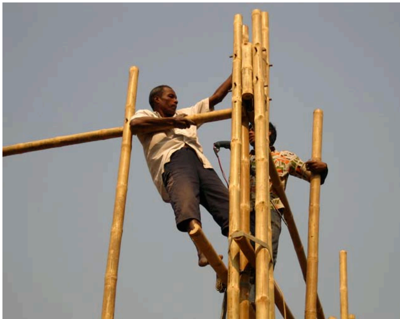
8.80. Beams attached to columns by bamboo workers
