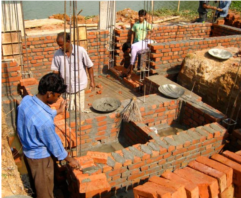
8.29. Walls of the service spine around the composting latrine storage pits
