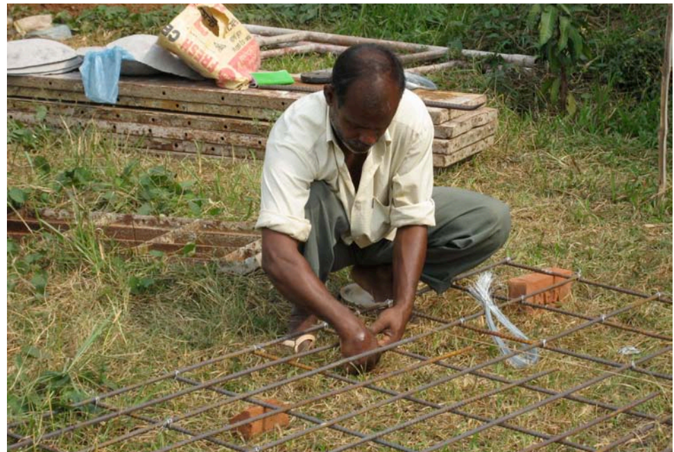
8.23. Reinforcing bars prepared for concrete slab
