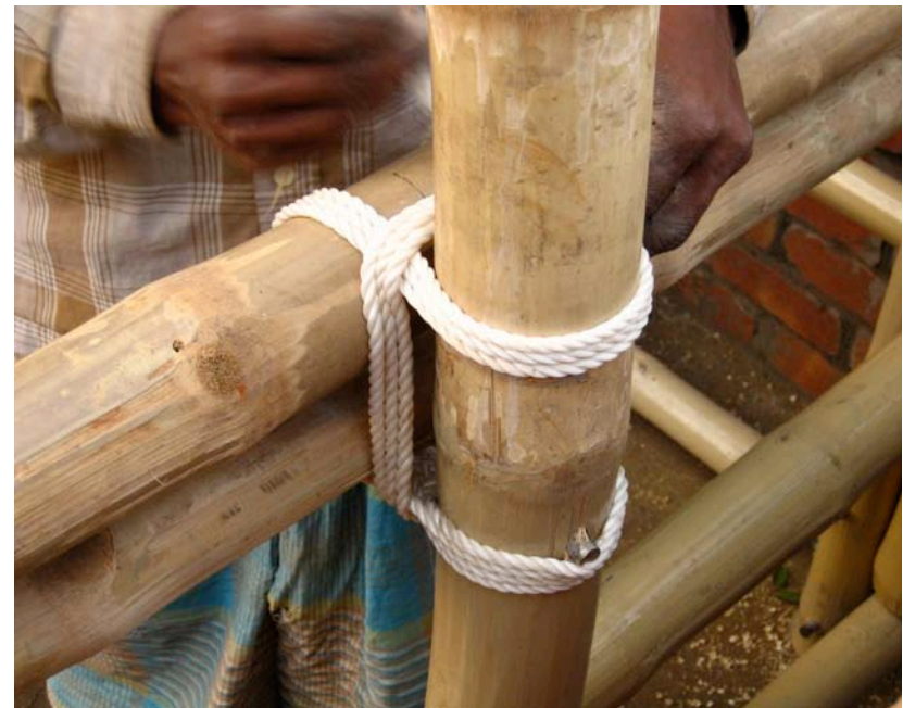
8.82. Nylon tied around bamboo connection
