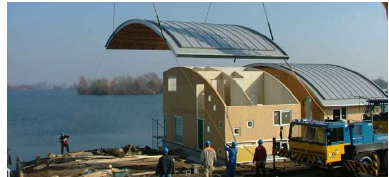
5.9. Roof installation on amphibious houses
