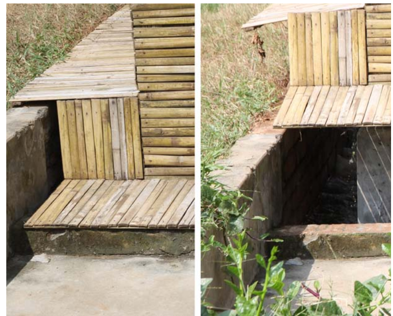
8.168. Ferrocement foundation dwelling on ground (left) and buoyant on water (right)
