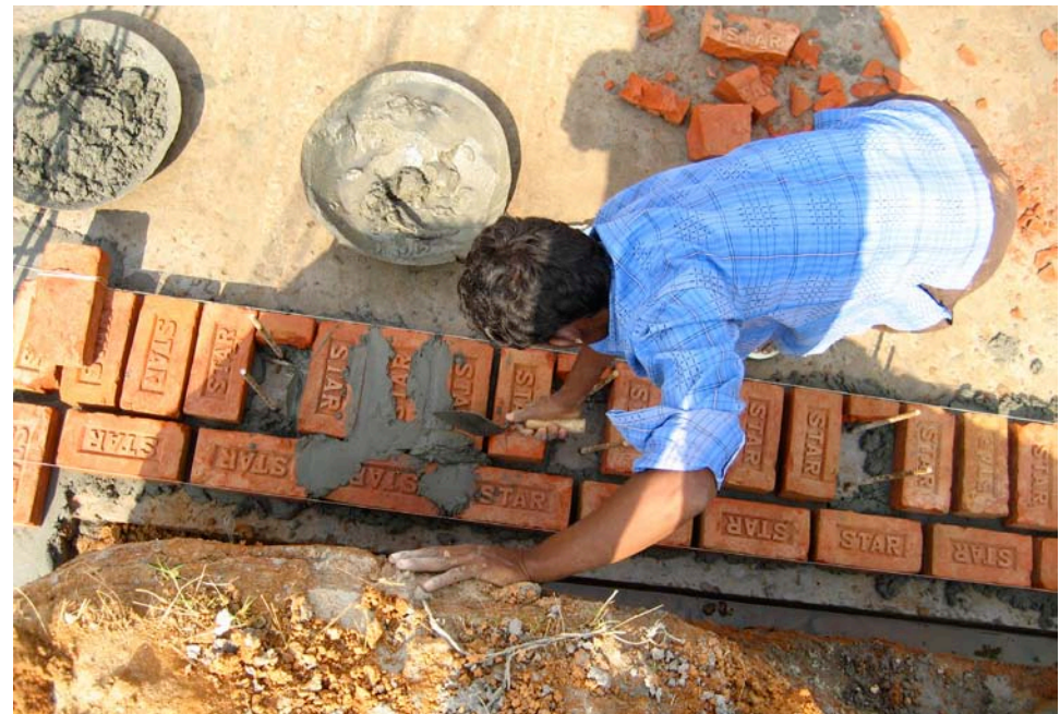
8.28. 15” perimeter wall with dowels for added strength
