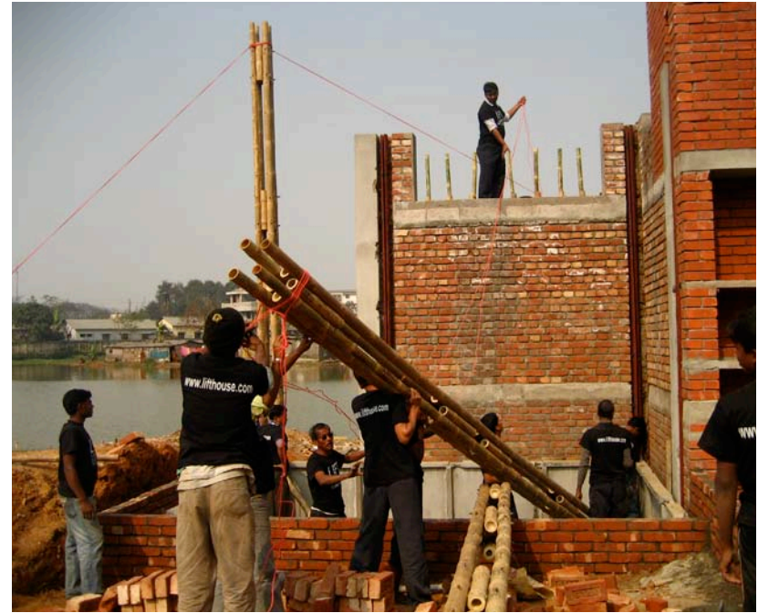
8.102. Columns pulled in place on ferrocement foundation
