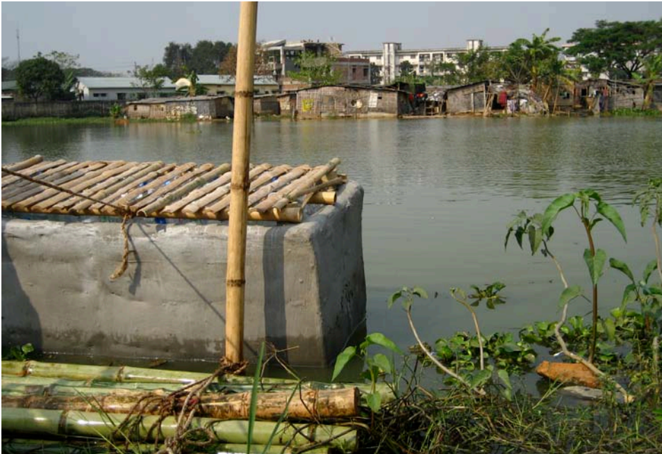
8.41. Bamboo floor built for volunteers to be able to sit on model
