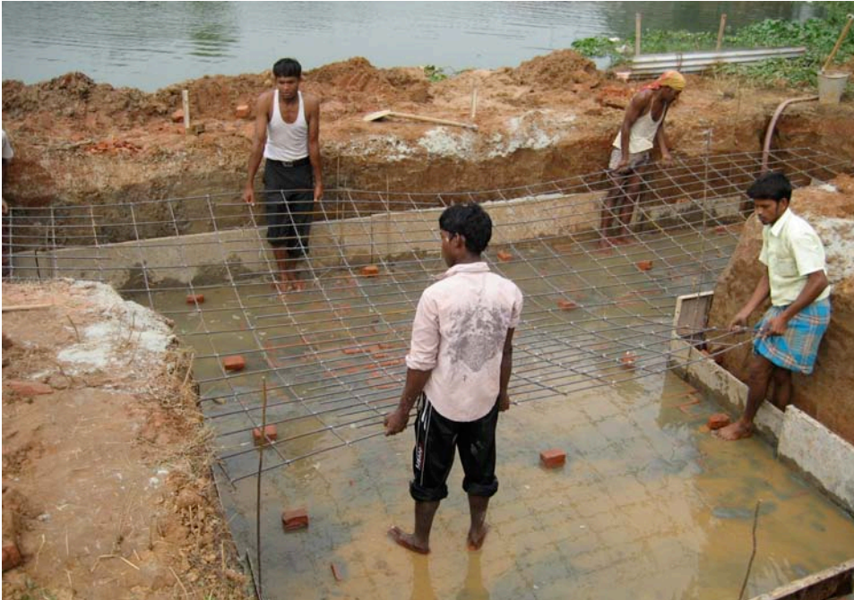
8.24. Reinforcement laid for concrete slab
