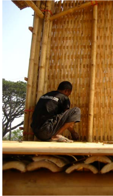
8.118. Installment of walls
