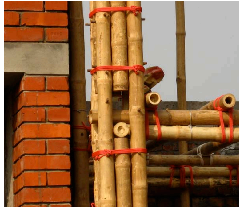
8.84. Detail of column and beam connection
