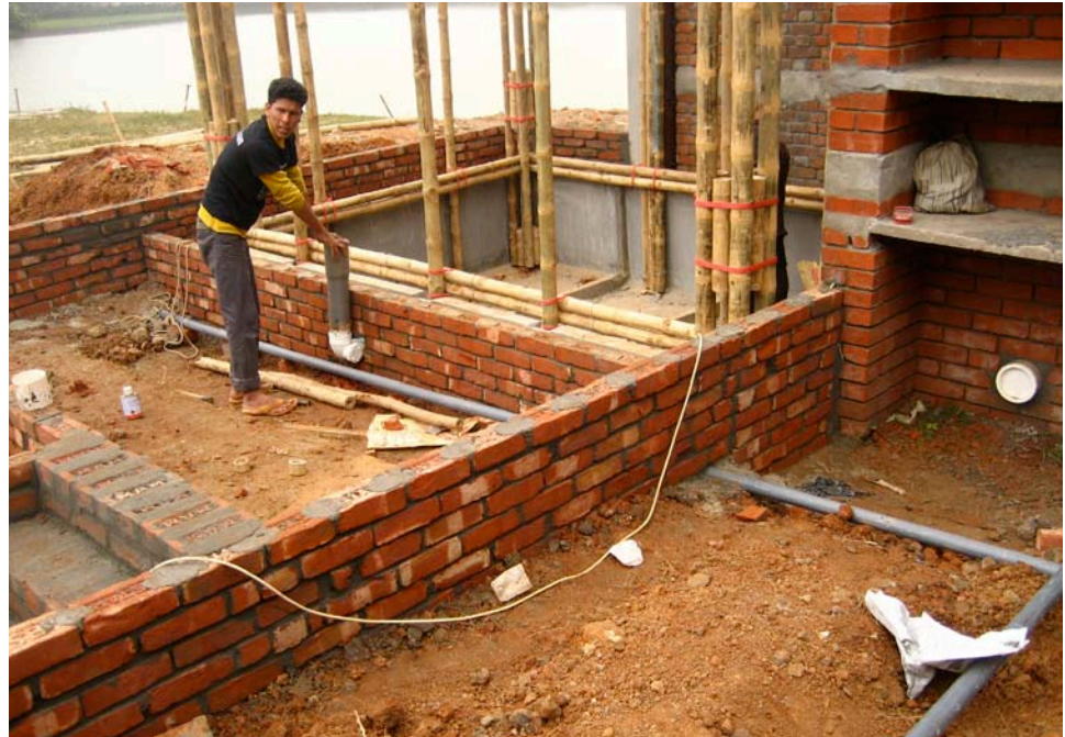
8.115. Plumbing laid for drainage
