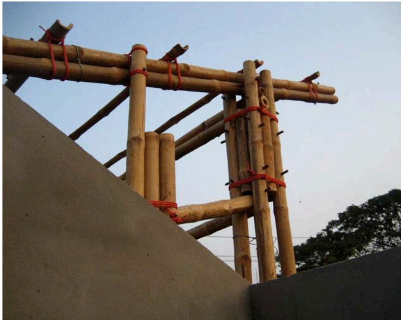
8.101. Bamboo frame showing connections
