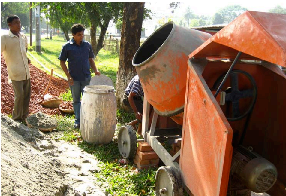
8.25. HBRI's concrete mixture used to pour floor slab of the service spine
