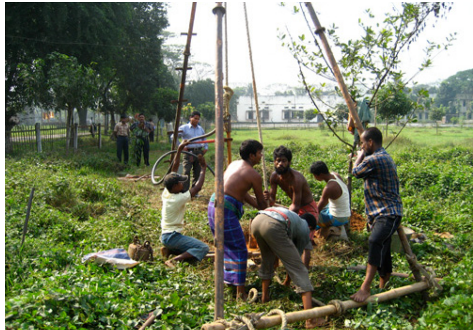
8.0. Soil test conducted on site
