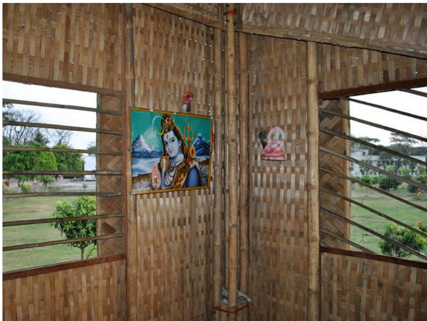
8.166. Interior wall used to hang personal items
