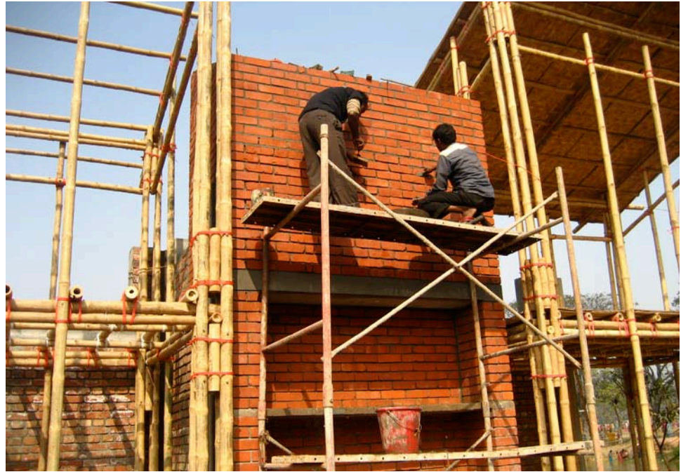
8.108. Grout lines cleaned by workers
