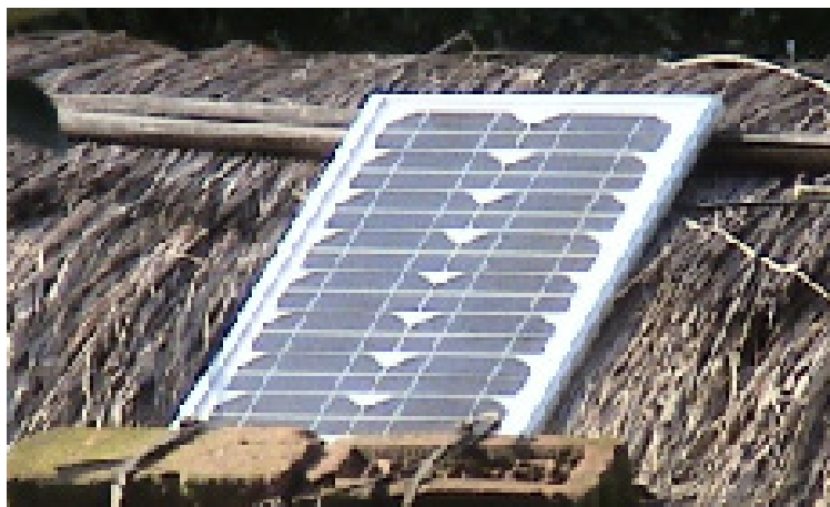
7.8. Photovoltaic panel installed on a thatched roof in rural Bangladesh
