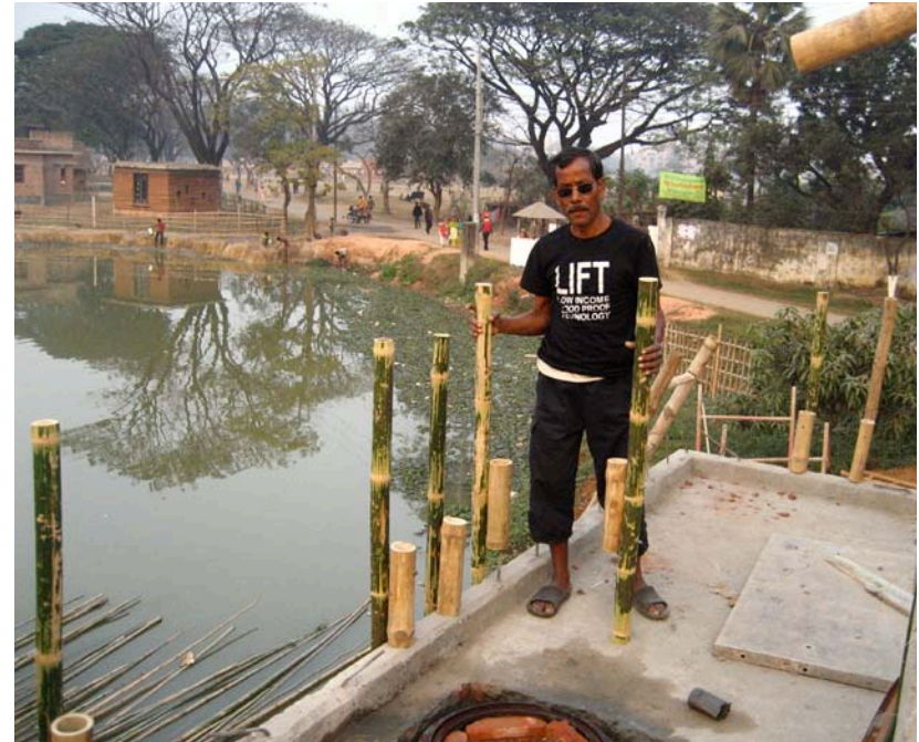
8.98. Installment of bamboo railings
