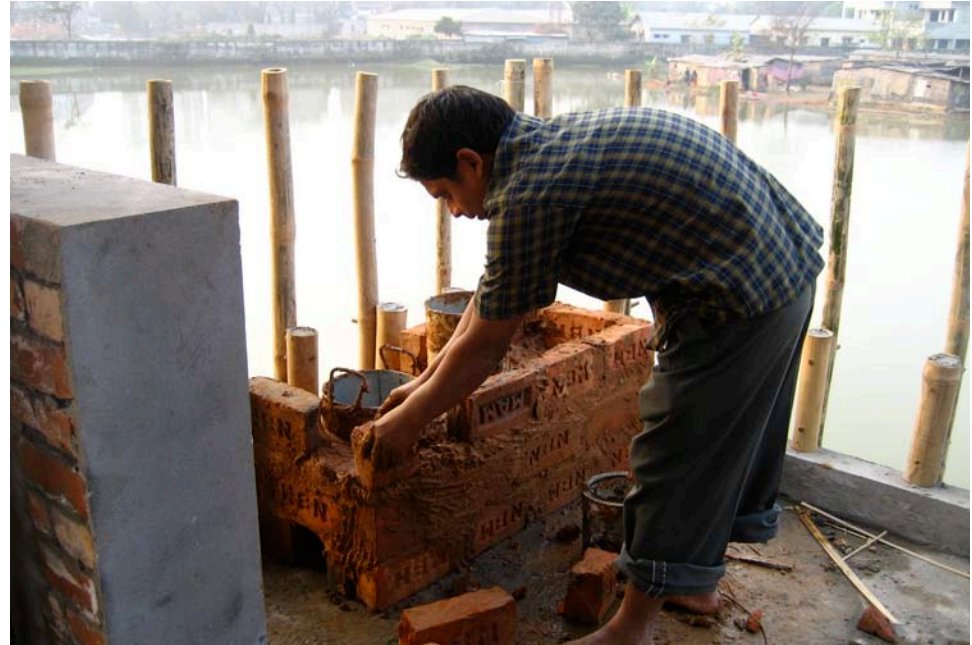
8.128. Installation of Grameen Shakti improved stove
