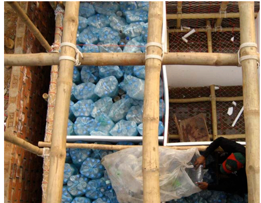
8.107. Used water bottles inserted into foundation
