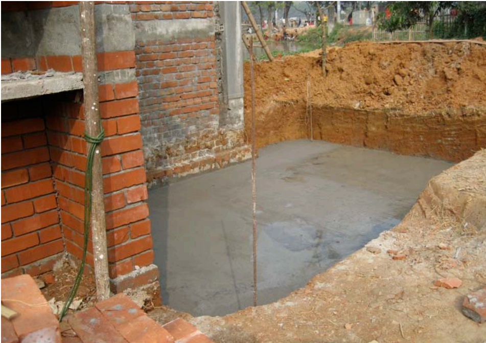
8.57. Layer of concrete on brick soiling on the bottom of the water bottle foundation dwelling holding tank
