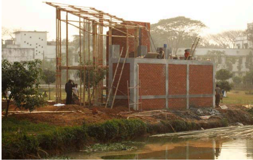
8.104. View of LIFT house across the pond
