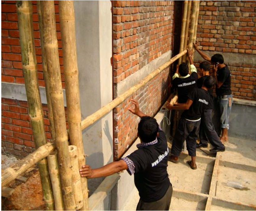
8.100. Beam placement in ferrocement foundation dwelling
