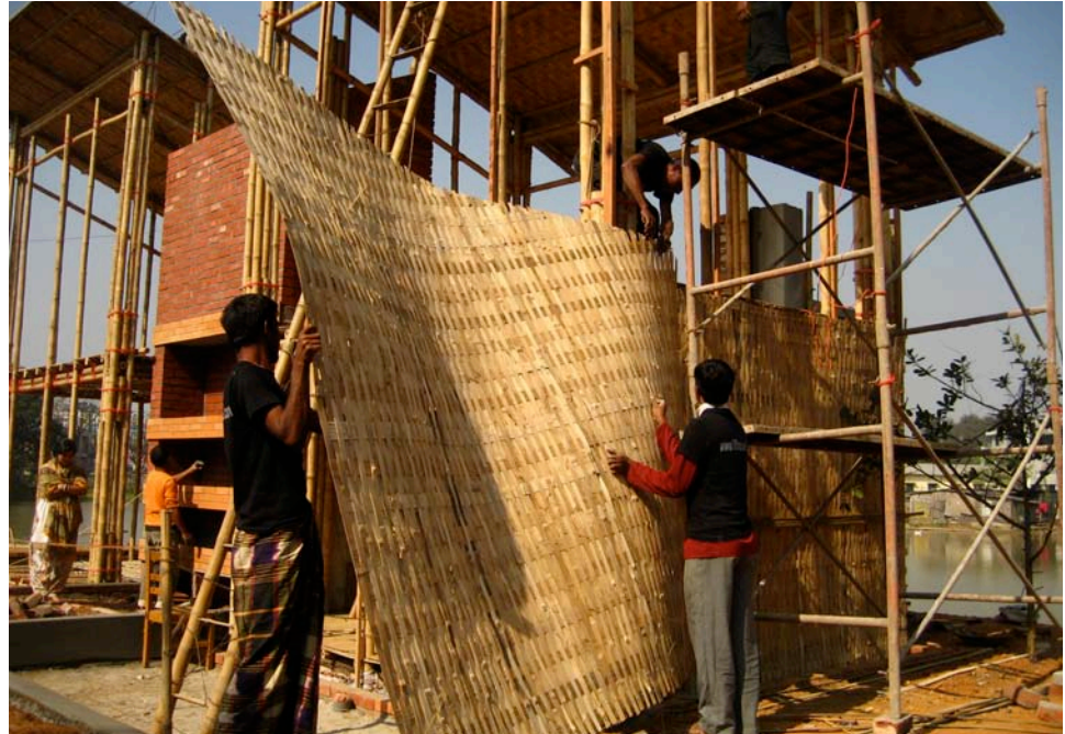
8.116. Installation of interior bamboo wall
