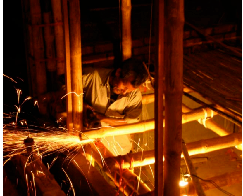
8.120. Installment of floor joists in ferrocement foundation
