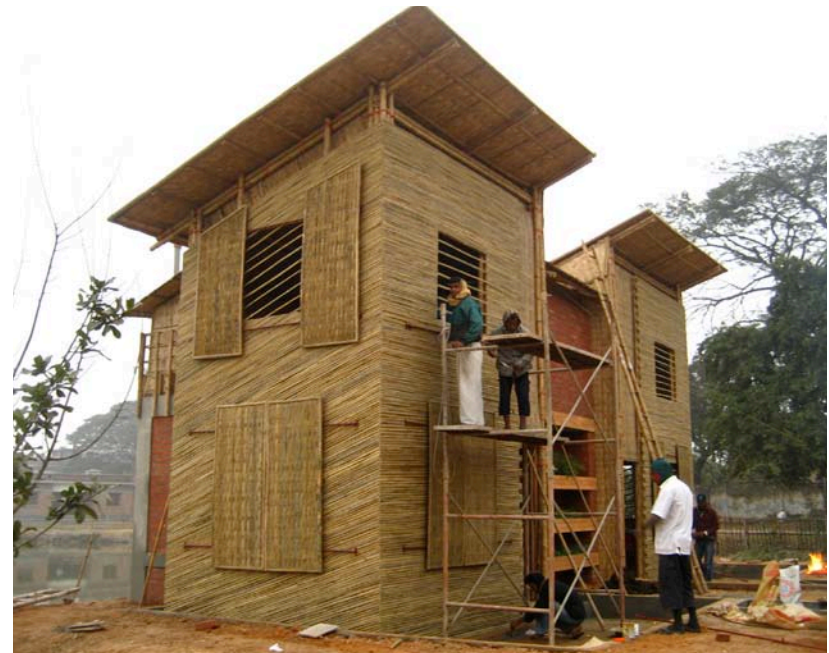
8.148. Installation of sliding shutters
