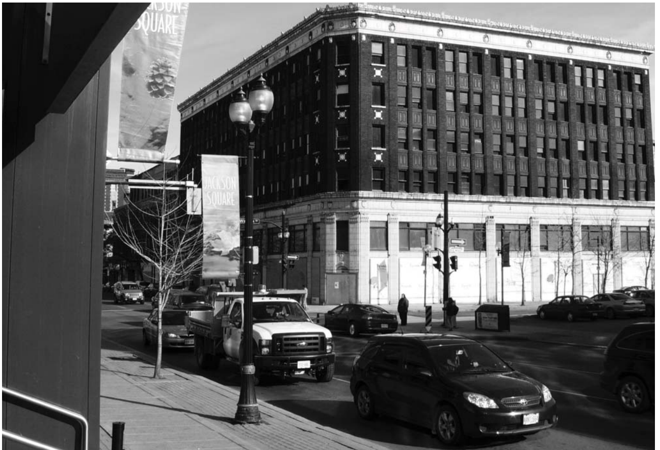
Figure 2.65 NE Corner James Street North and King William Street
