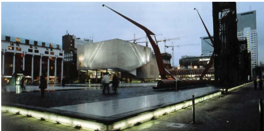
Figure 1.14 Schouwburgplein in Rotterdam, The Netherlands. Unique, interactive, and sculptural lighting features provide interest and safety.
