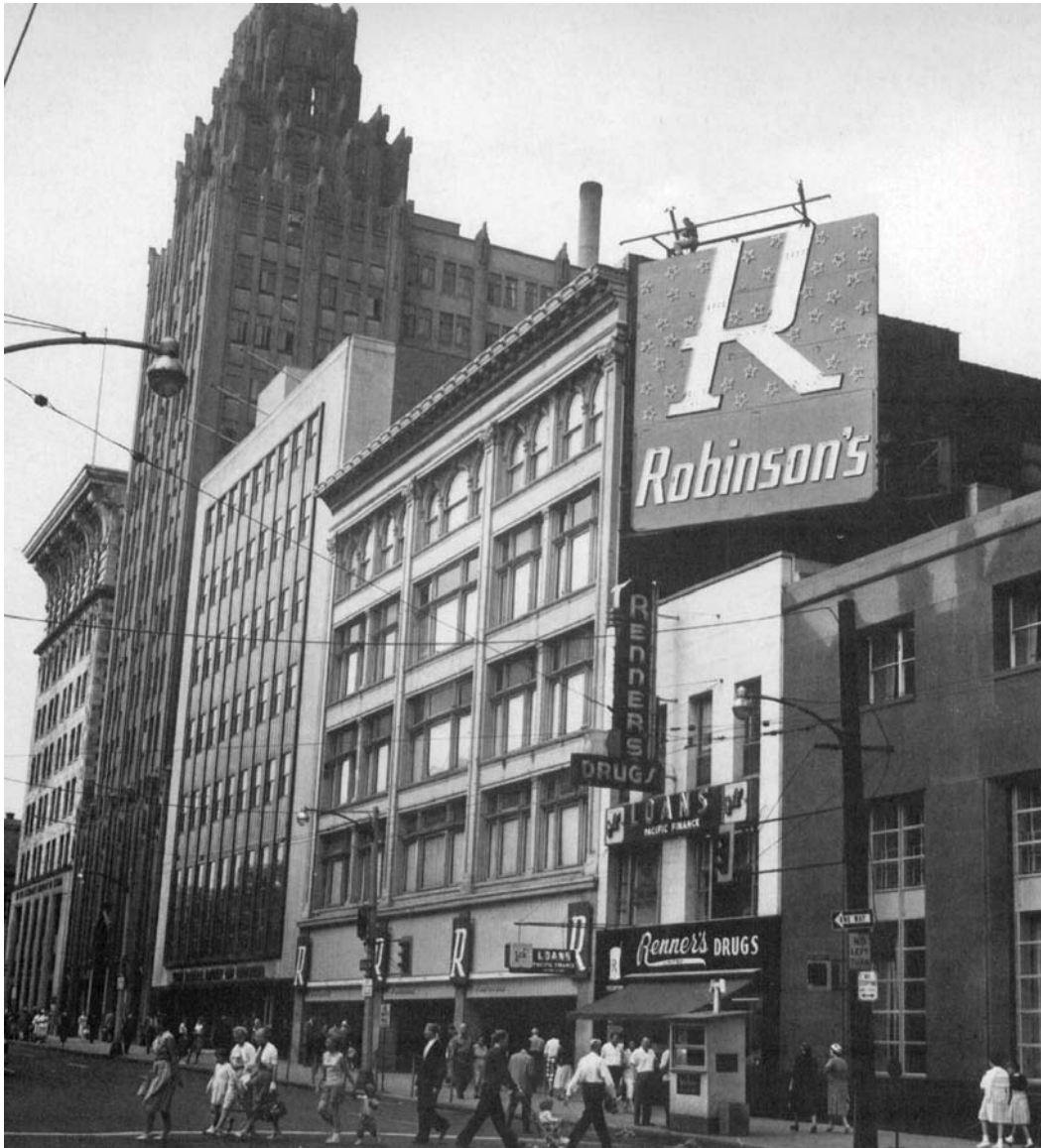
Figure 2.30 W Side of James Street South Between King Street and Main Street
