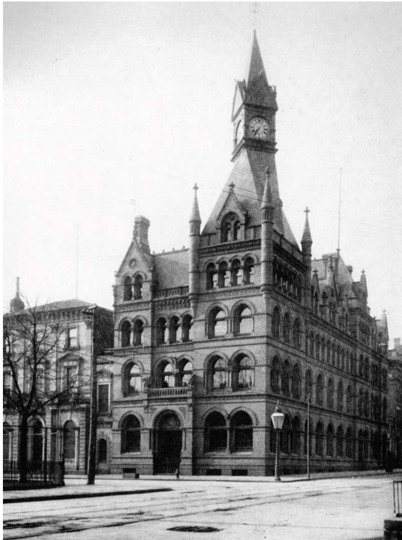
Figure 2.32 SE Corner James Street South and King Street
