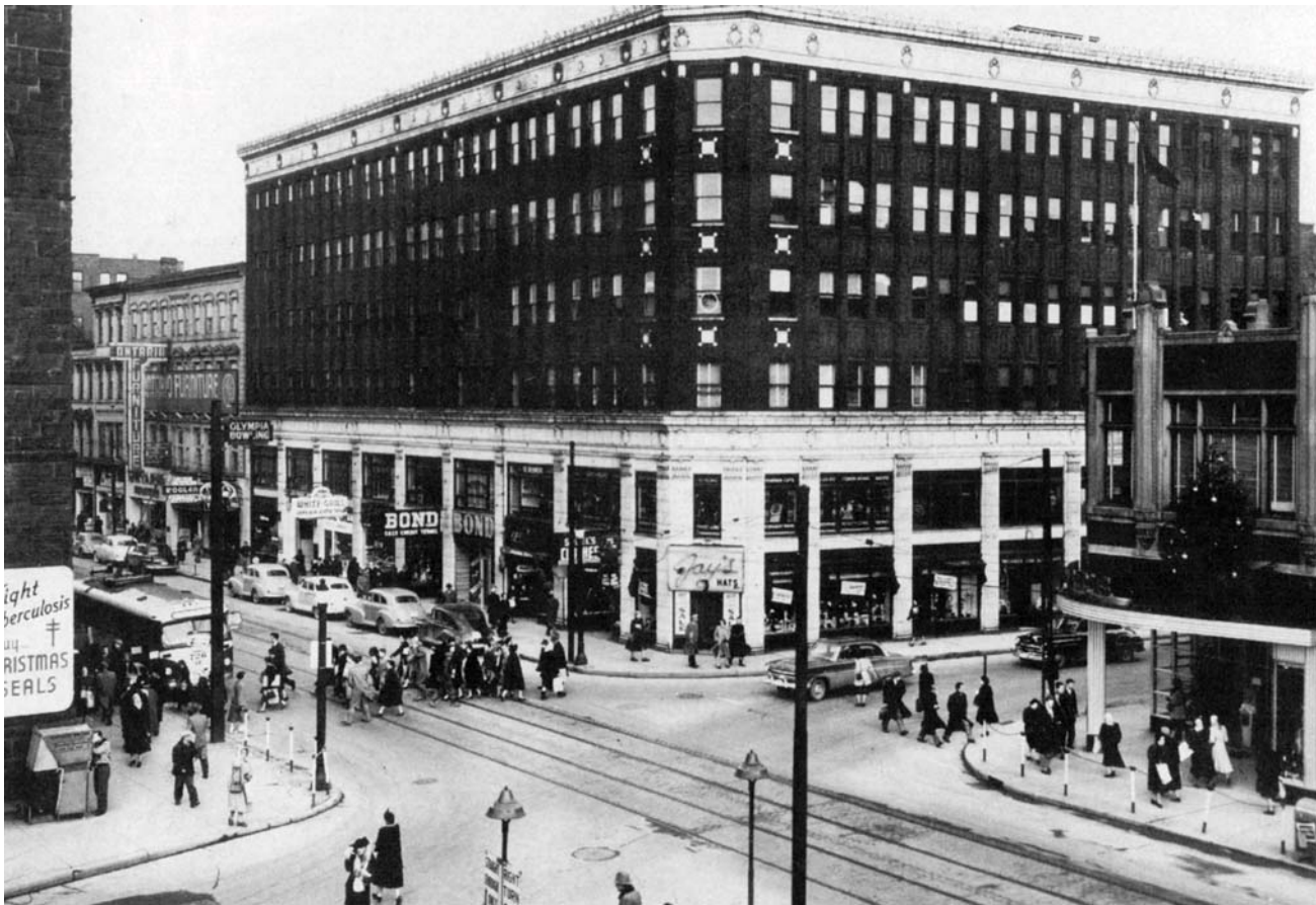
Figure 2.64 NE Corner James Street North and King William Street
