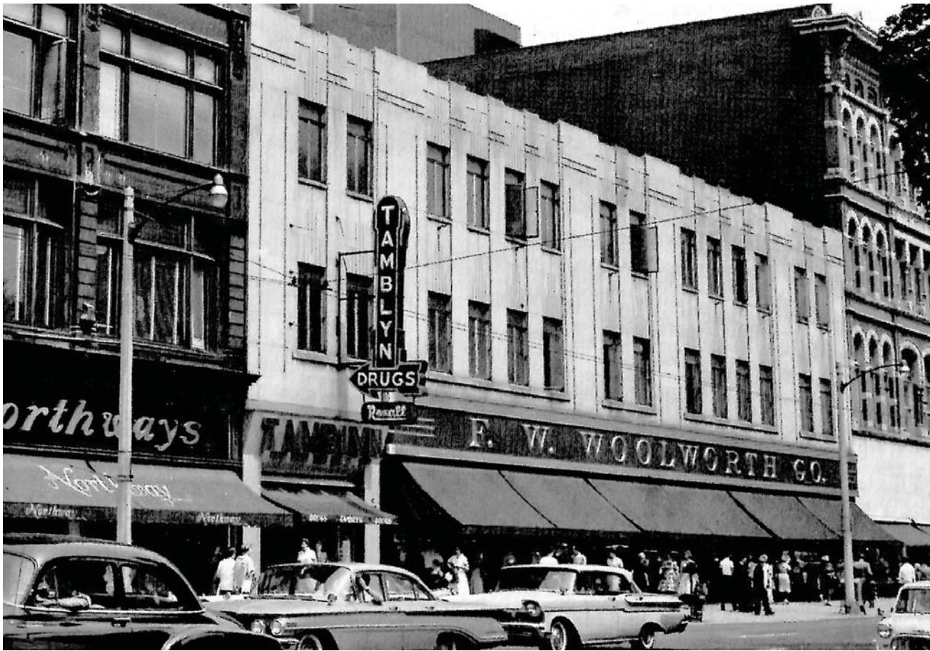
Figure 2.36 N Side of King Street East between James and Hughson
