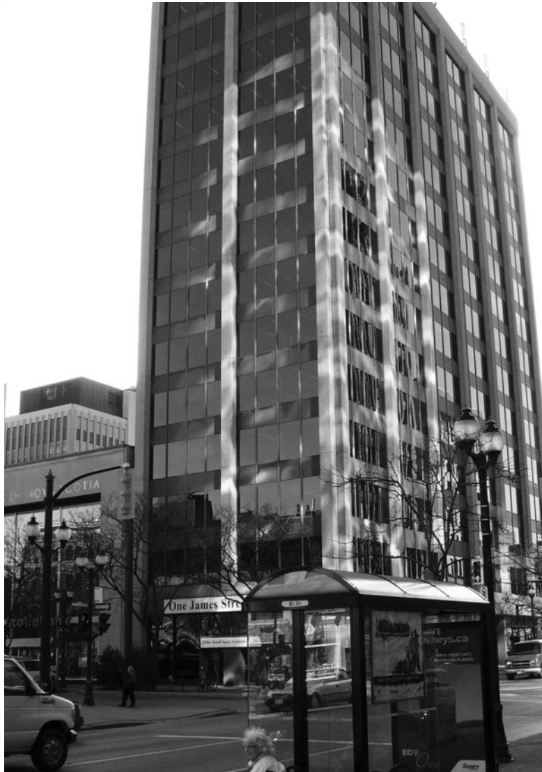
Figure 2.33 SE Corner James Street South and King Street
