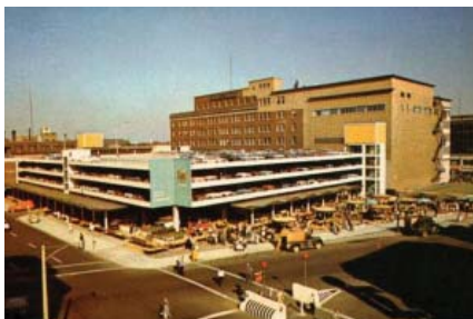
Figure 2.17 Market Square Carpark, 1961
