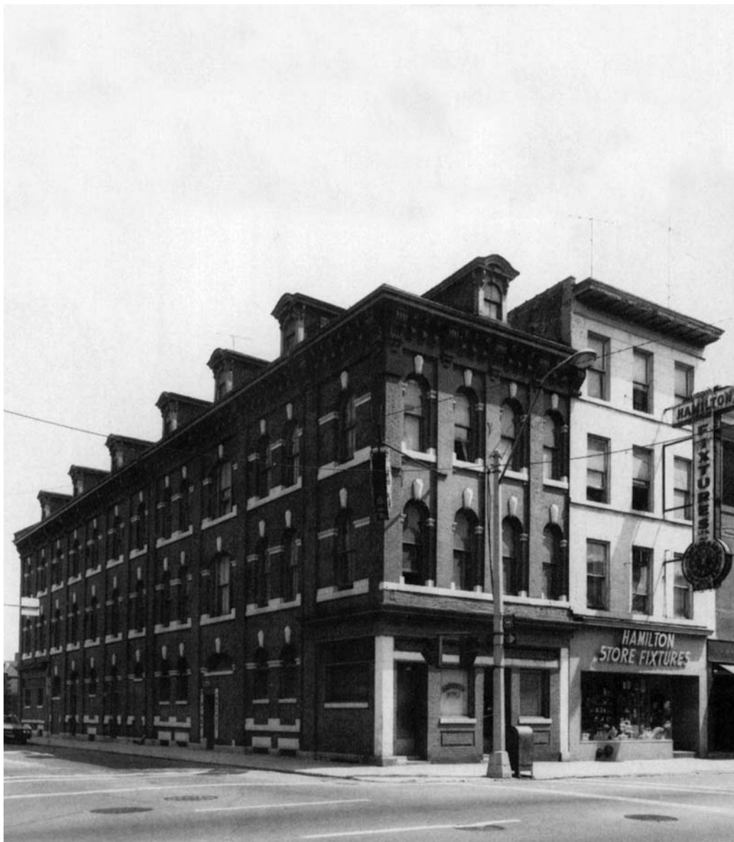
Figure 2.52 NE Corner King Street West and Park Street North
