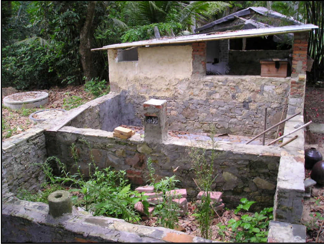
Figure 4.9: An Abandoned Anaerobic Digester in Maoshan Village (Wenchang)
