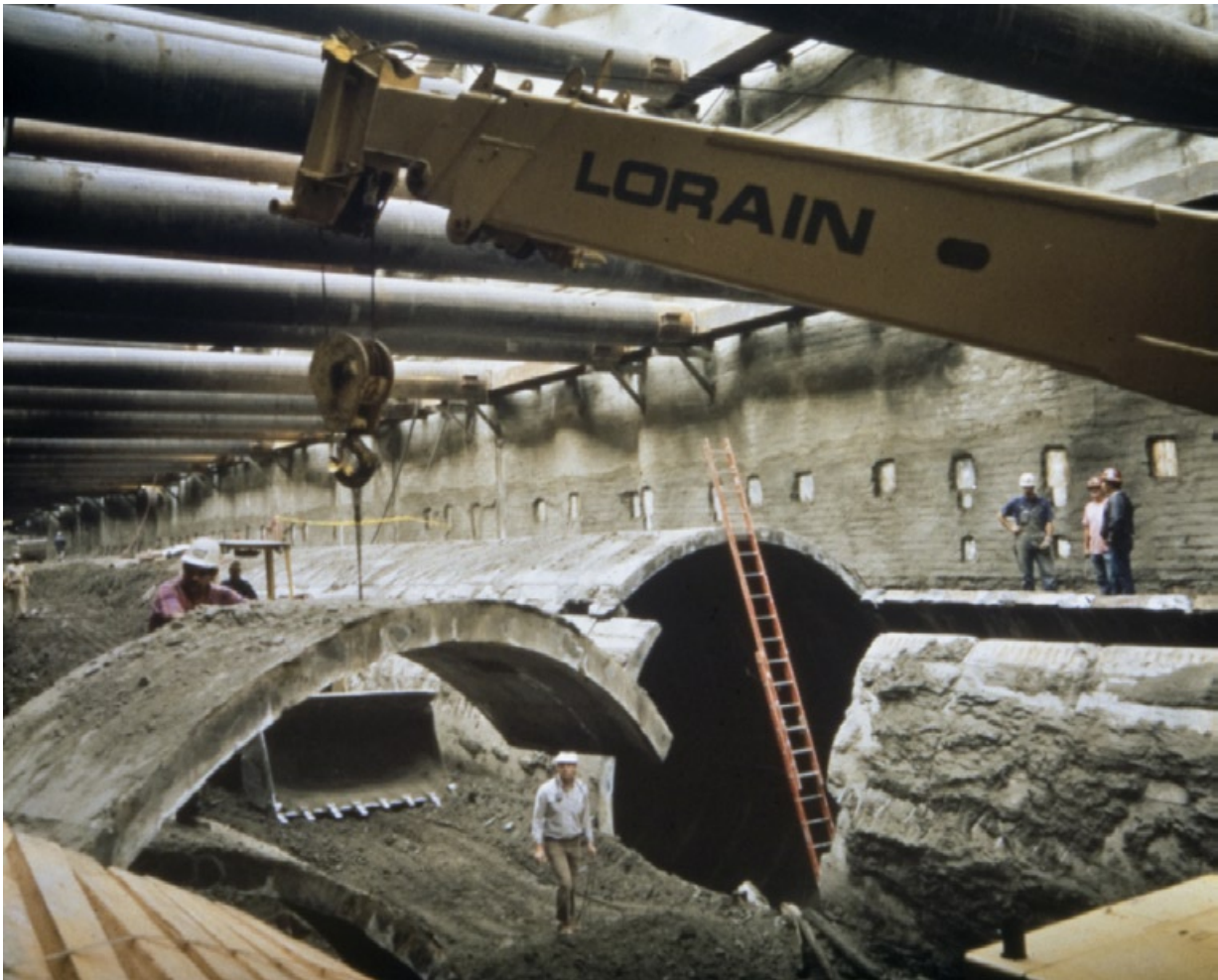
Fig 1.17 Metro Red Line Tunnel During Construction
