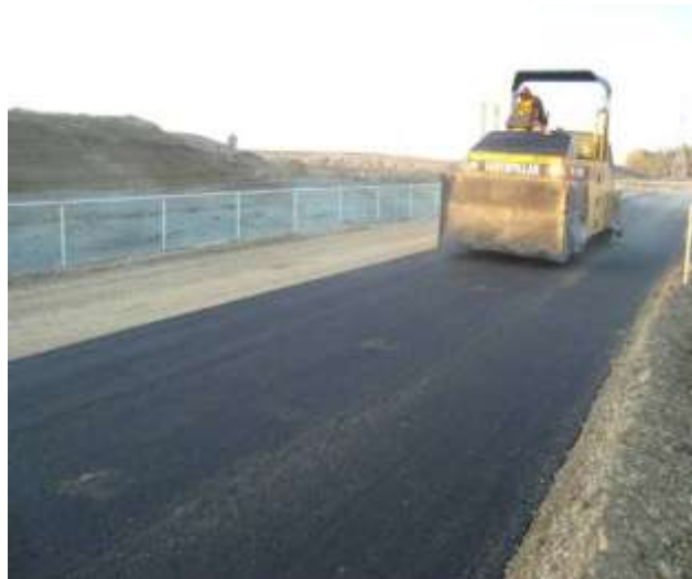
Figure 5-6 : Compaction of Asphalt with Pneumatic Tire Compactor at Station 0+1100
