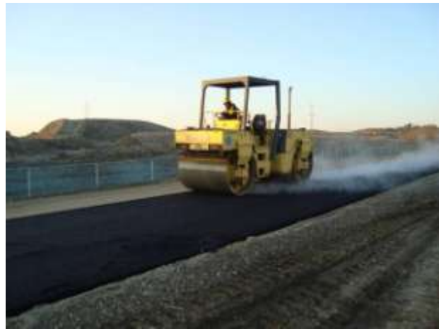
Figure 5-5 : Compaction of the Asphalt with Steel Wheel Roller at Station 0+1100
