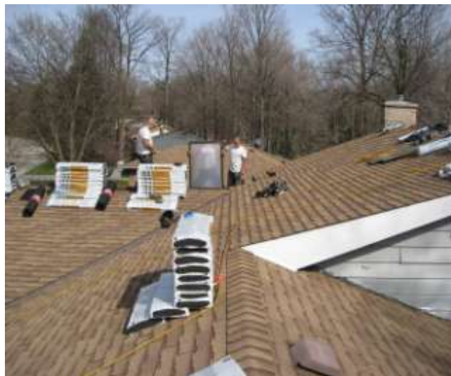
Figure 2-1 : Asphalt Shingles on a Residential Roof
