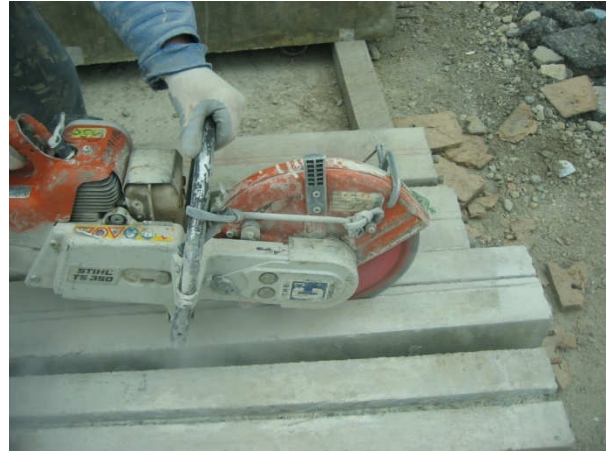
b-Grooves being cut in the concrete
