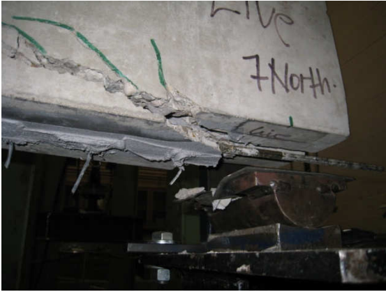
a-Bottom view showing the CFRP separation from the beam in region 1
