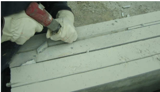
c-Chipping concrete pieces from the groove
