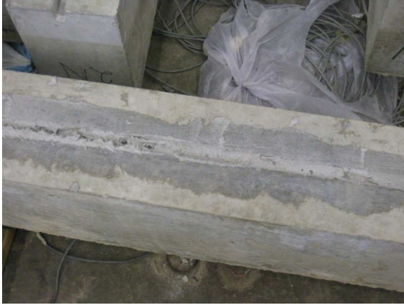
a- Groove half filled with epoxy
