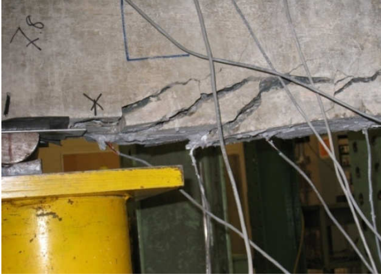
a-Beam after failure
