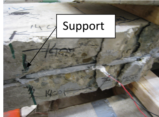
b-Soffit of the beam after failure
