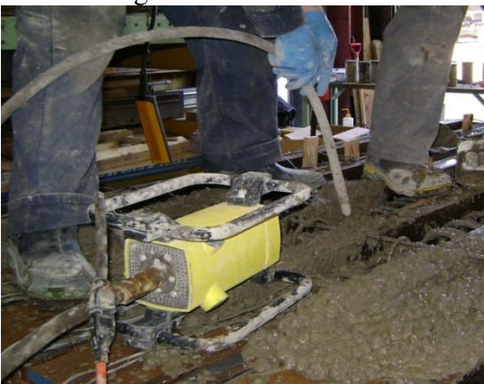
c- Concrete vibration
