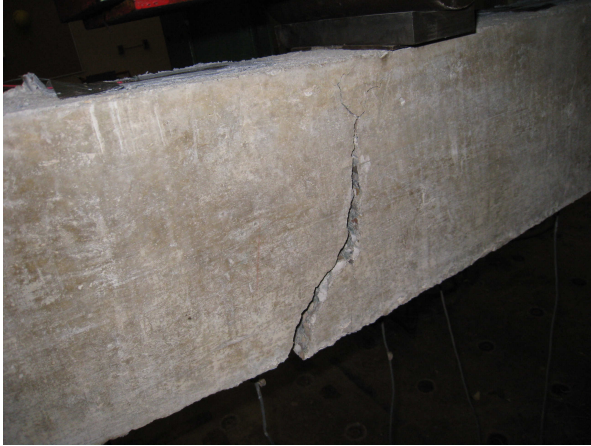
a-Crack in the shear span
