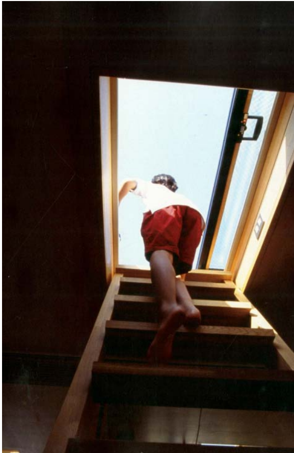
Fig.5.19- skylight roof access
