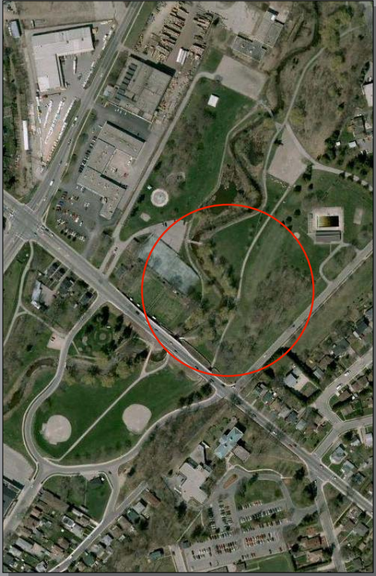
Fig.7.42- aerial view - Soper Park
