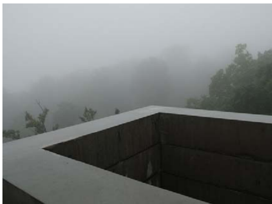
Fig.7.4- Pavilion at Kivik Art Center - tower
