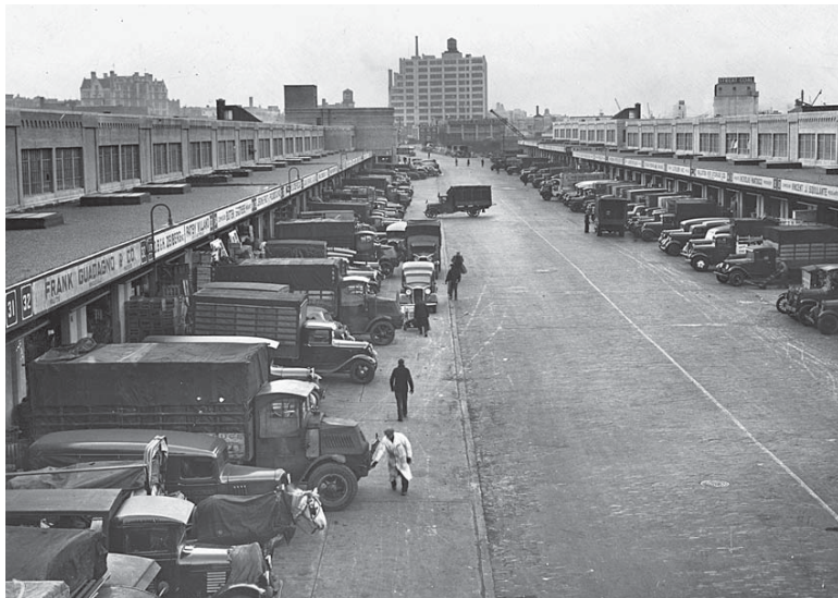
1.03 Newer wholesale distribution facilities were designed with wide traffic lanes and individual docks to accommodate the increased number of truck deliveries. This system has expanded further to accommodate even larger trucks with semitrailers.
