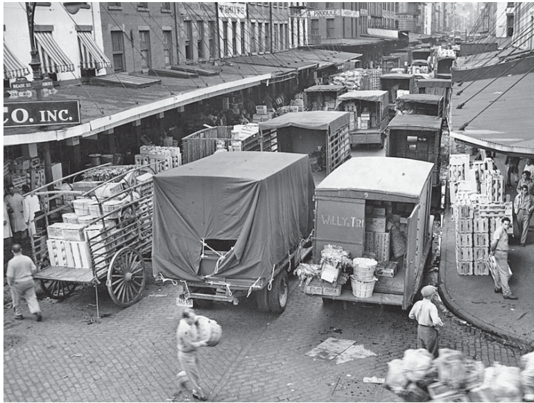
1.02 As transportation evolved, deliveries became increasingly difficult. Trucks created massive amounts of congestion while attempting to squeeze through narrow streets designed for pedestrians and carts.
