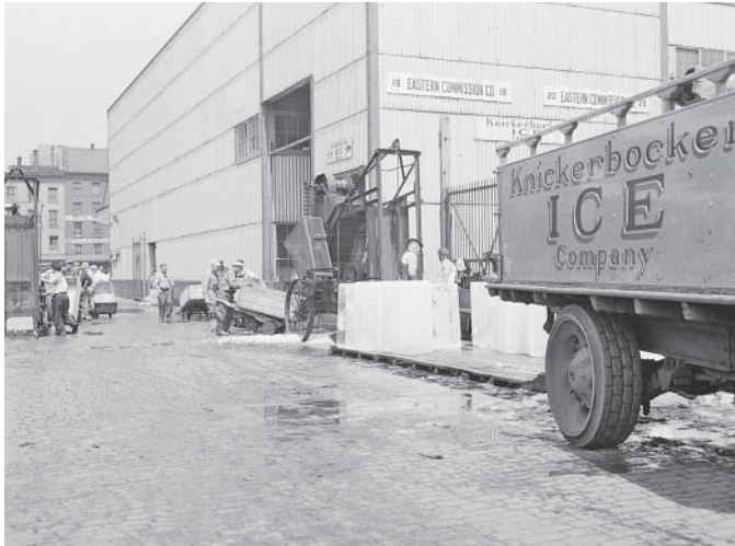
1.06 Up until the end of the nineteenth century, refrigeration was relatively primitive. Methods of cooling were basically derived from man-made ice blocks and were used almost solely for keeping seafood and dairy products. (Anderson 1953, 31)
