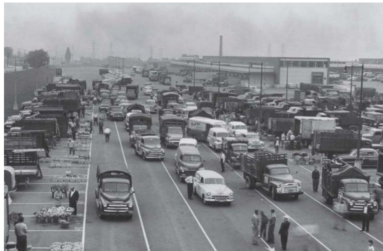
1.11 The Farmers' Market area in 1959, prior to construction of the parking deck.
