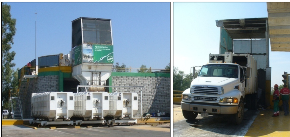
Figure 4.8: The north compaction and transfer station in Aguascalientes.
