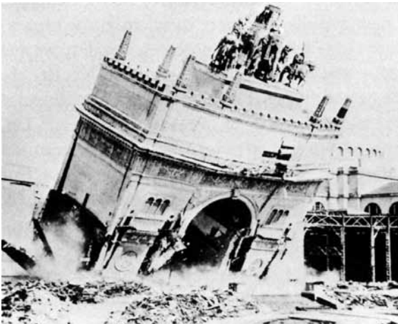
Demolition of the Court of the Universe, 1914
