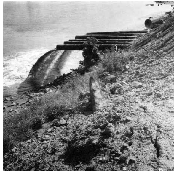
The Fountain Monument: Side View
