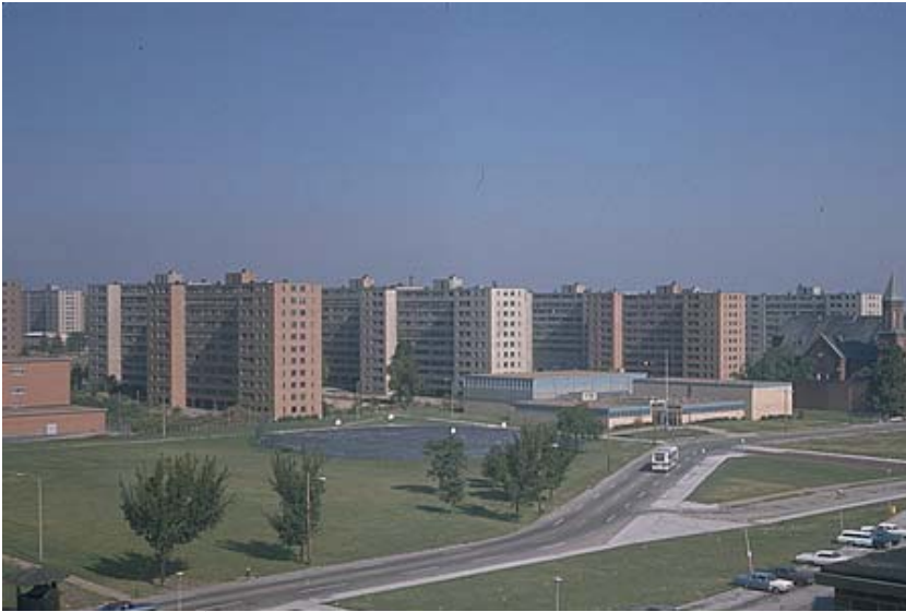
Fig. 2.11 Pruitt-Igoe housing project - St. Louis, Missouri
