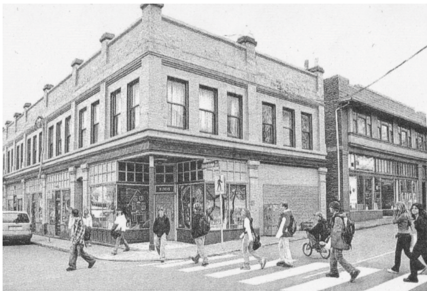
Fig. 3.12 Cornerstone Building before renovations
