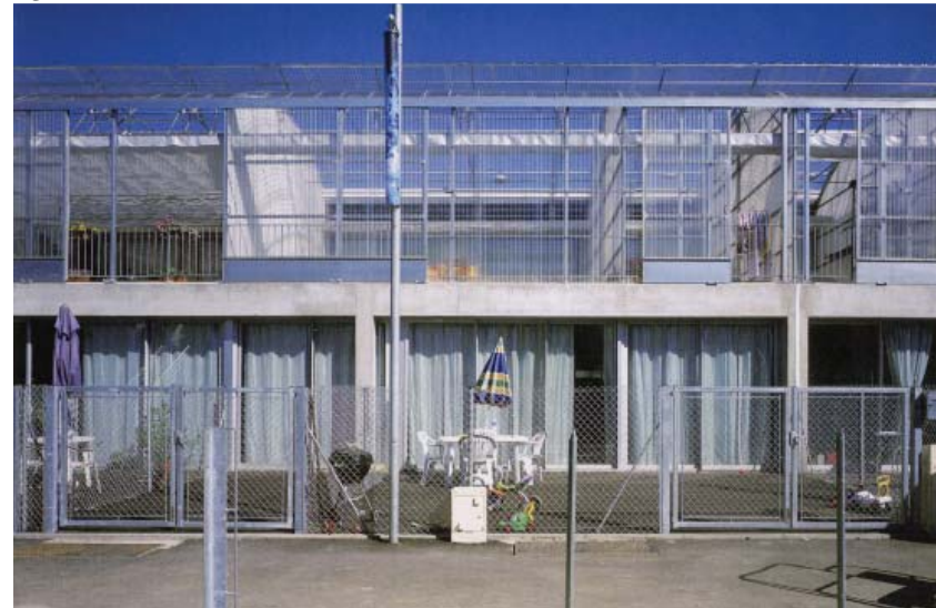
Fig. 3.4 Lacaton & Vassal front facade
