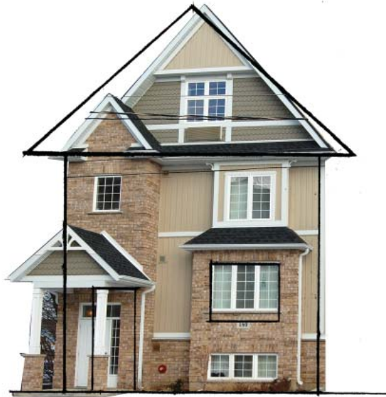
Fig. 3.40 160 Ontario Street front facade
