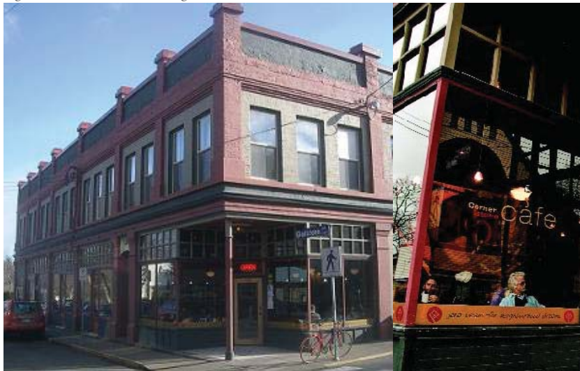
Fig. 3.13 Cornerstone Building after renovations
