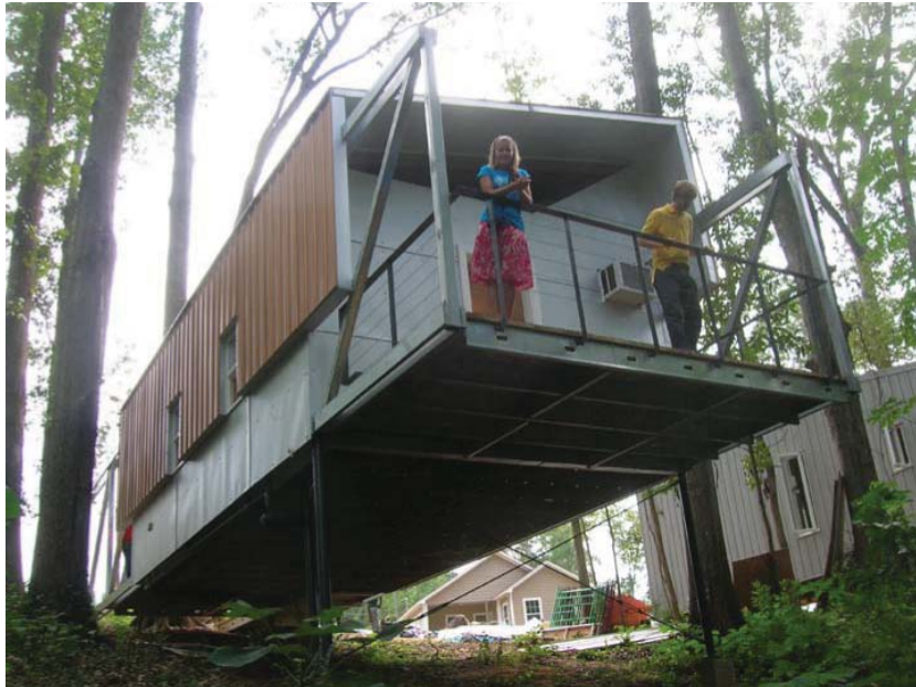
Fig. 3.45 20K Bridge House back porch
