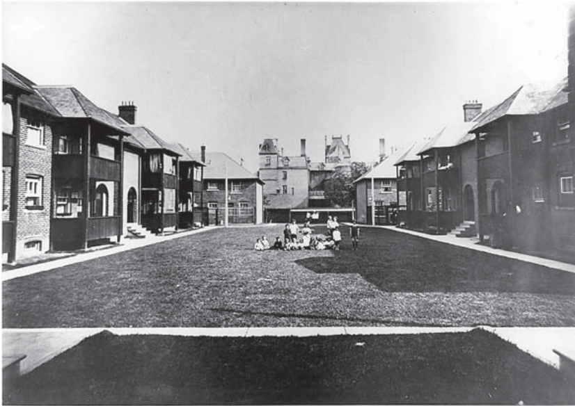
Bain Ave. apartments (first urban renewal?) 1920?
