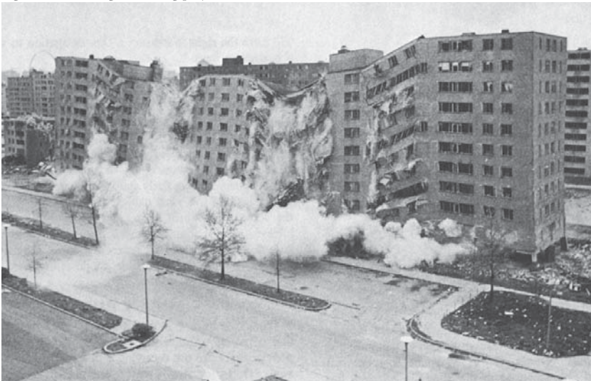
Fig. 2.12 Pruitt-Igoe housing project - demolition 1970s
