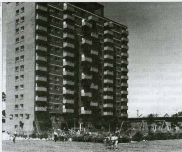
The Jeanne Mance public housing project in Montreal was typical of the early 1950s: large scale "slum" clearance, followed by the erection of a structure which bore little relationship to its surroundings, and lots of open green space.
