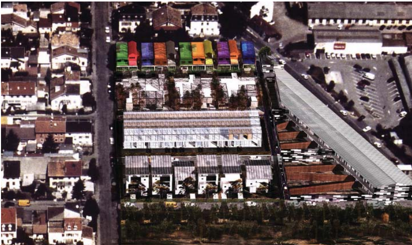
Fig. 3.41 Mulhouse Social Housing aerial view
