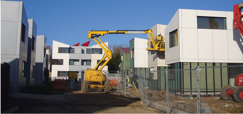
Fig. 3.48 Oxley Woods under construction
