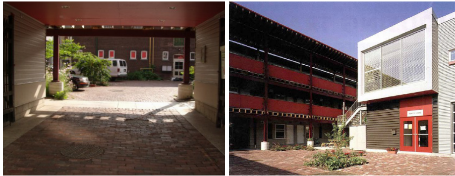
3.13 (Right) The courtyard is open to the main facade and creates a link between the Centre and the street.
