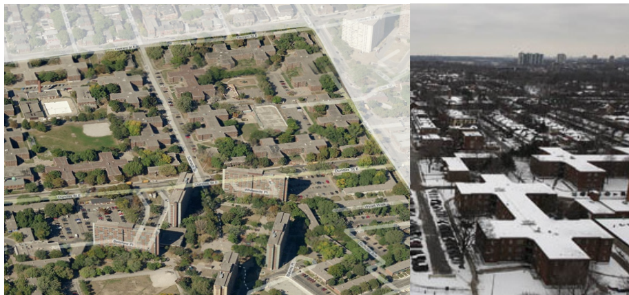
3.19 The existing, uniform, and physically isolated development of Regent Park
