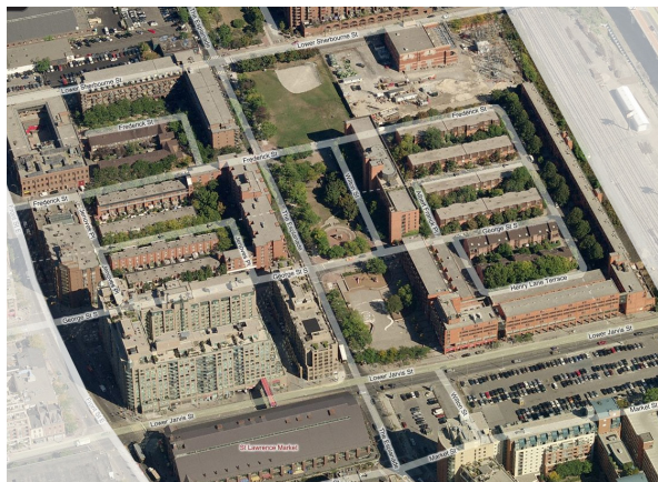
3.21 (Right) St. Lawrence Market is one of the many integrated amenities which are blended into development
