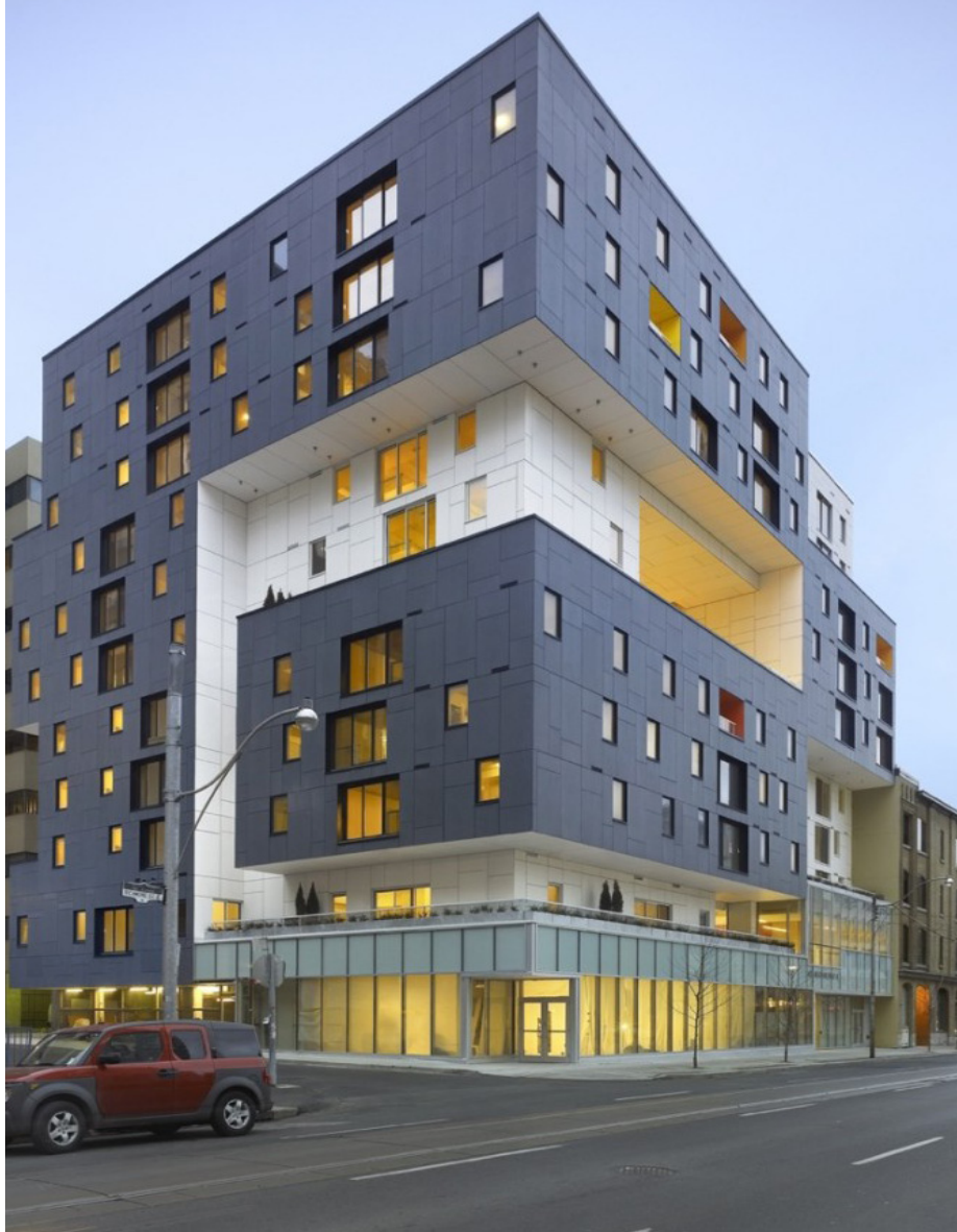
3.15 View of 60 Richmond, exemplifying common terraces and transparent facade. (The interior of the ground level is under construction at the time of this photograph)
