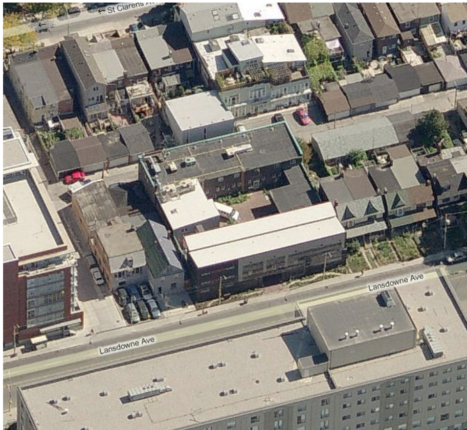
3.10 Aerial Photograph of the Christie Ossington Neighbourhood Centre. The centre is tightly inserted into the existing fabric.
