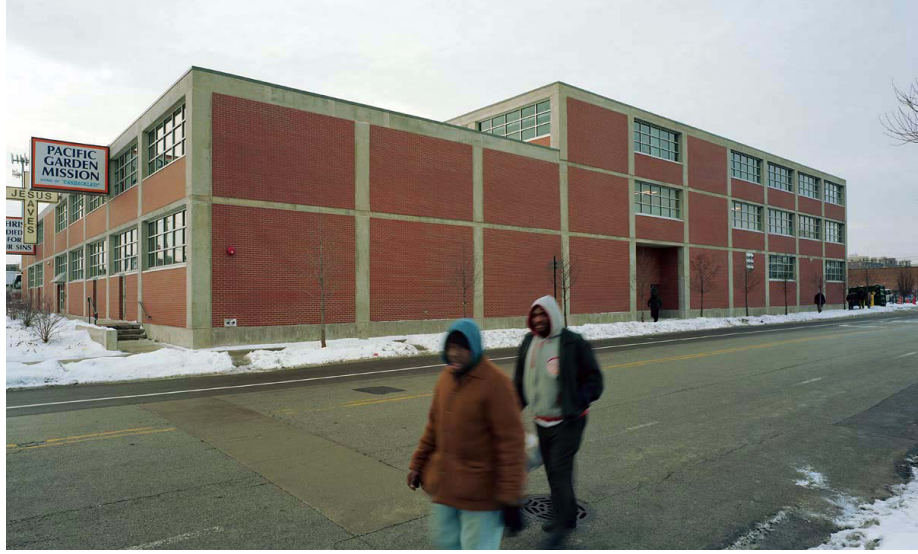
3.5 Exterior Facade of the PGM
