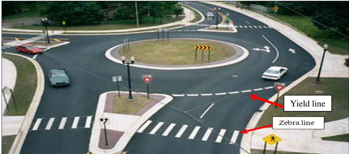
Figure 2: Characteristics of modern roundabout (Three-leg Multi-Lane Roundabout in East Lansing, Michigan, 2011)
