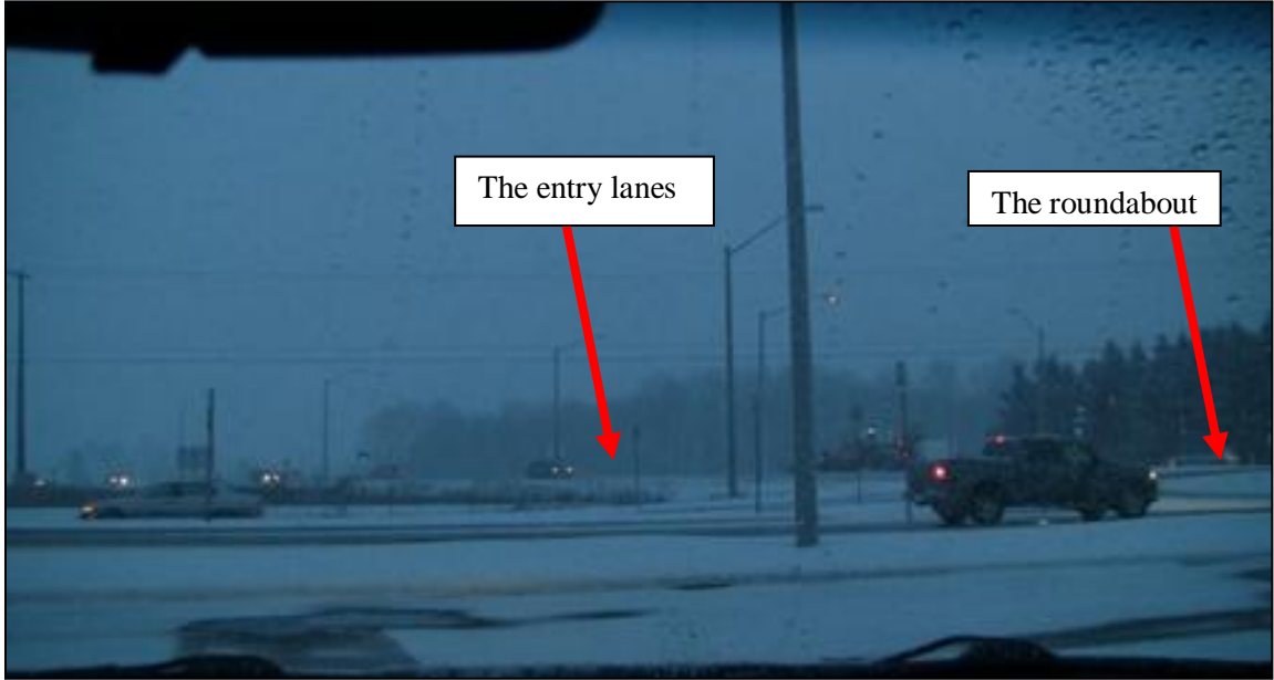
Figure 82: Roundabout in the Sawmill Rd. / Arthur St. S (HW 85) as video recorded
