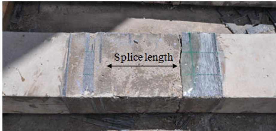
b) Elevation view after removing the CFRP wrap
