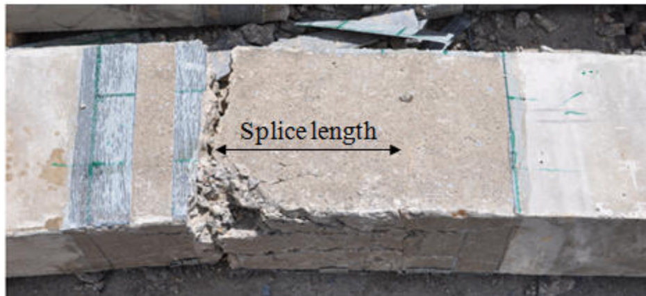
b) Elevation view after removing the CFRP wrap
