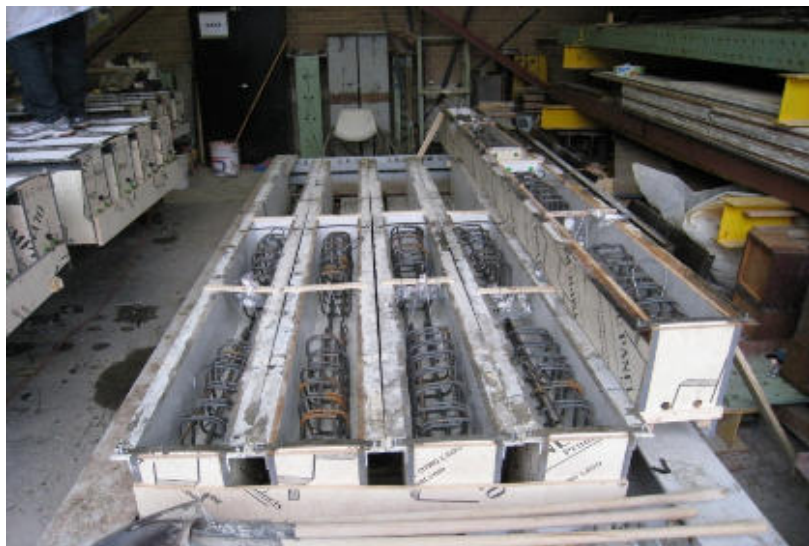
Figure 3-7 Reinforcing steel cages inside the form work
