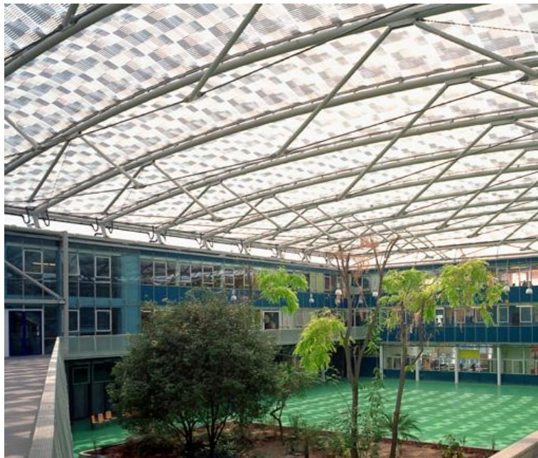
Figure 1.12 - Kingsdale School courtyard, with both chambers of the ETFE cushions inflated (Vector Foiltec, 2011d)
