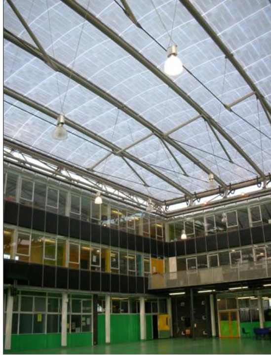
Figure 1.13 - Kingsdale School courtyard, with only one chamber of the ETFE cushions inflated (Vector Foiltec, 2011d)
