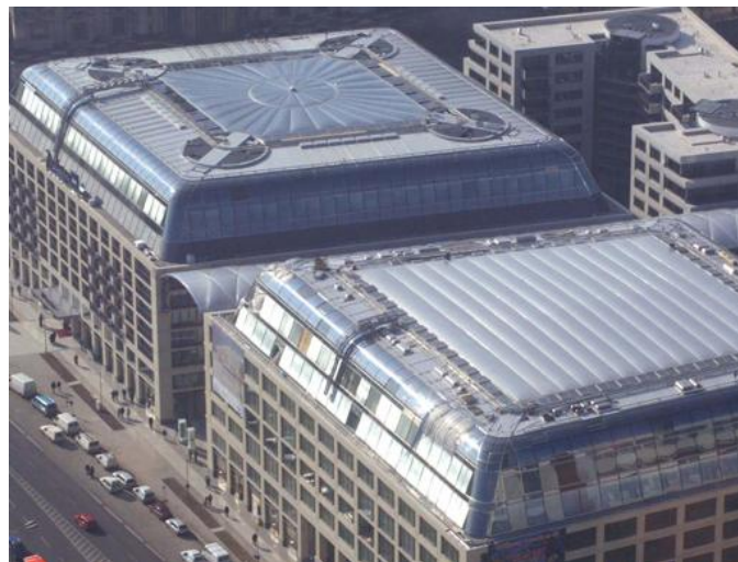
Figure 1.8 - The three ETFE roofs at DomAuarée (Vector Foiltec, 2011a)
