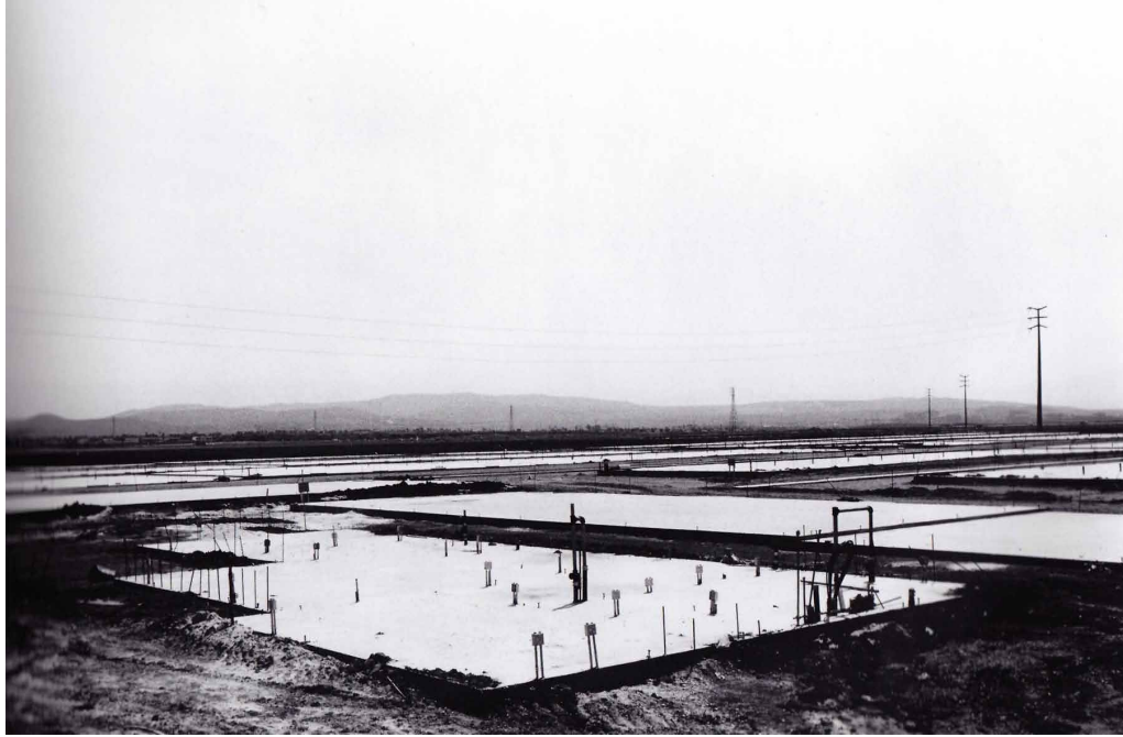
Plate 13. Lewis Baltz, Foundation Construction, Many Warehouses, 2891 Kelvin, Irvine, 1974.
