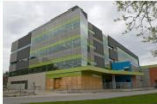
The Construction of the Environment 3 Building, University of Waterloo Main Campus
