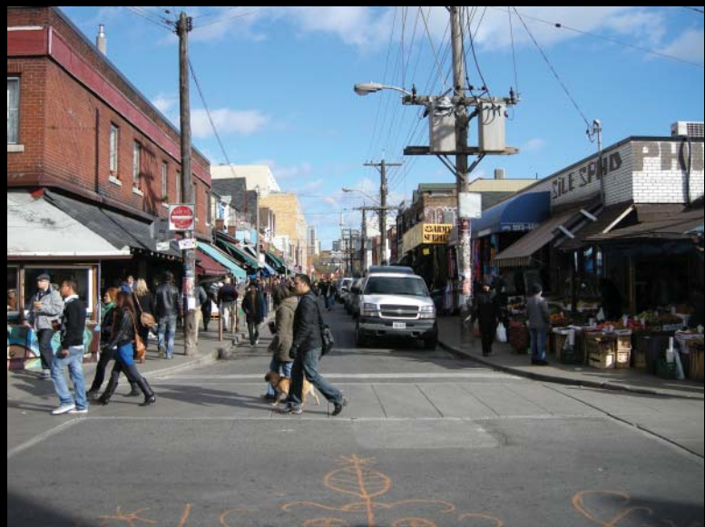
Fig. 5 View of site and existing building (right) looking down Baldwin St..
