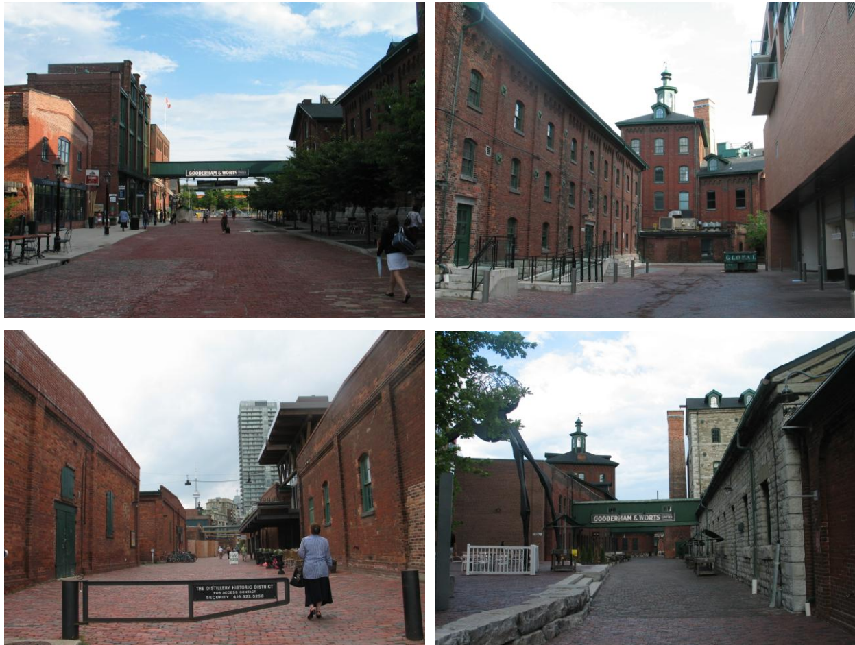
Exhibit 6.16: Photos of the Gooderham & Worts Project (August 10, 2009)
