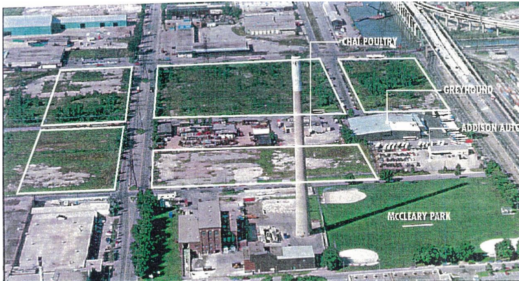
Exhibit 7.2: Aerial Photo of the Project Site for PCD (TEDCO, November 1996)
