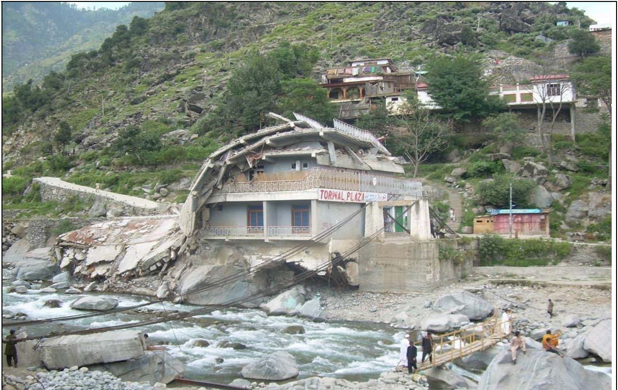
Damaged buildings and suspension bridge after the flood (Source: MinaAllah, 2010a).
