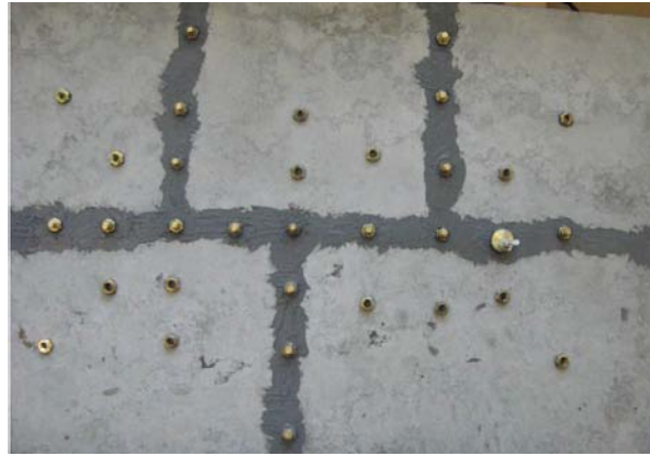
Figure 2.4: Photograph of the Sealed Fractures and the Ports
