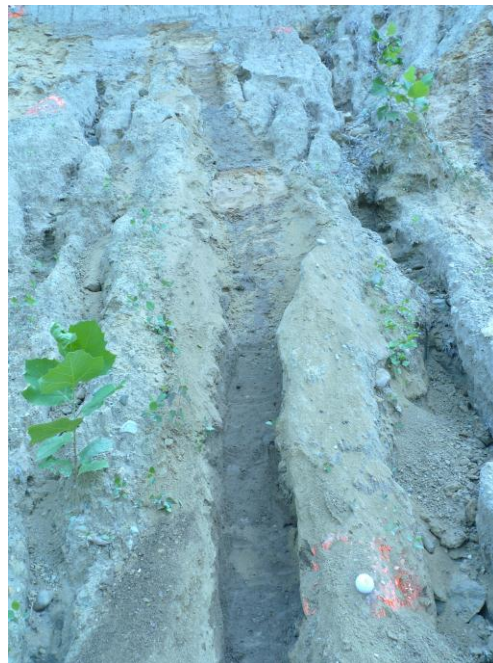
Figure A.9: Trench at the Higginsville section where sediments assigned to the Glasford deglacial unit were described.
