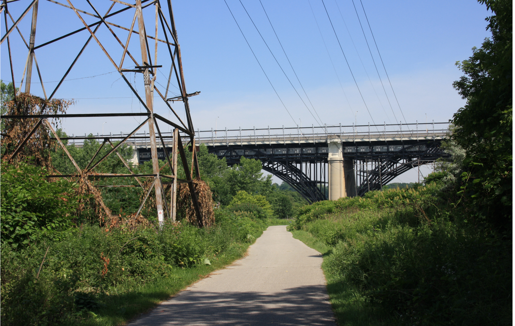
2.12 Subway train passing on the Viaduct
