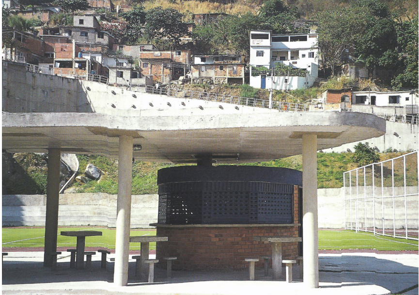
Fig. 2.12 RIGHT - View of community football pavilion in favela in Rio de Janeiro constructed as part of the Favela-Bairro Project.
