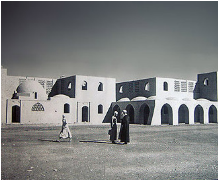
Fig. 2.11 RIGHT - View of street in New Gourna Village, Near Luxor, Egypt, showing the traditional vernacular employed.
