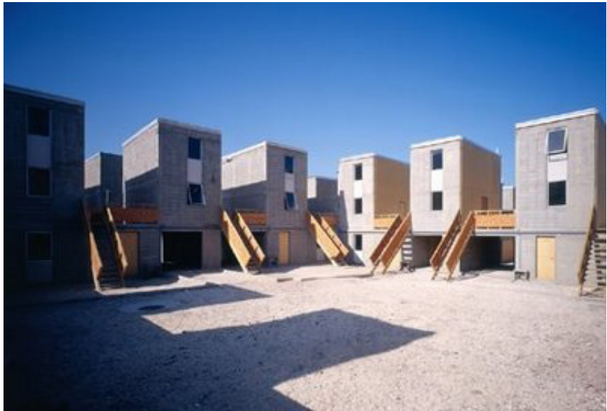
Fig. 2.27 RIGHT - Ground Level View of affordable housing units designed by the firm Elemental, in Chile. The Modular Units are arranged to allow for future expansion between units by residents.
