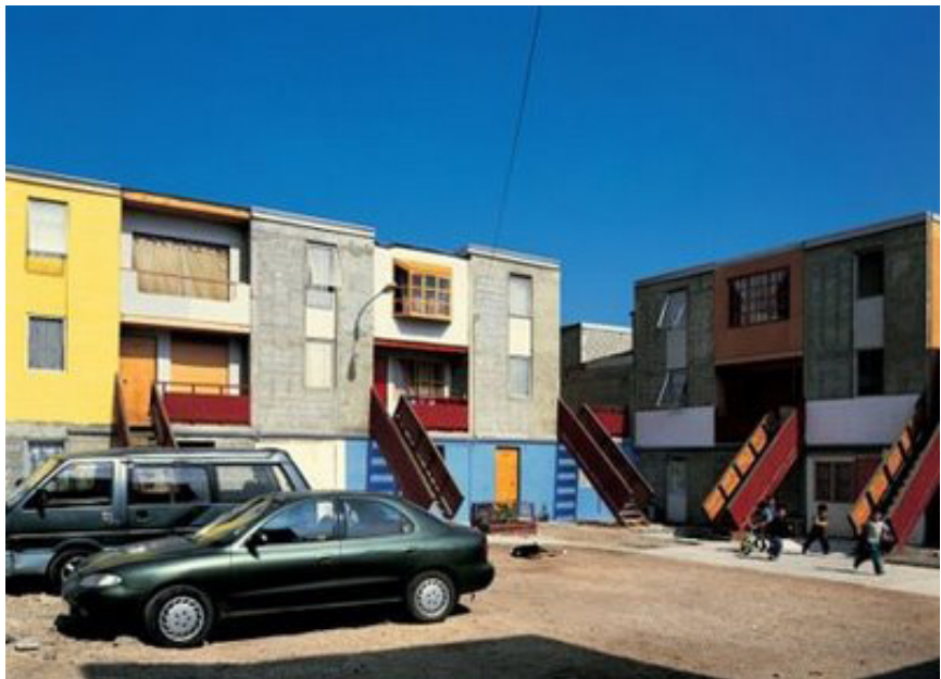
Fig. 2.28 RIGHT - Subsequent Ground Level View of affordable housing units with expansion between original units by residents.
