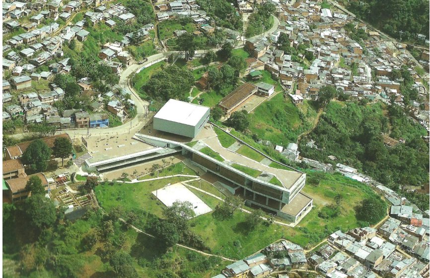
Fig. 2.21 RIGHT - Aerial View of a school and community center built as part of the program of social urbanism undertaken in Medellin, Colombia.
