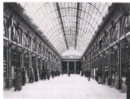
Figure 2.1-2 P. Fontaine's Galerie d'Orleans, Paris (1829) was an early example of the use of modular, mass-produced building components to augment more traditional architectural forms.
