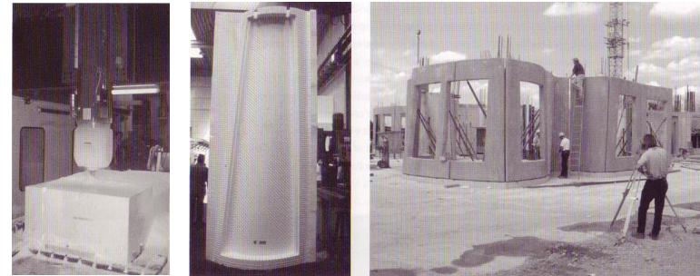
Figure 2.1-9 For Gehry Partners' Zollhof Towers, the complexly-shaped formwork needed for the prefabricated concrete panels was created using a CNC milling machine.
