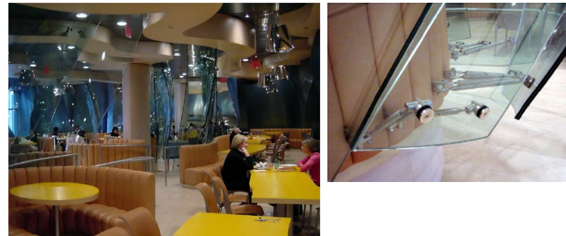
Figure 6-10 The doubly-curved glass panels Gehry Partners' Conde Nast Cafeteria required a custom glass-forming process to create. Numerous mock-ups and design revisions made by the fabricators C-Tek (glass) and TriPyramid (fasteners) were needed in order to find an elegant suspension solution that wouldn't cause the glass to fail. 44
