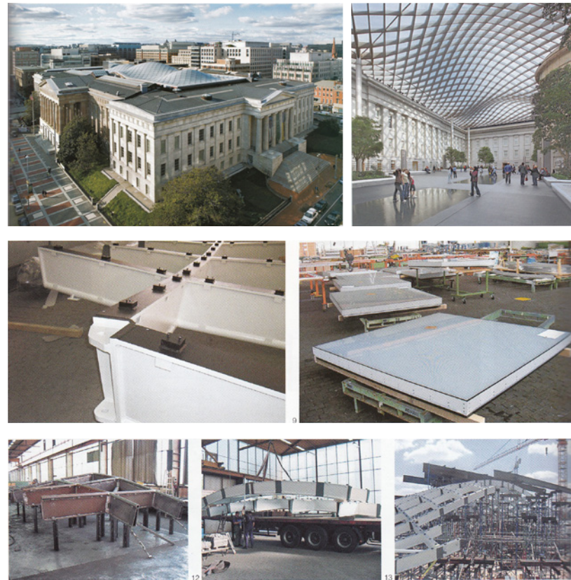
Figure 2.3-6 For the Smithsonian Courtyard Enclosure by Foster and Partners a simple control surface in the 3D model controlled thousands of unique parts. An optimized solution for the roof shape was determined based on feedback from the model with respect to factors such as sight lines, drainage, structural performance, and acoustics.
