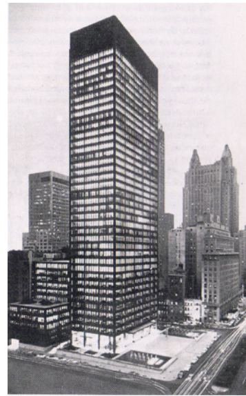
Figure 2.1-3 Mies van der Rohe's Seagram's Tower, New York (1958), was an iconic building that influenced the design of office towers for decades. Highly glazed uniform designs, while often cheap to produce, can present many challenges for energy efficiency and occupant comfort.
