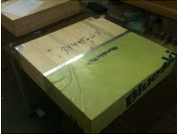
Step 3- Apply first half of self-adhering membrane Step 4- Finish membrane application
