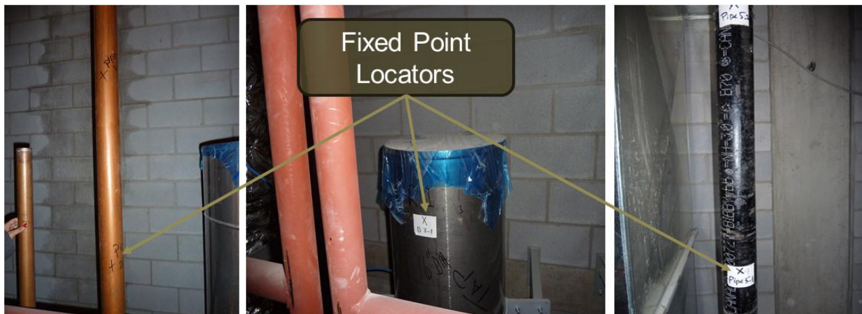
Figure 5-8: Point Locator Installations
