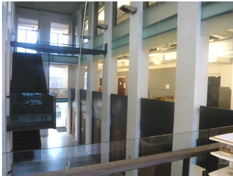
Figure 14-4: UWSA atrium columns
