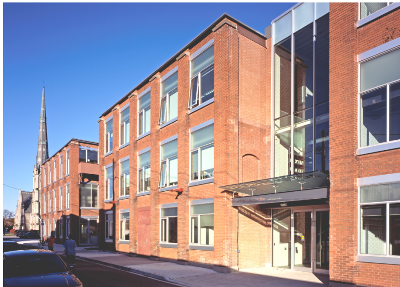
Figure 14-8: UWSA exterior, by Ben Rahn at A-Frame
