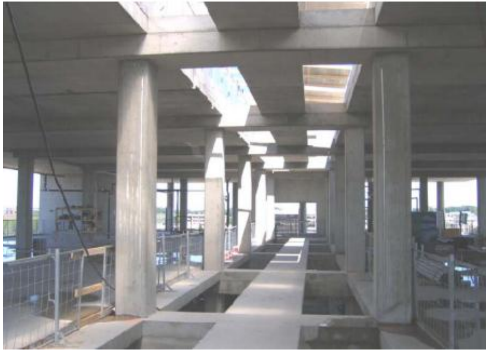
Figure 11: Service Corridor at the beginning of the study
