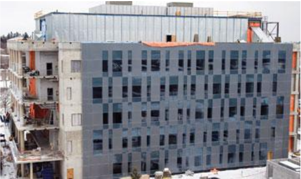
Figure 4: Engineering VI under construction, University of Waterloo
