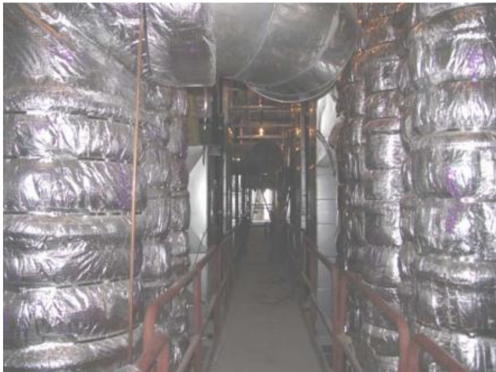
Figure 12: Service corridor at the end of the study
