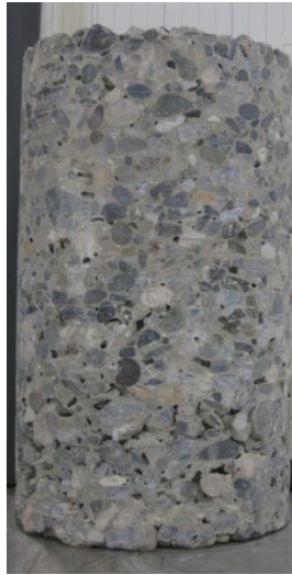
Figure 5-2: Core 2U1 from Site 3
