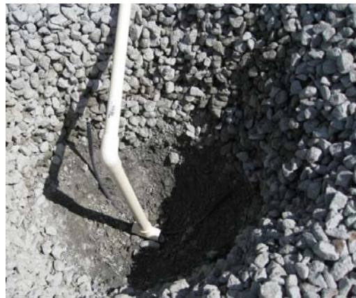
Figure 3-14: Temperature Probes Being Installed
