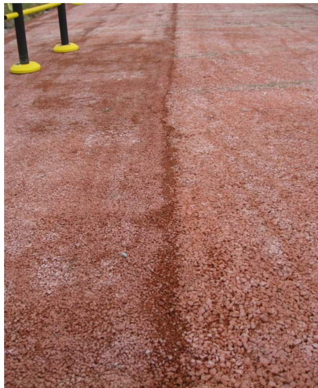
Figure 5-12: Construction Joint A/B at Site 4 November 2008 (1 Month)
