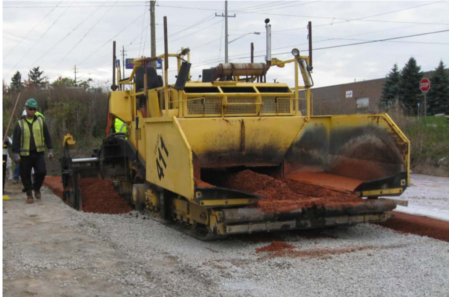
Figure 5-11: Construction of Site 4
