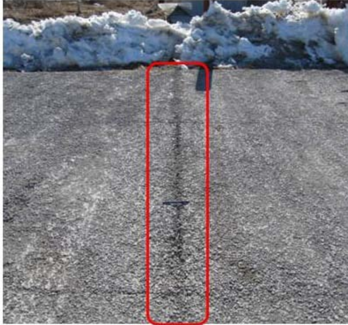
Figure 5-6: Formed Joint March 2010 (33 Months) Site 1
